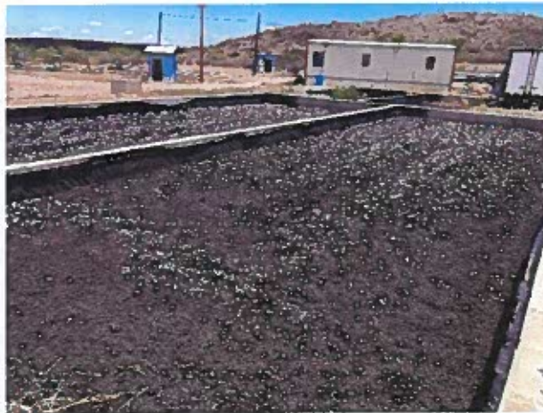
Figure 10 : Sludge Drying Beds
