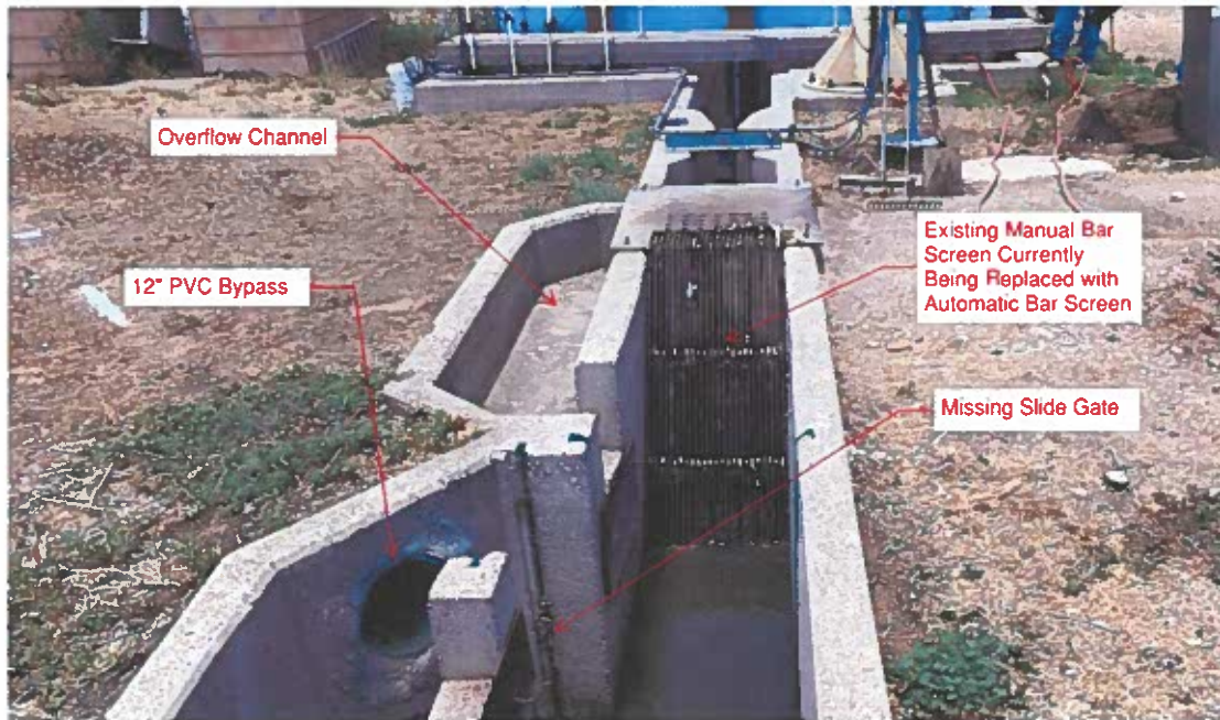
Figure 1 : Bar Screen and Emergency Bypass
