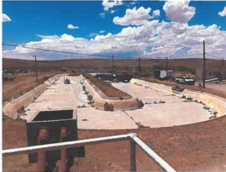
Figure 3 : Decommissioned Oxidation Ditch
