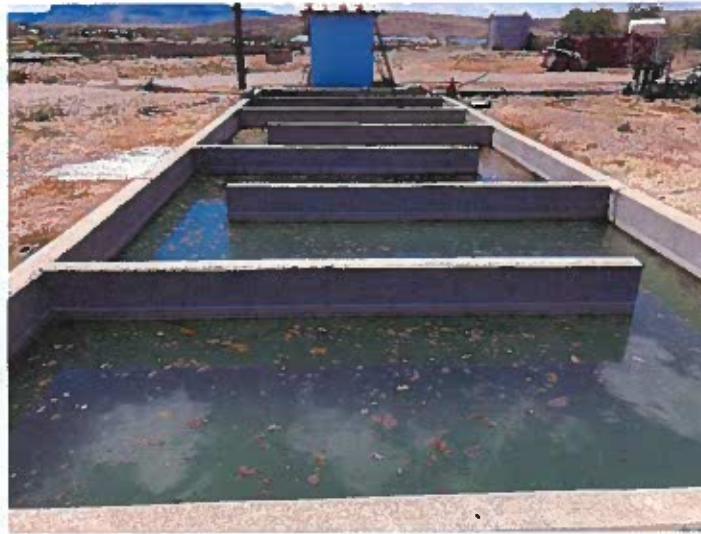
Figure 6 : Chlorine Contact Basin (1980)
