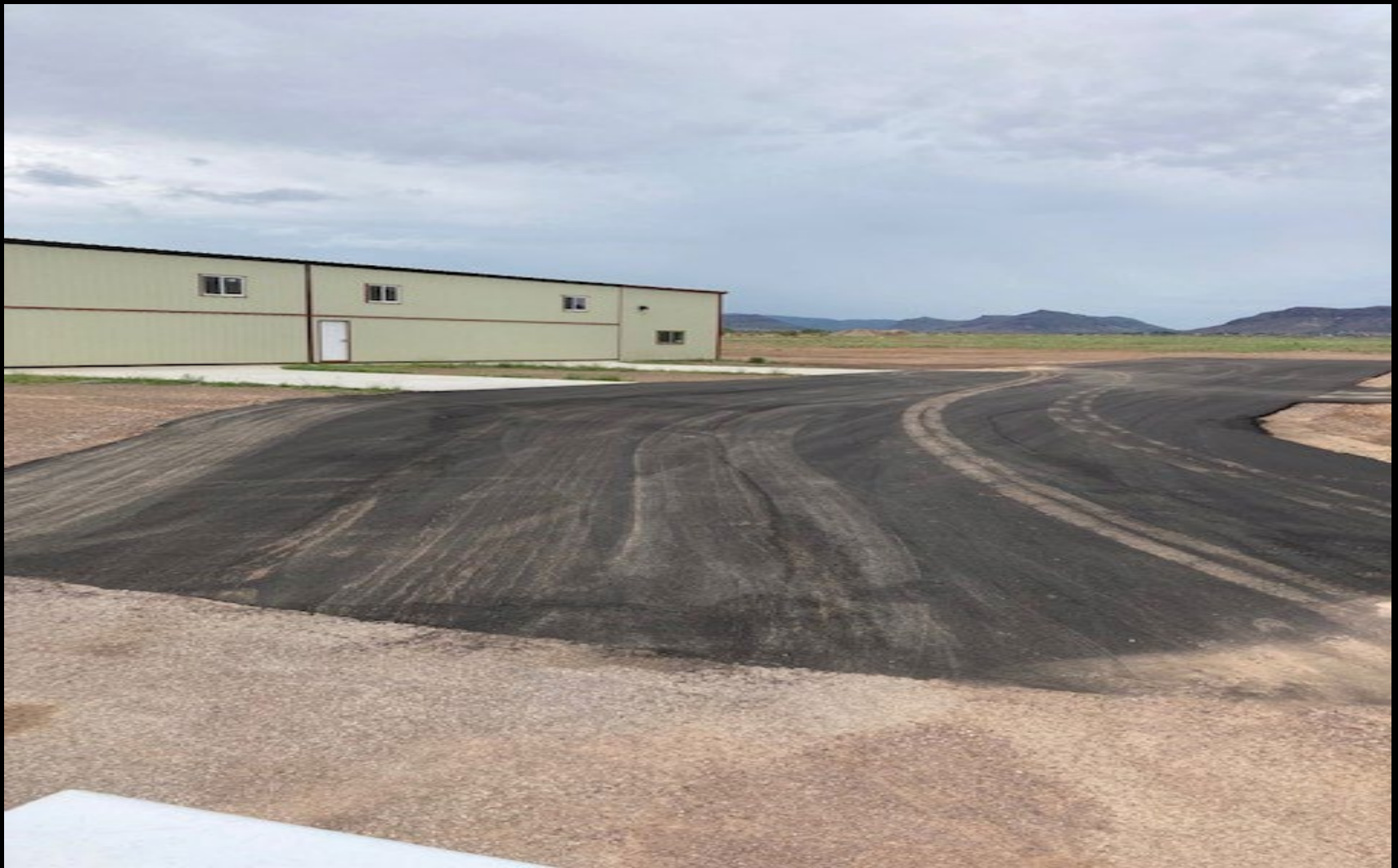
Recently Completed Paving Project: Taxiway north of Hangars #43 & #44
