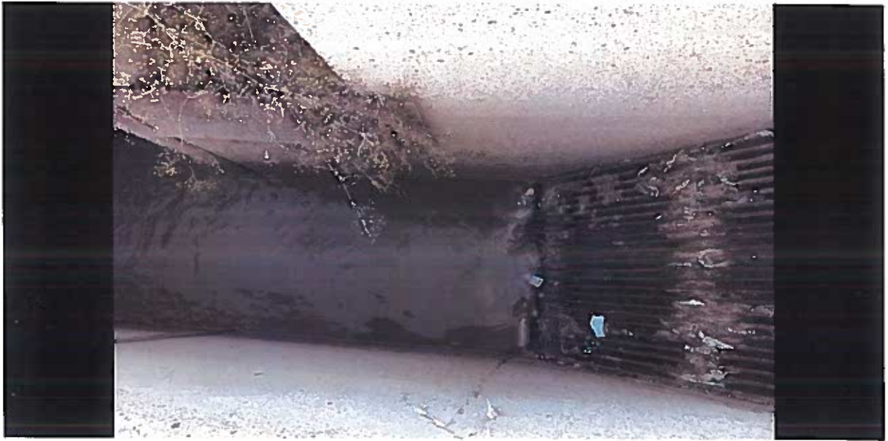
BAR SCREEN CURRENTLY IN USE AT THE WASTEWATER TREATMENT PLANT
