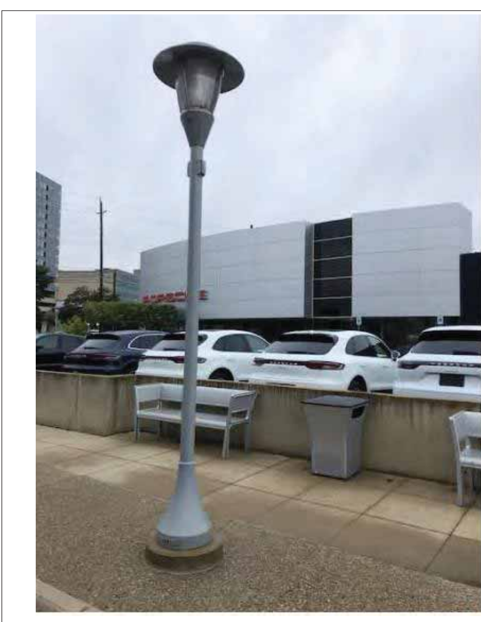
E EXISTING + NEW STREETLIGHTS (BL-X & BL-P) Lumen Street Light Model P790-42W To conform with Triangle District Standards
