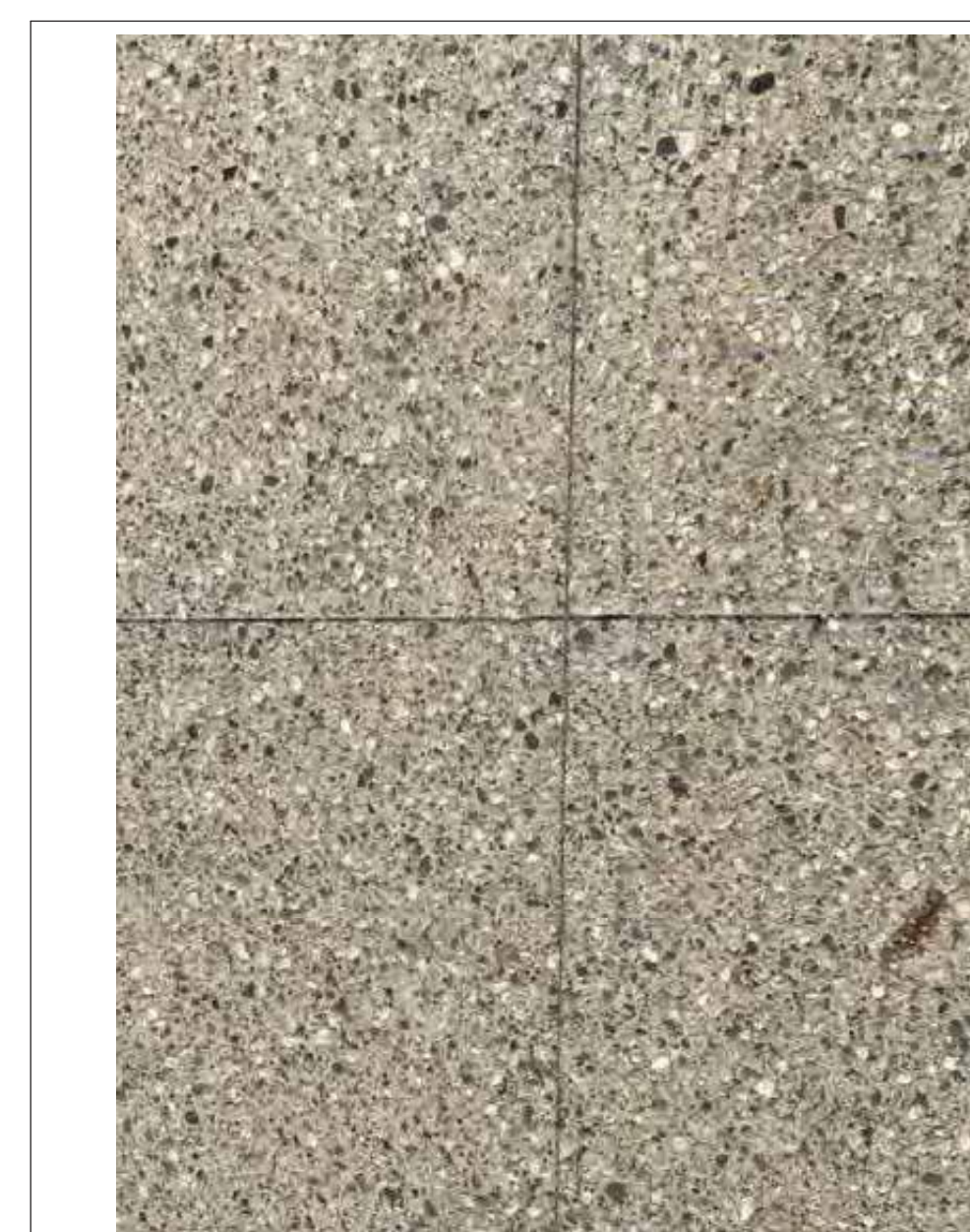
D EXPOSED AGGREGATE CONCRETE PAVING 30"x30" Scoring Pattern Typical
