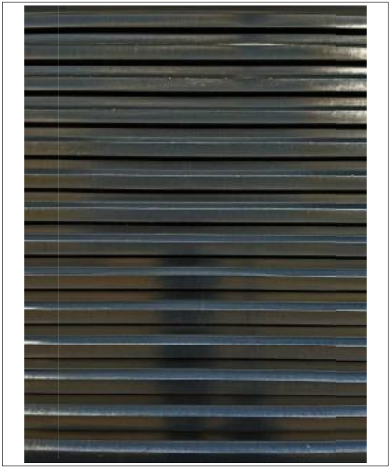
5 TYPICAL RIBBED METAL WALL PANELING (MP-1)
