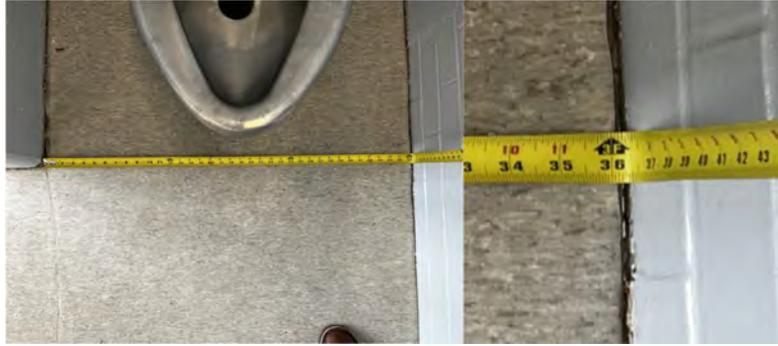
**IMAGE 4.2.33 - LOCK UP WATER CLOSET CLEARANCE**
