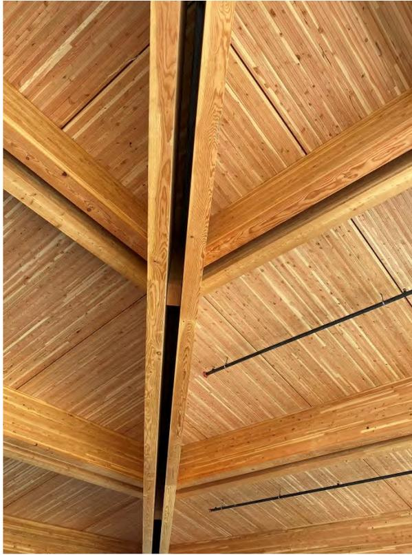
Figure 5.2: NLT and Glulam Girder System
