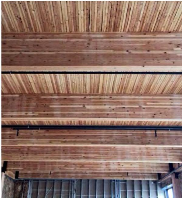
Figure 5.1: NLT and Glulam Girder System
