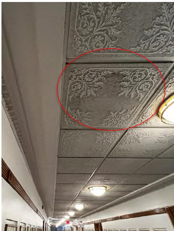
**FIGURE 2.3.06 – DUST BUILD-UP ON ACOUSTICAL CEILING TILES IN THE PRIMARY CORRIDORS.**
