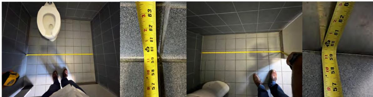
IMAGE 4.2.33 - 1ST FLOOR MENS WATER CLOSET CLEARANCE
