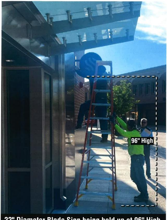
22" Diameter Blade Sign being held up at 96" High from the bottom of the Blade Sign to the ground.
