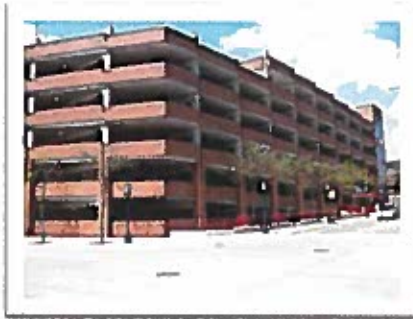
Peabody St. Parking Structure
