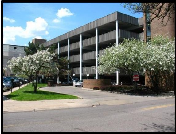
Park St. Parking Structure
