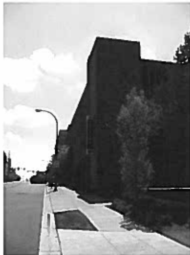
N. Old Woodward Ave. Parking Structure
