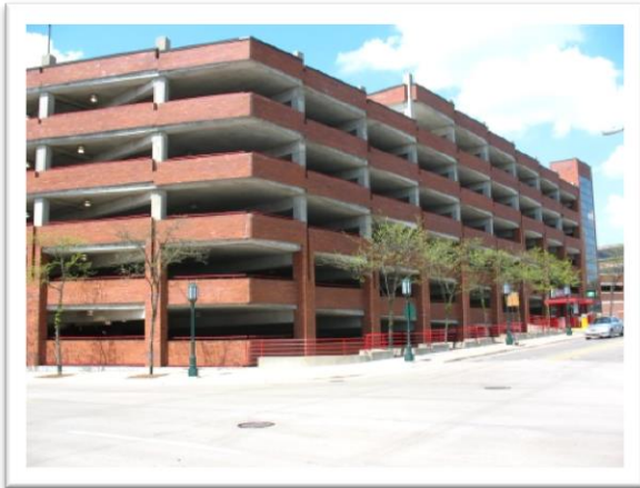
Peabody St. Parking Structure
