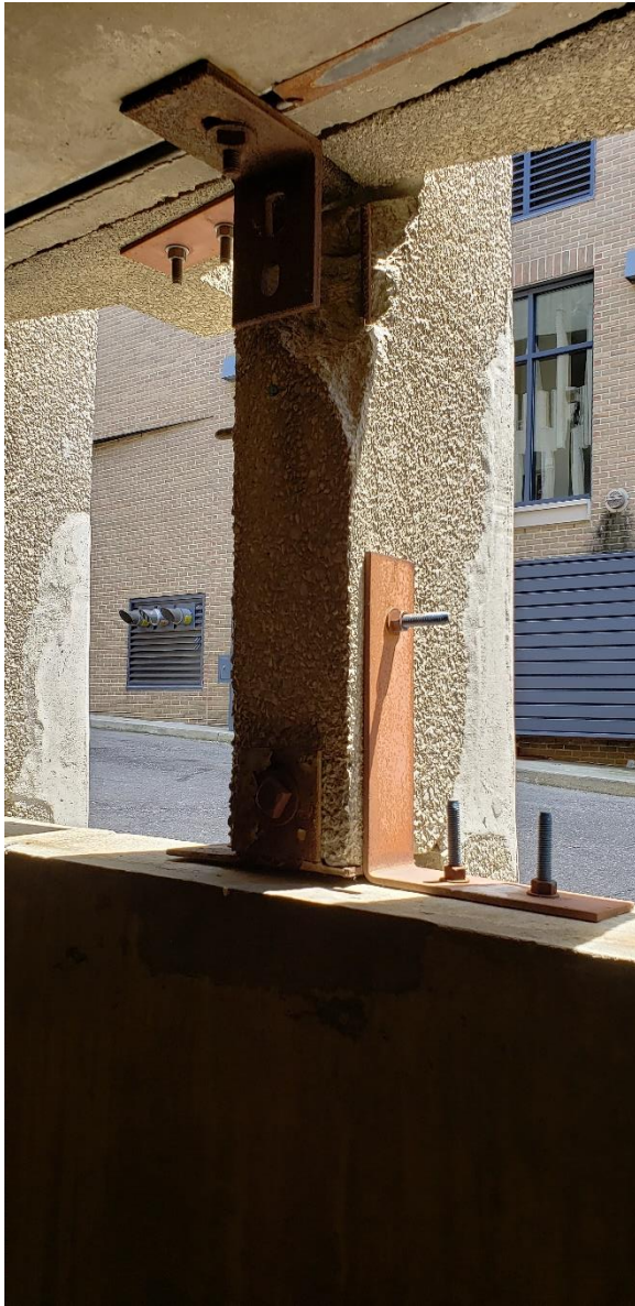
Figure 14. Single Level 1 precast concrete panel with post-installed connections..
