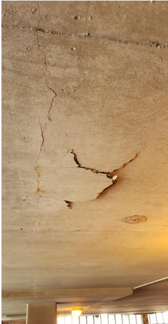
Figure 1. Spalled, loose concrete on the slab underside.
