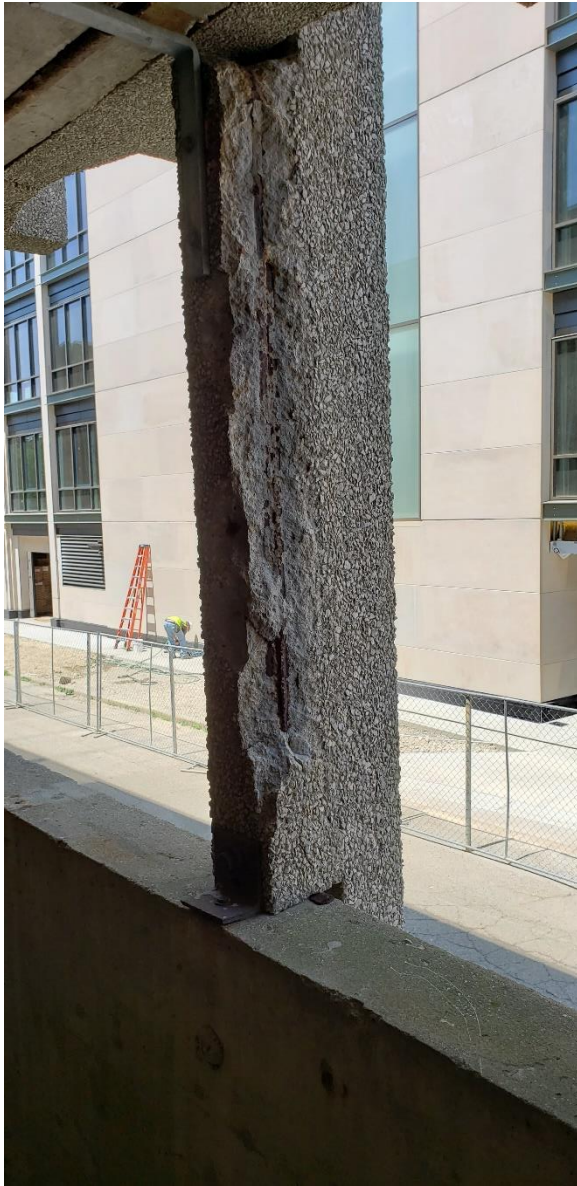
Figure 18. Concrete spall exposing corroded reinforcing bars at the interior of a precast panel.
