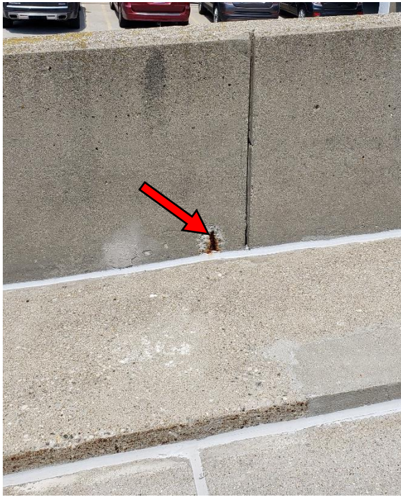
Figure 11. Localized spall at the Level 5 ramp wall.
