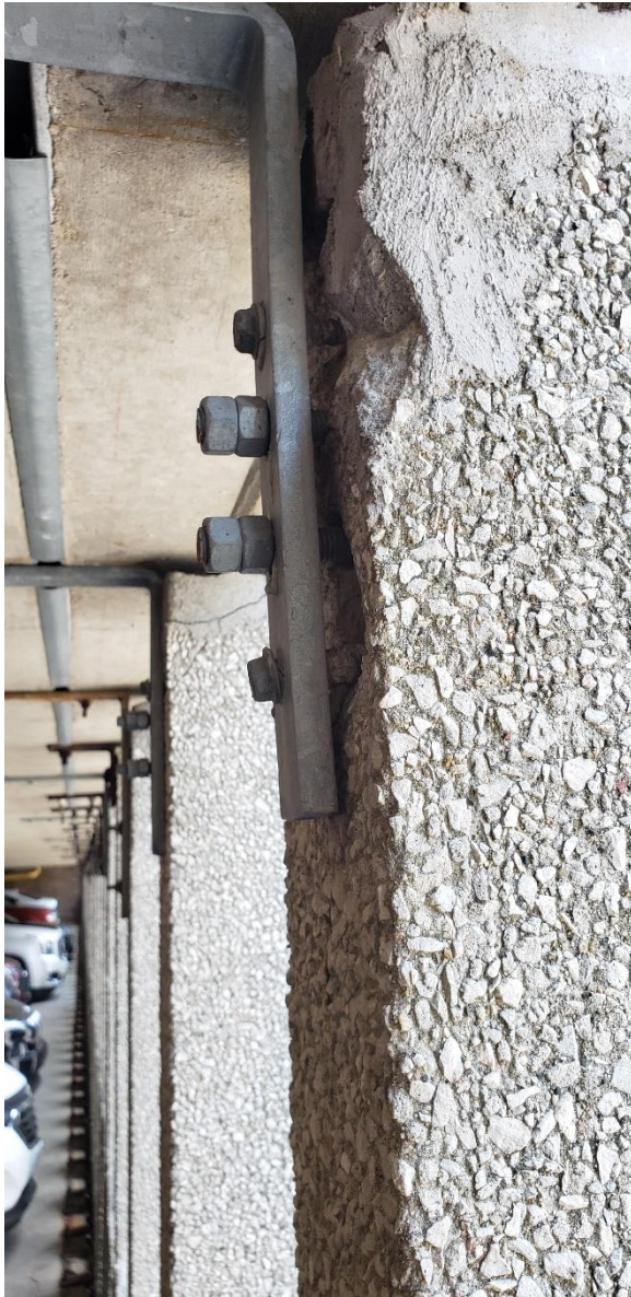
Figure 15. Post-installed panel connection with missing concrete at the connection bolts.
