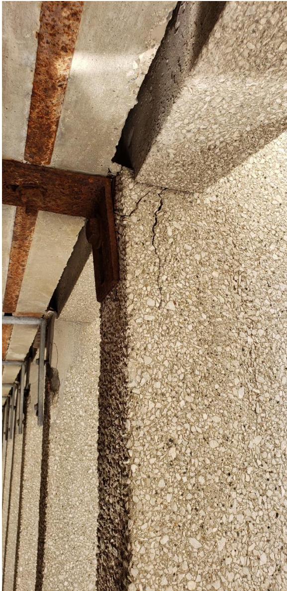
Figure 19. Incipient spall at the top connection of a precast panel.
