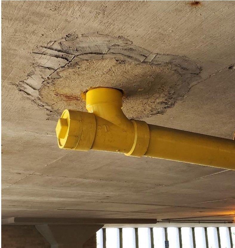
Figure 7. Unsound, failed previous repair at piping.
