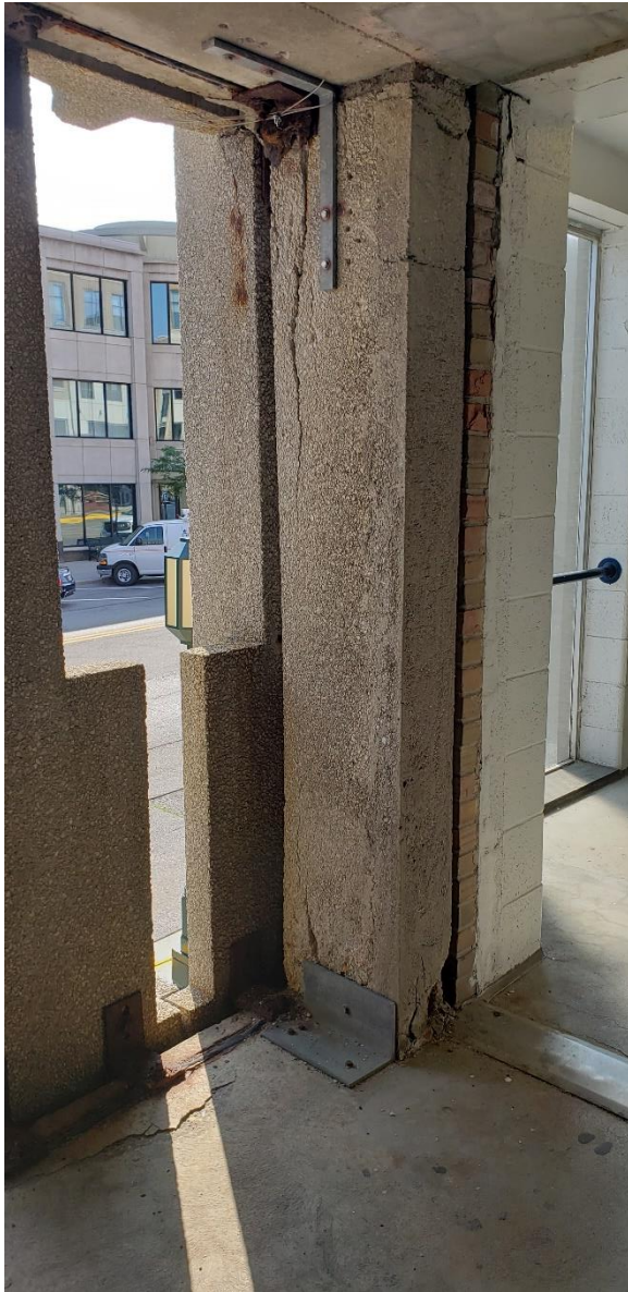
Figure 8. Exterior column exhibiting cracks, spalls, and unsound concrete.
