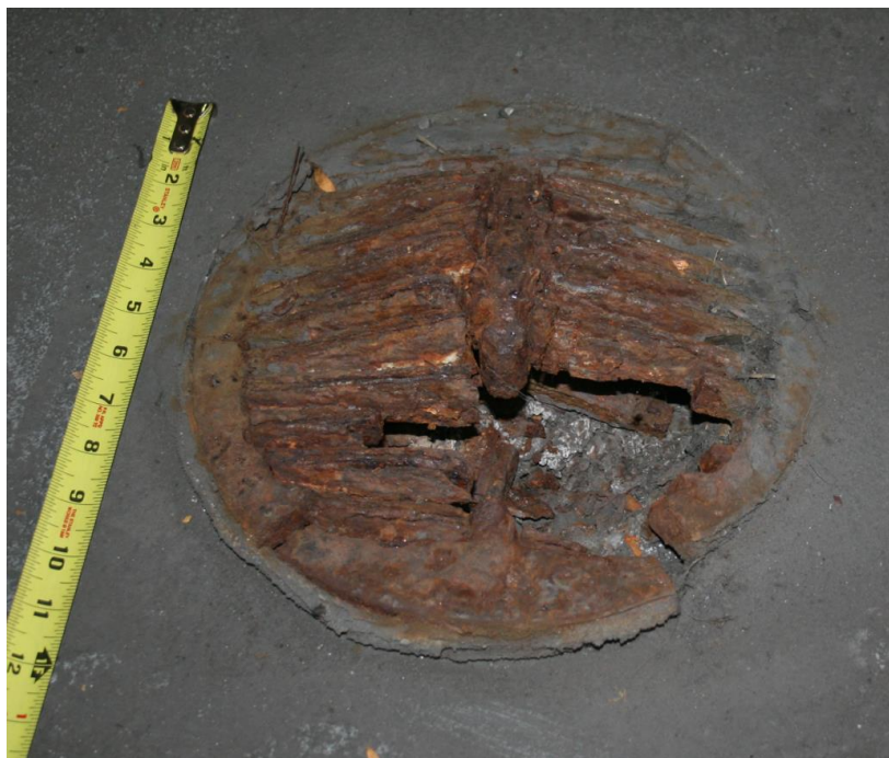
Figure 9. Severely corroded drain head
