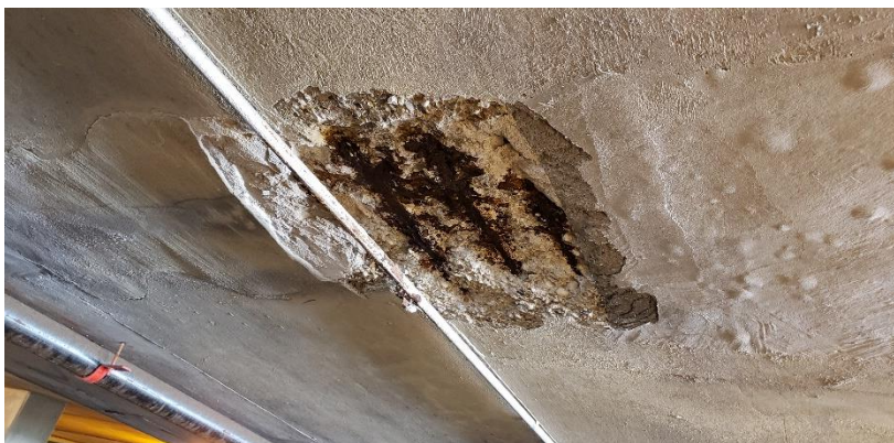
Figure 3. Spall near previous repair with corroded reinforcing bars.
