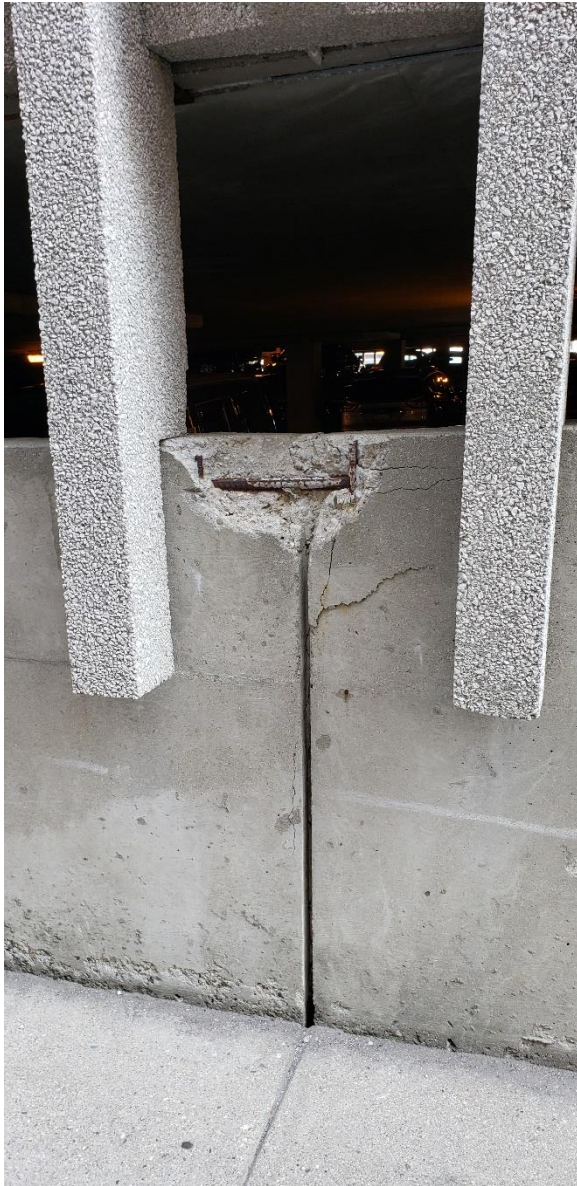
Figure 12. Localized spall at the Level 1 wall.
