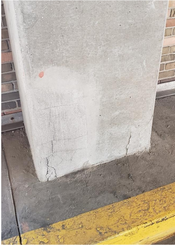
Figure 9. Interior column with unsound concrete at the bottom corners (unsound concrete on the bottom left is at a previous repair).
