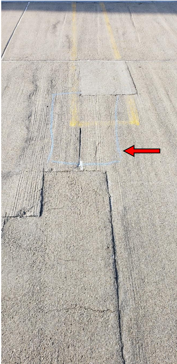
Figure 4. Unsound concrete outlined in blue (indicated by the arrow) adjacent to previous topside slab repairs.
