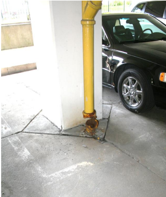
Figure 10. Corroded steel drain line at clean out
