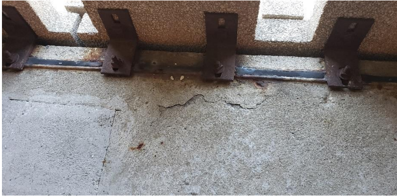
Figure 22. Typical surface corrosion at the precast panel steel angles.
