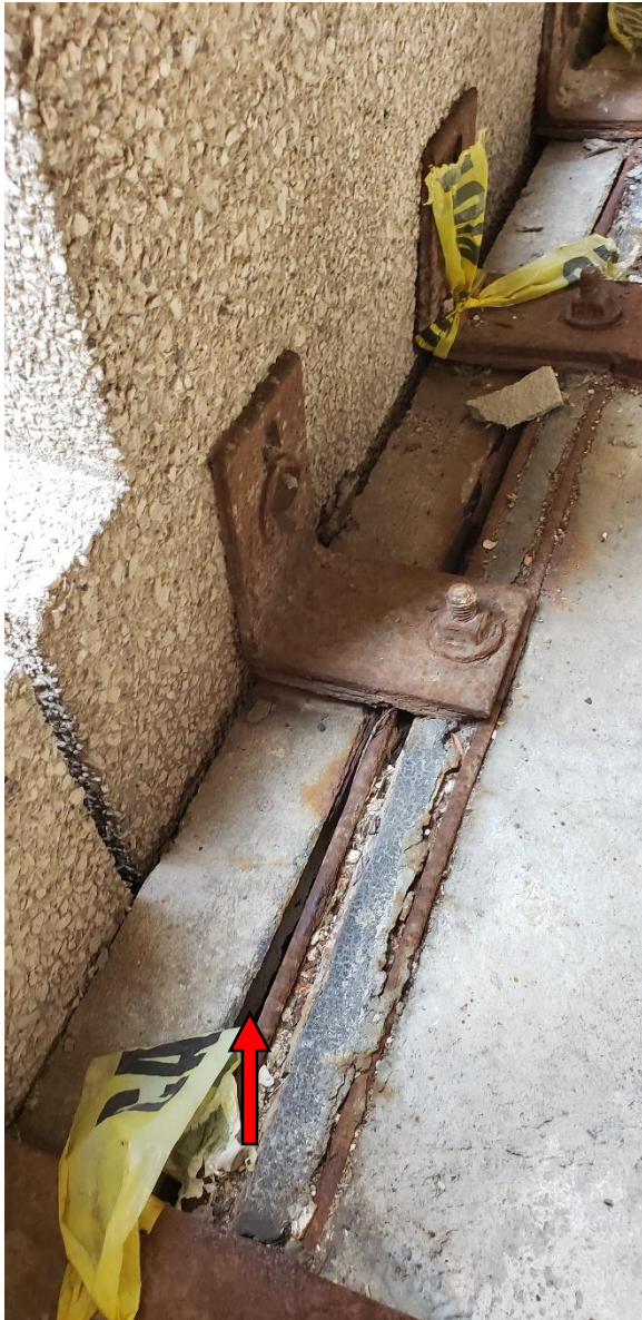
Figure 21. Concrete deterioration and separation (indicated by the arrow) at the bottom connections of a precast panel.
