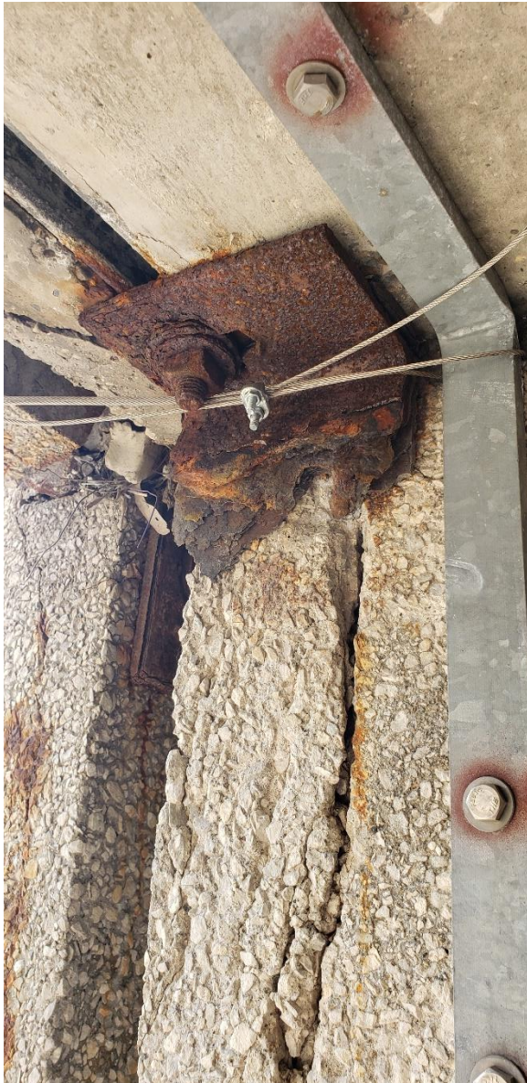
Figure 10. Pack rust at the top angle attachment of an exterior column.
