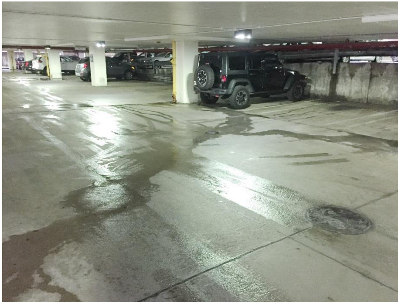
Figure 11. Water on the ground floor entering the floor drains.
