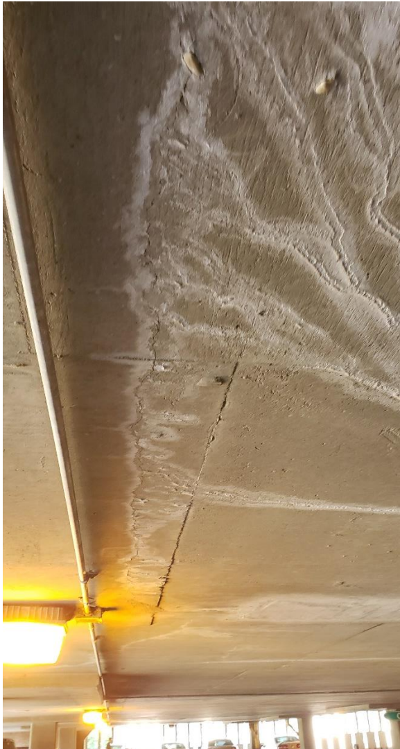
Figure 5. Cracks with leaching efflorescence.
