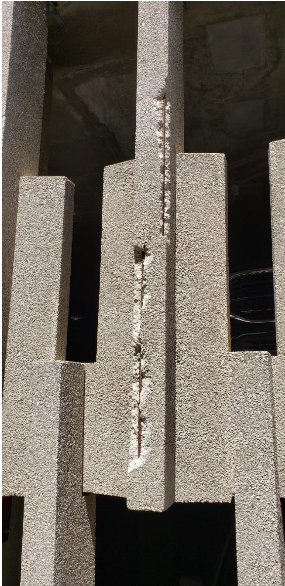
Figure 17. Concrete spalls exposing corroded reinforcing bars at the exterior of a precast panel.
