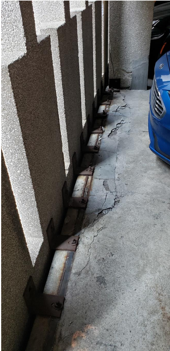
Figure 24. Concrete curb spalls near the connections at the bottom of precast panels.
