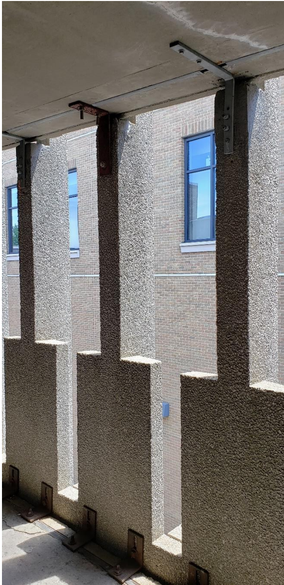
Figure 13. Typical single precast panel. Note the three vertical sections connected at the bottom, creating a single panel.
