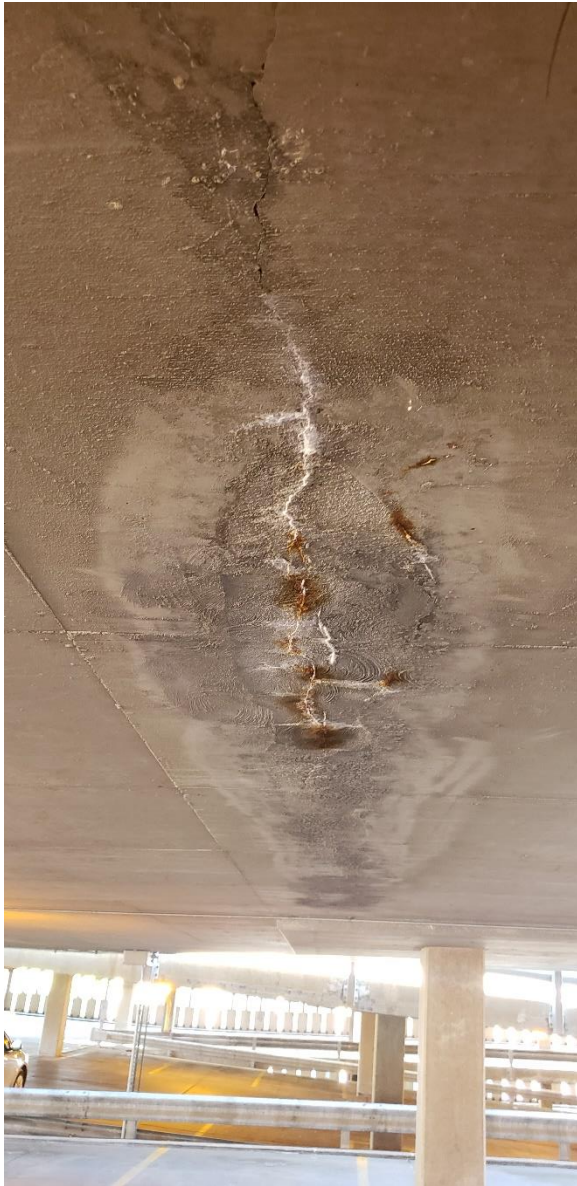
Figure 6. Cracked previous repair with efflorescence and corrosion staining.
