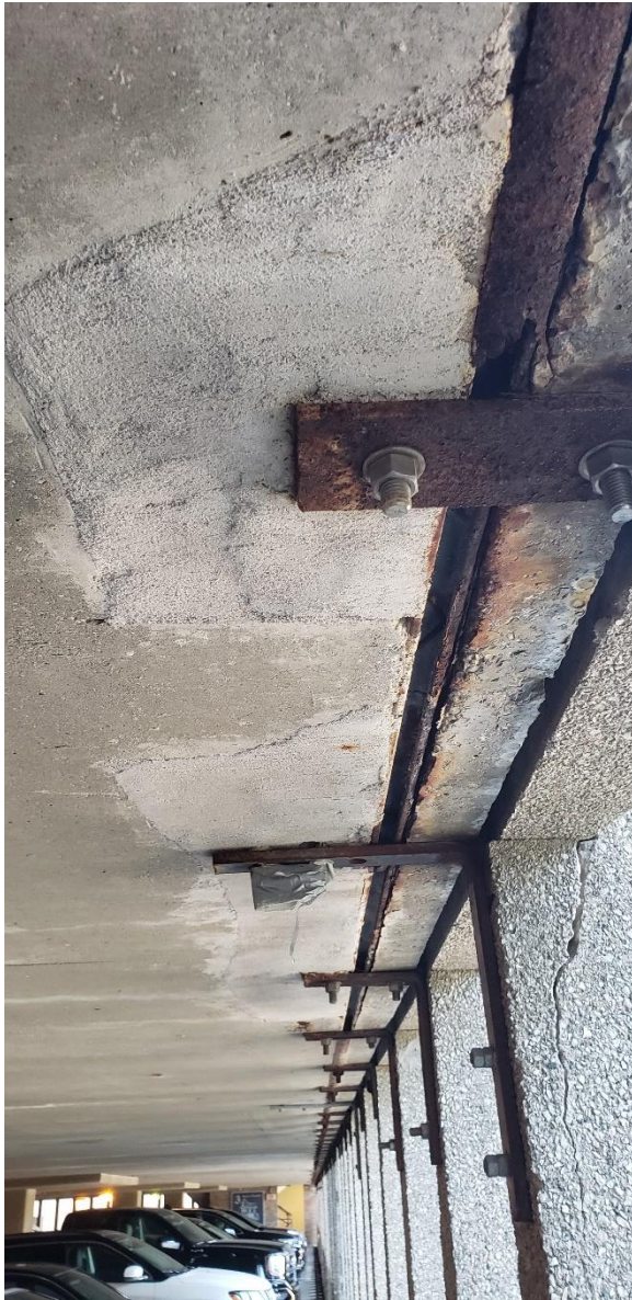
Figure 23. Corroded embedded steel slot.
