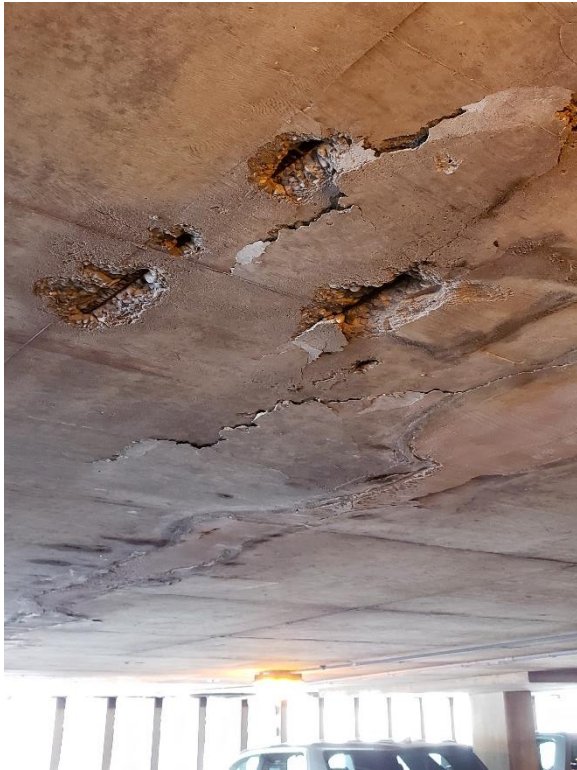
Figure 2. Spalled, loose concrete with visible corroded reinforcing bars on the slab underside.
