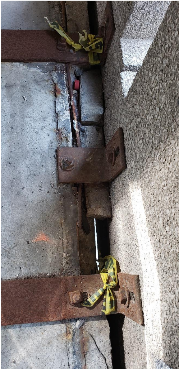
Figure 25. Concrete spalls and missing concrete at the concrete curb edge at the bottom precast panel connections.
