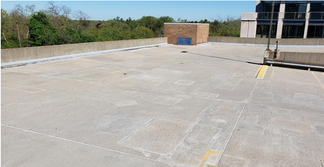
Figure 4. Partial overview of Level 5 with multiple locations of unsound concrete outlined in chalk.
