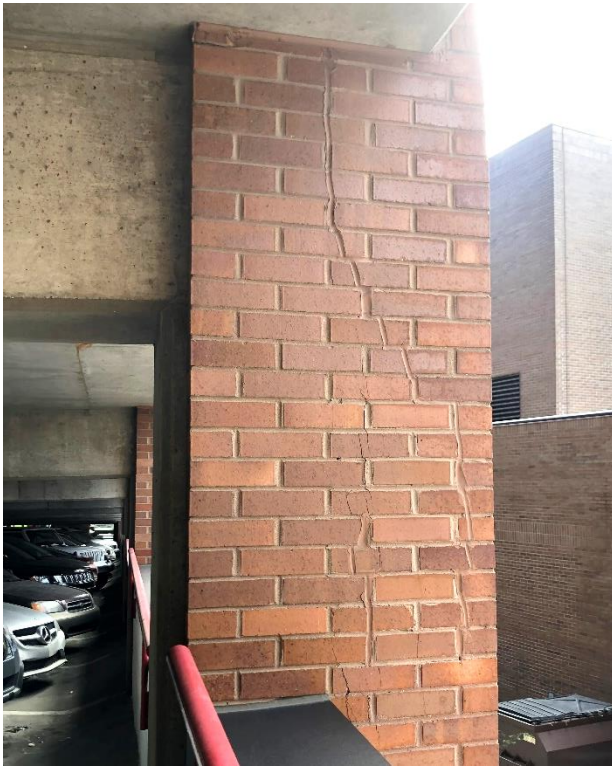
Figure 31. Vertical cracking in brick veneer at column cap.
