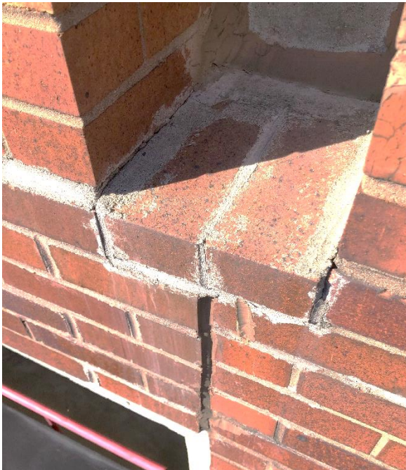
Figure 41. Debonded mortar at vertical discontinuity within brick cladding.
