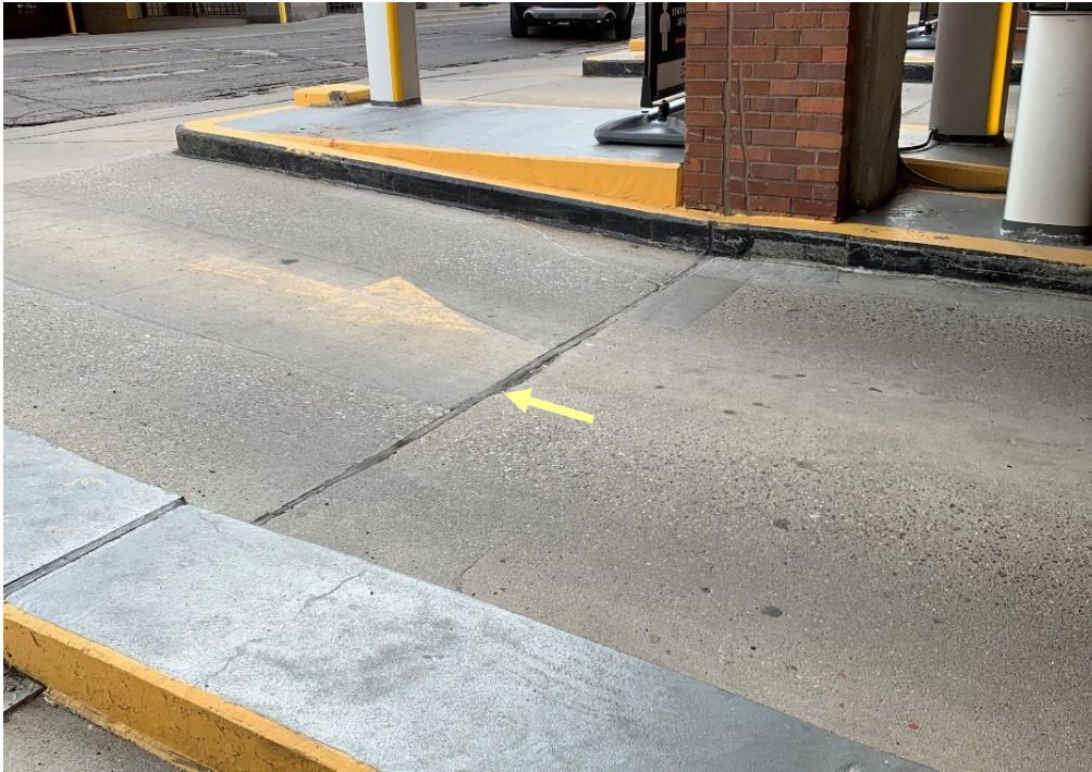
Figure 19. Joint sealant at vehicle entry between vaulted sidewalk region (plenum) and garage interior.
