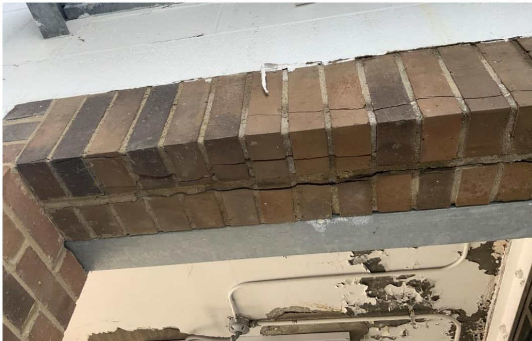
Figure 81. Cracked brick masonry header
