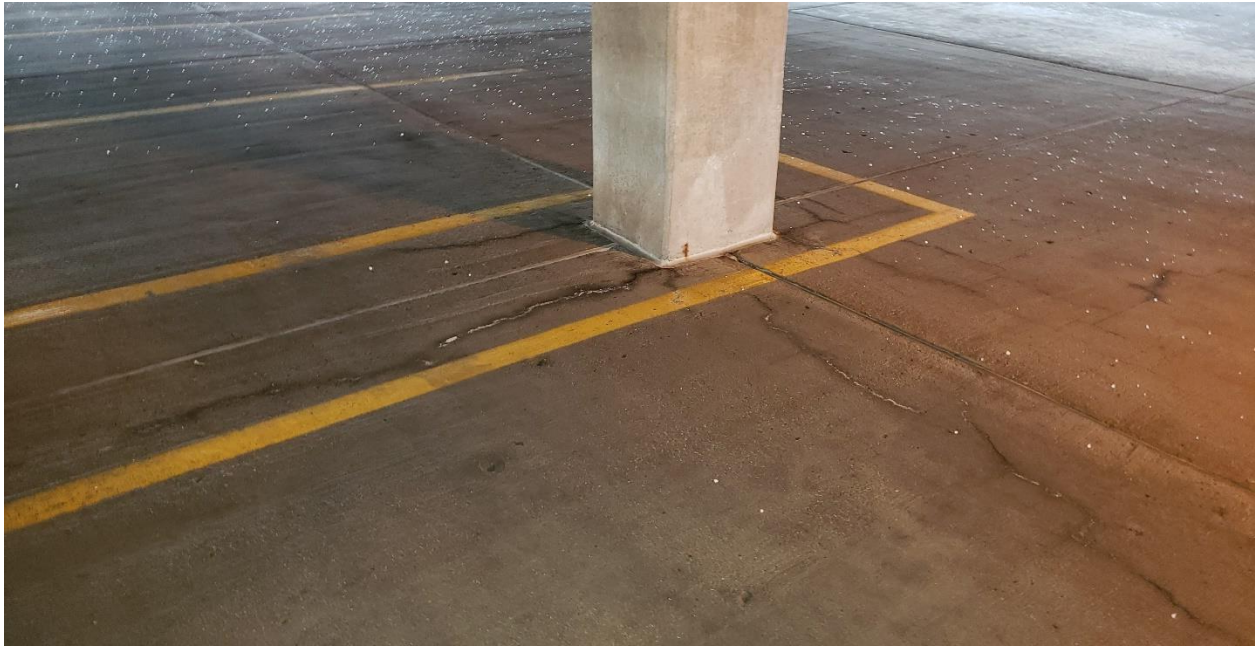
Figure 7. Radial cracks extending from a column.
