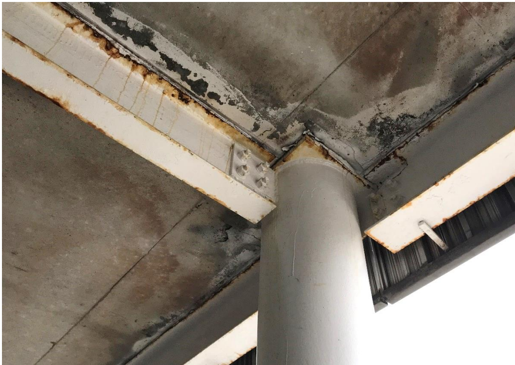
Figure 45. Corroded top of column and beam
