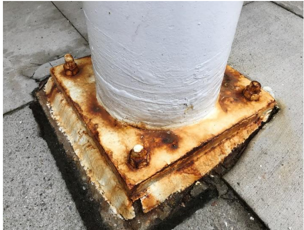
Figure 42. Corroded base plate at exterior pipe column
