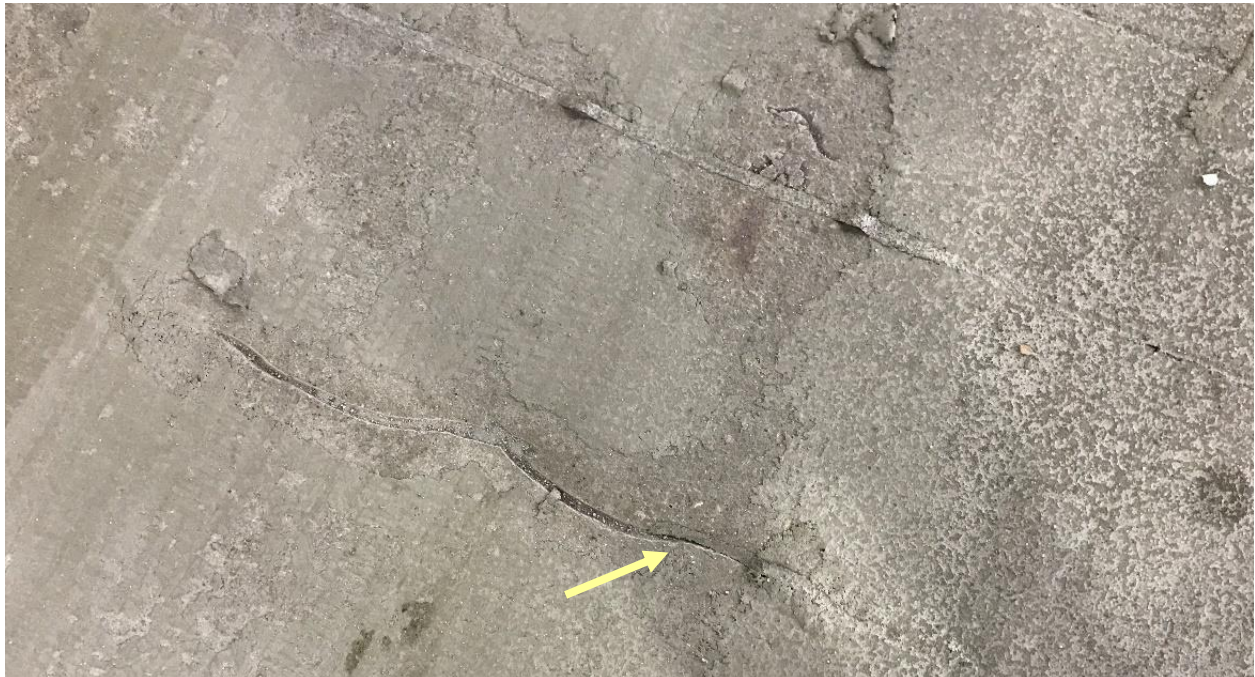
Figure 35. Failed sealant at crack
