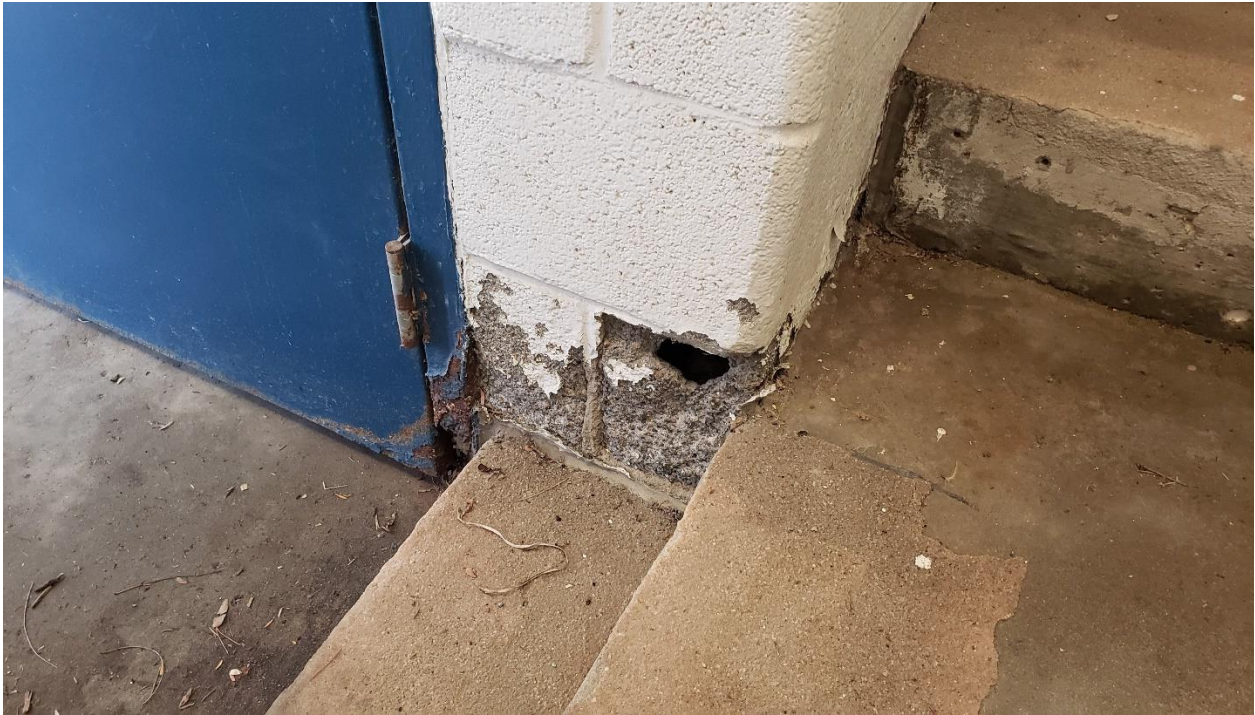
Figure 27. Deteriorated CMU blocks at the base of the stair.
