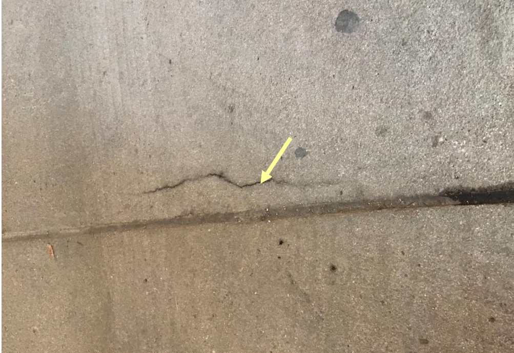
Figure 1. Area of unsound concrete along construction joint.
