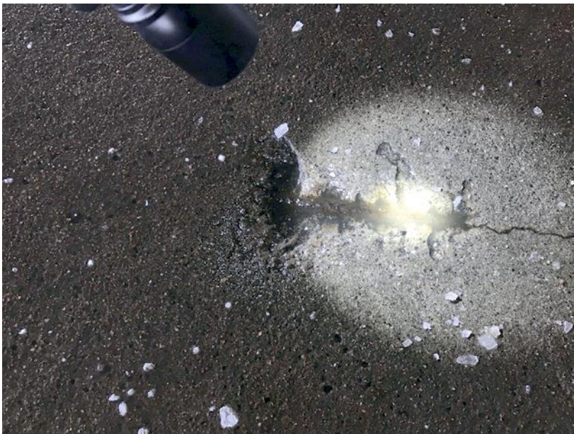
Figure 2. Spall exposing corroded mild reinforcing steel.
