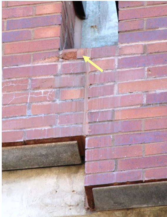
Figure 40. Brick distress at vertical discontinuity.
