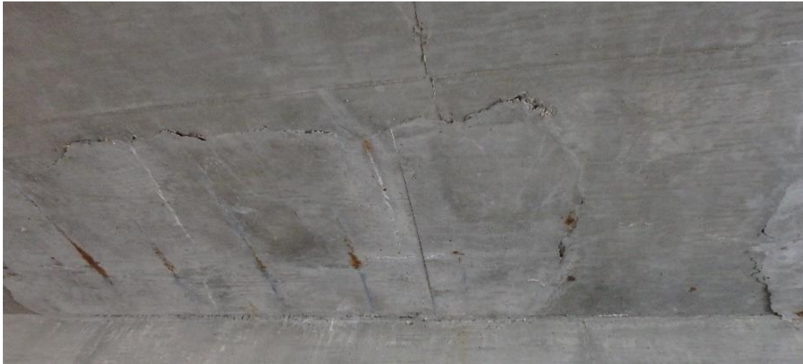
Figure 5. Isolated cracks, efflorescence, and corrosion staining at PT tendon anchorage repairs.
