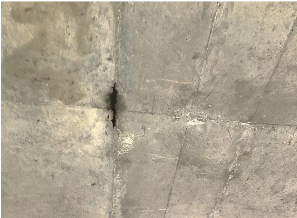
Figure 11 . Grease stains at underside of elevated slab at construction joint.
