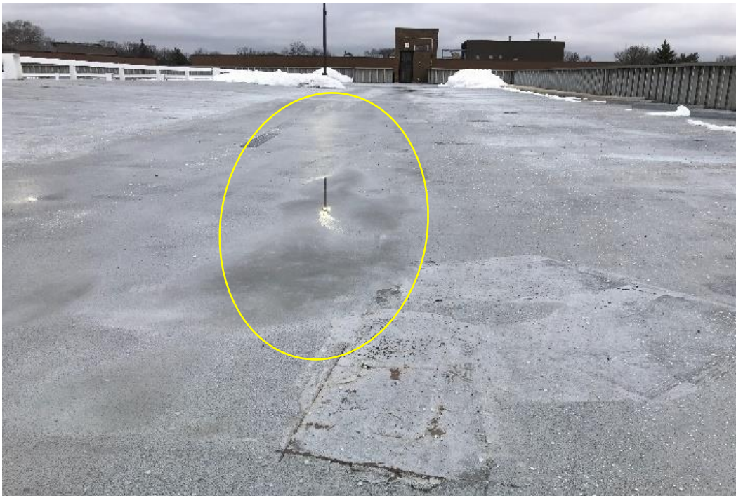
Figure 71. Standing water at unsloped bay of roof level
