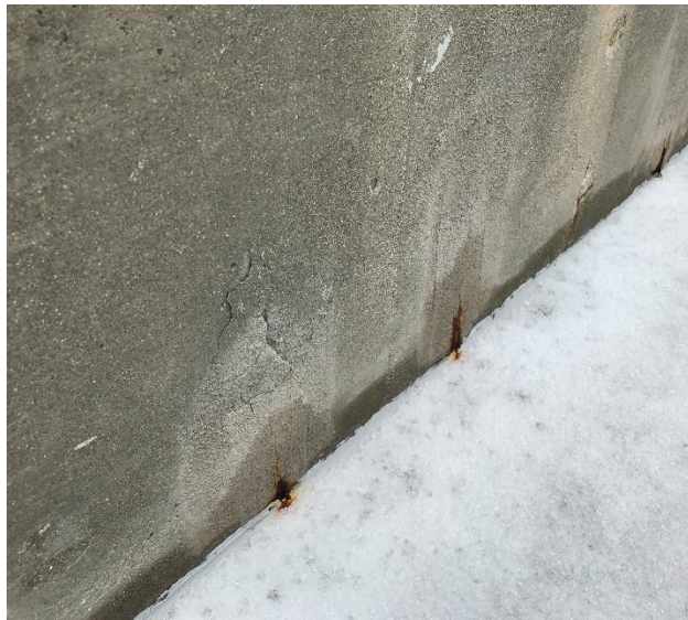
Figure 16. Corrosion stains and exposed corroded reinforcing bars at areas of low concrete cover.
