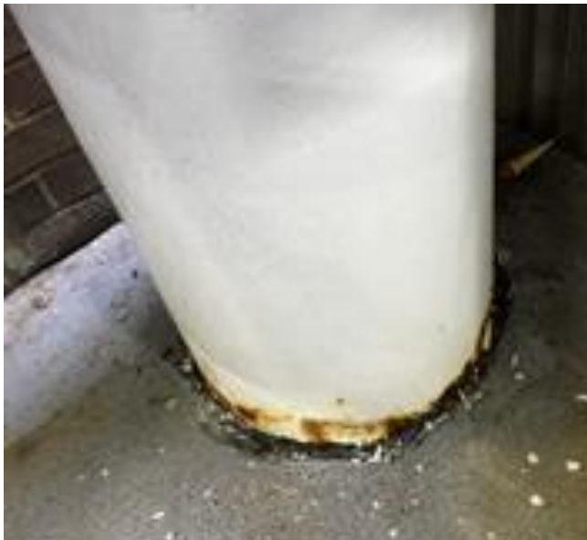
Figure 40. Corrosion at base of exterior pipe column
