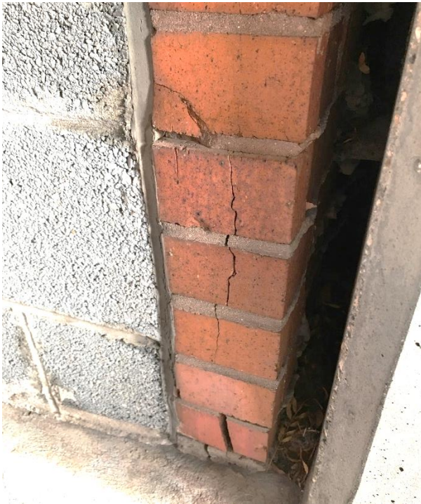
Figure 37. Vertical crack in veneer.
