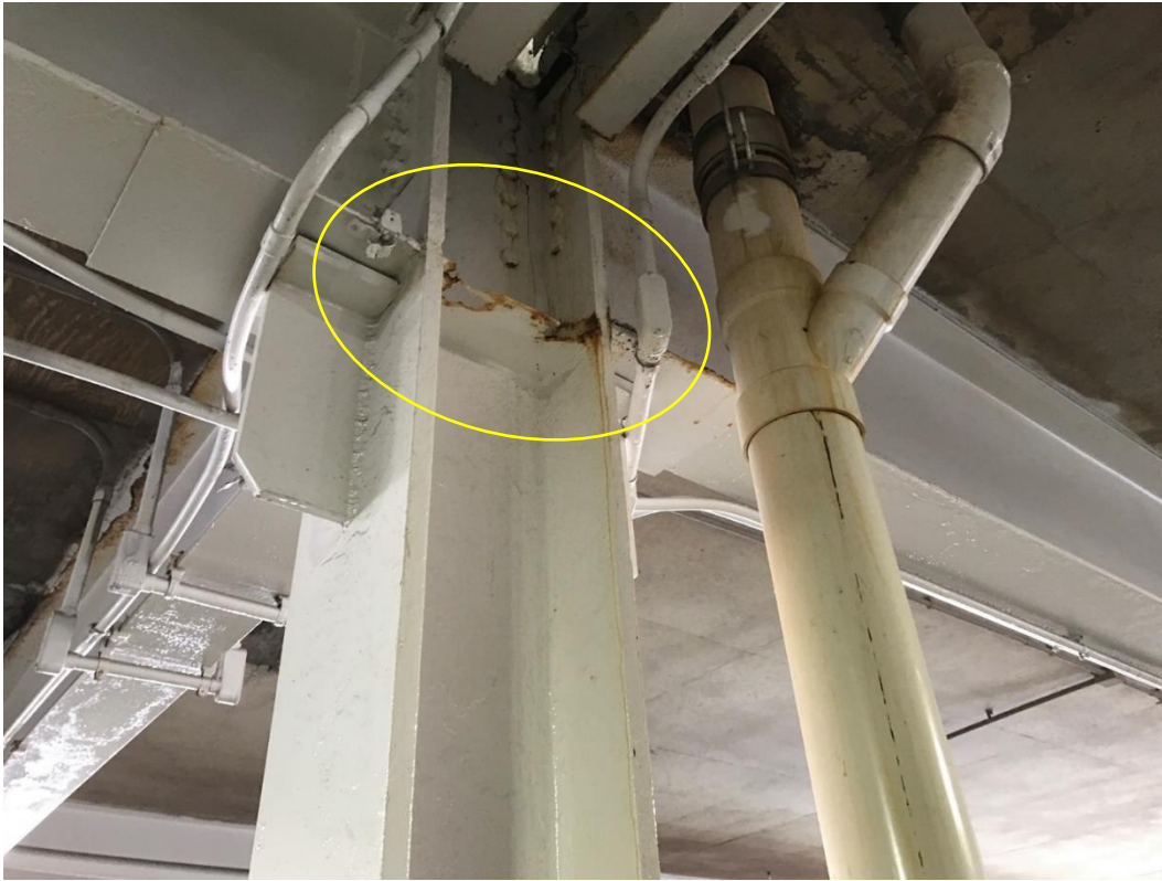
Figure 46. Section loss at column stiffener plate
