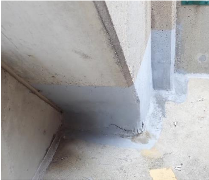
Figure 29. Delaminated coating at inclined column base, Tier 3.
