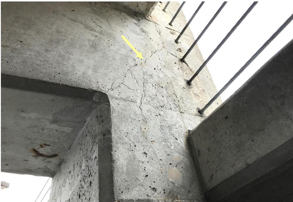
Figure 24. Cracking at the beam-column intersection.
