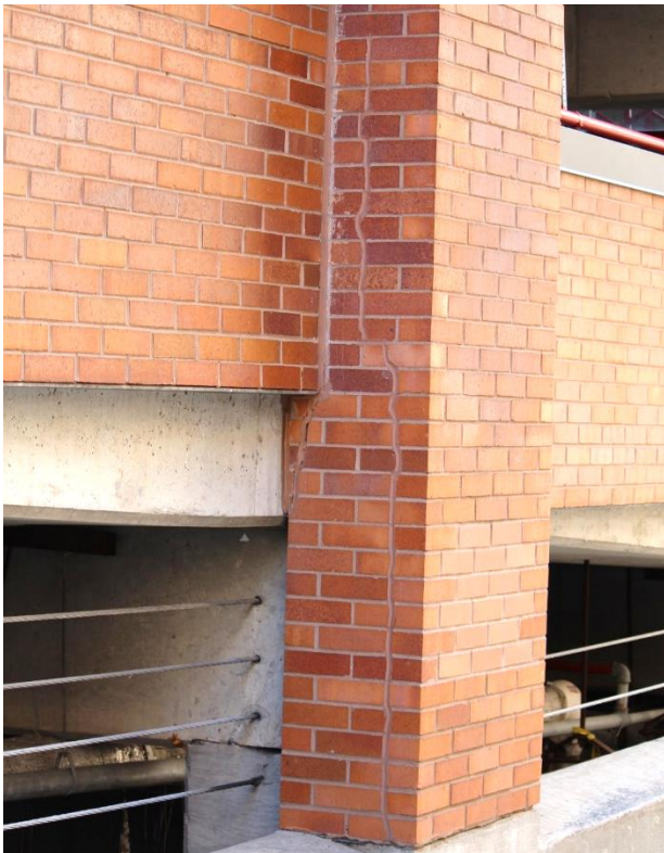
Figure 33. Vertical cracking in brick veneer at column cap.
