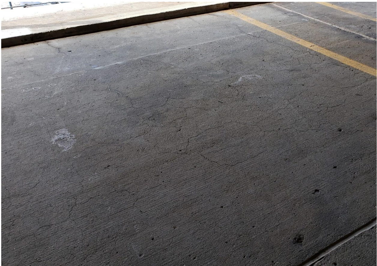
Figure 8. Example of crazing cracks on the top surface of a concrete slab.
