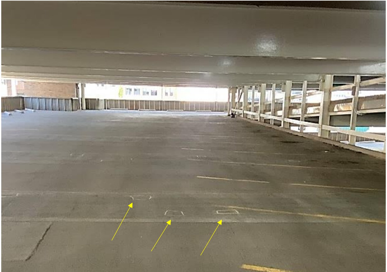
Figure 27. Delaminations near the beamlines marked in chalk
