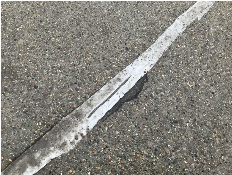
Figure 22. Joint seal adhesive failure in a topping slab joint.
