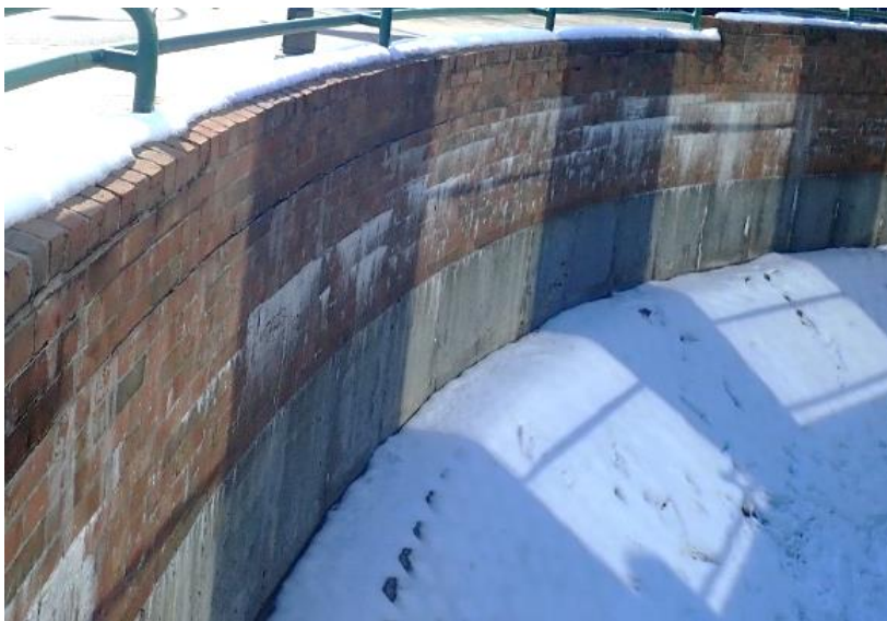
Figure 36. Efflorescence staining and eroded mortar joints at site wall.
