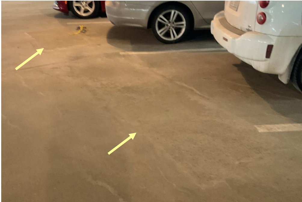
Figure 10. Previous PT tendon repair at Level 1.
