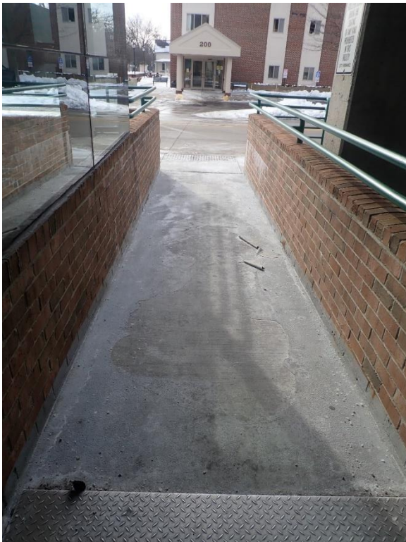
Figure 28. Delaminated coating at pedestrian bridge.
