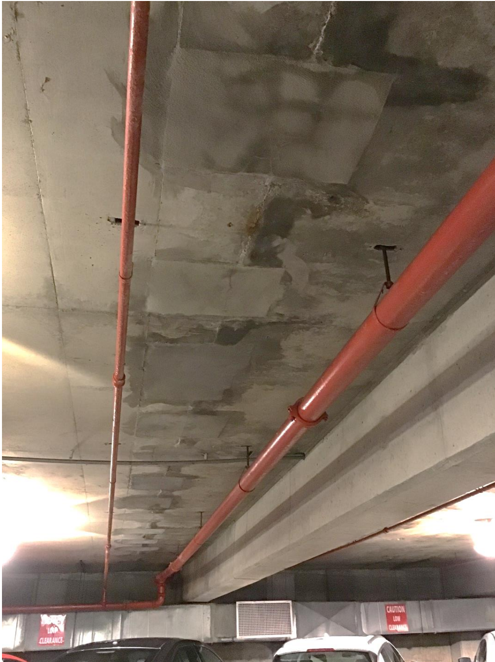
Figure 7. Previous partial-depth concrete repairs at Level 1 construction joint, aligned with mild reinforcing bars near bottom of slab surface.
