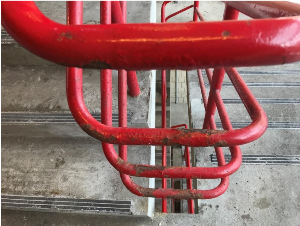
Figure 50. Chipped paint and corrosion at stairwell handrail.
