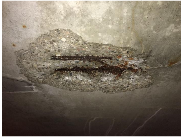
Figure 2. Spalled concrete with exposed corroded reinforcing bars.
