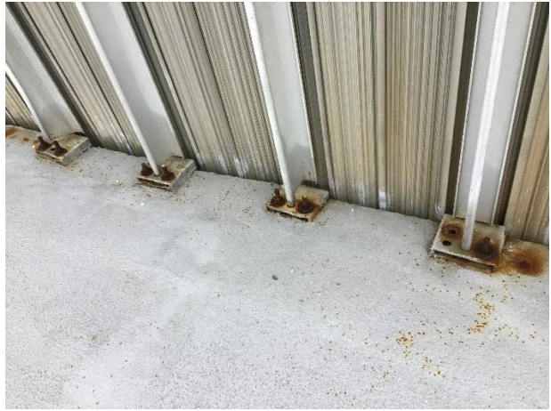
Figure 78. Corroded and missing anchors at facade panels
