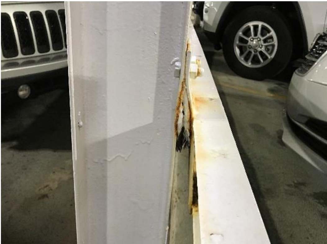
Figure 61. Corrosion byproduct buildup at channel to post connection
