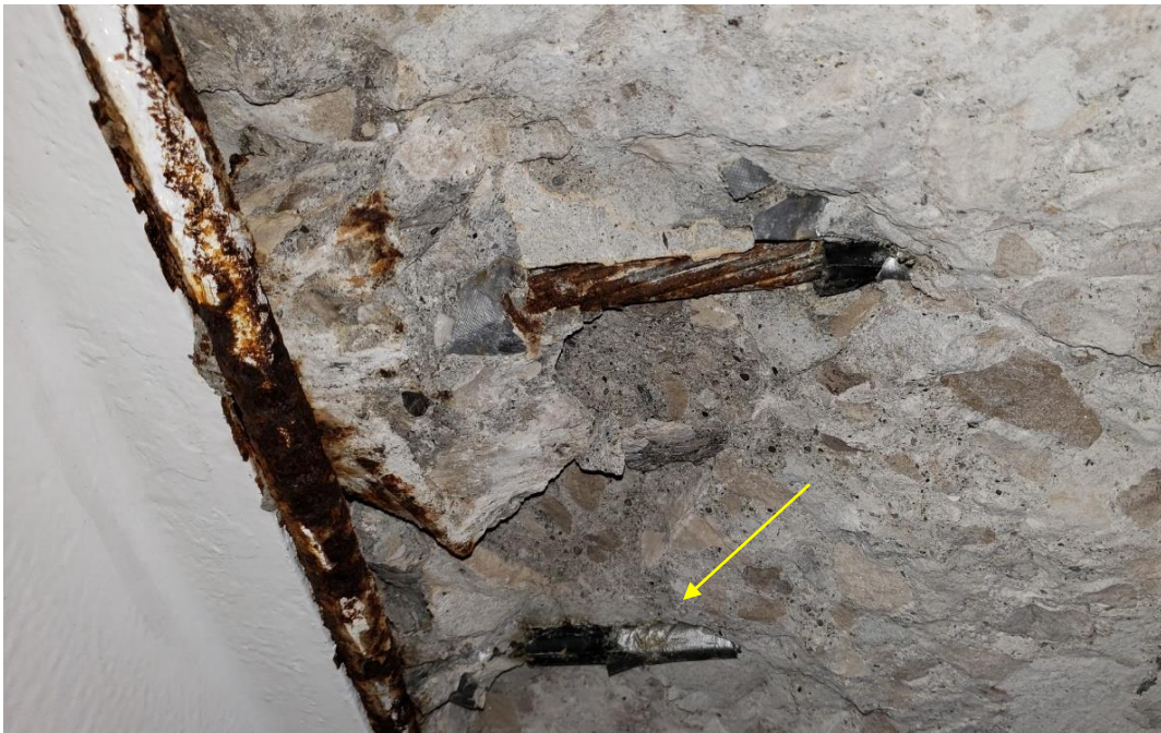
Figure 16. Exposed Tendon Location 5. Arrow indicates location of duct tape sheathing repair.
