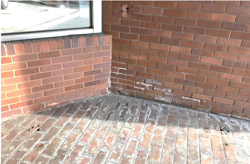
Figure 46. Mortar erosion, efflorescence, and spalled brick units near base of wall at stairwell.
