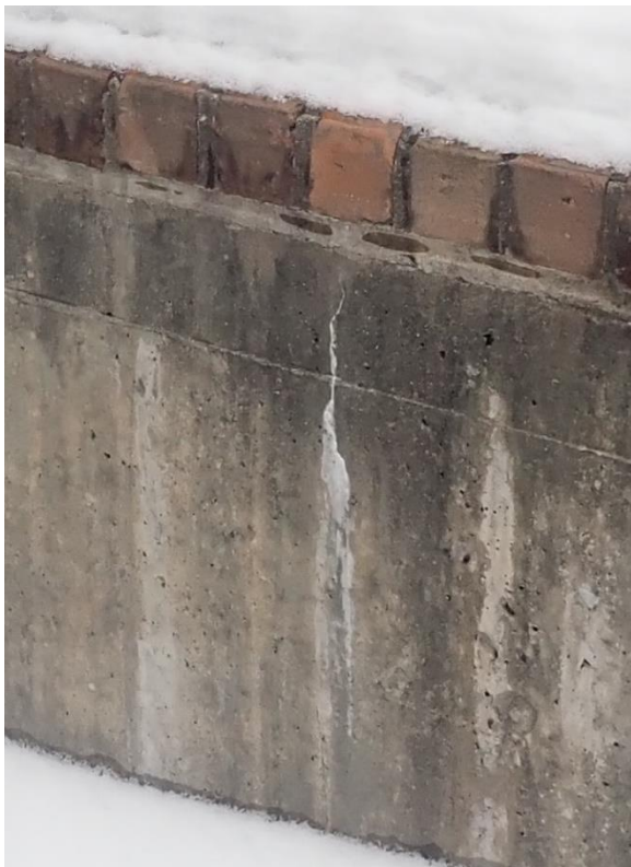
Figure 22. Crack with efflorescence staining on perimeter wall.
