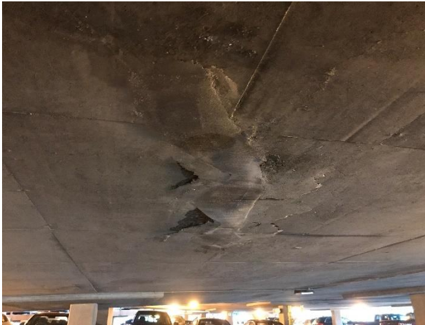
Figure 10. Unsound (delaminated) previous repair.
