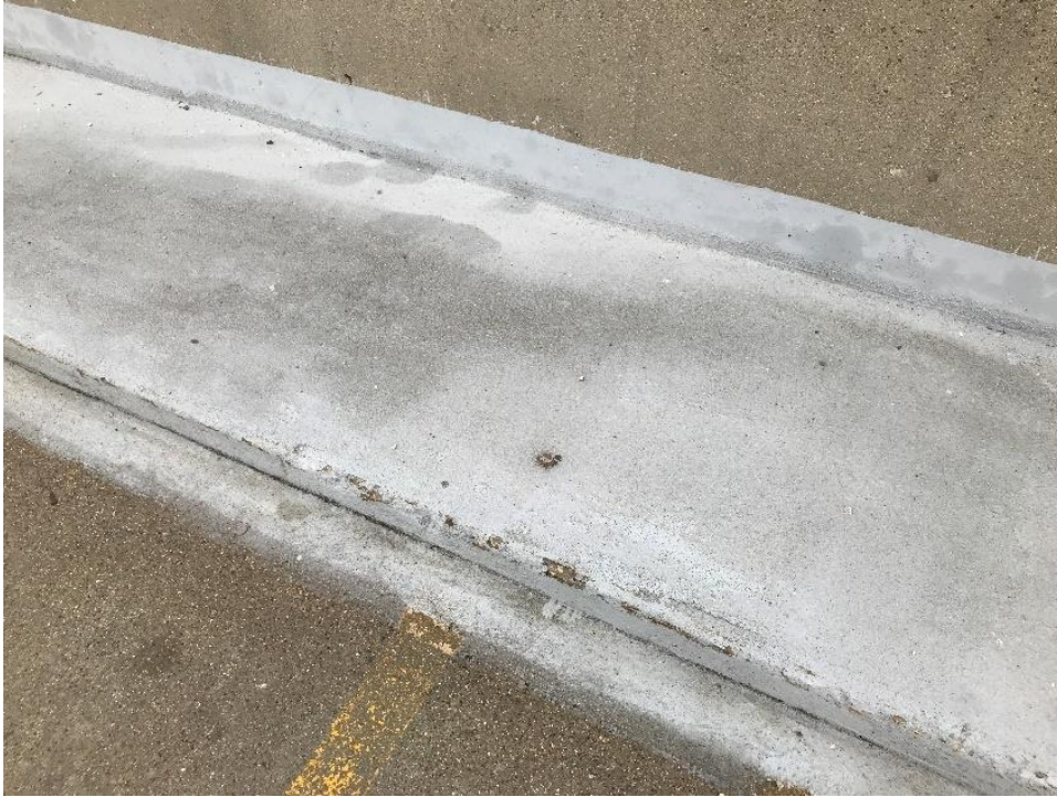
Figure 21. Area of membrane scrapes at a concrete curb on Level 5.
