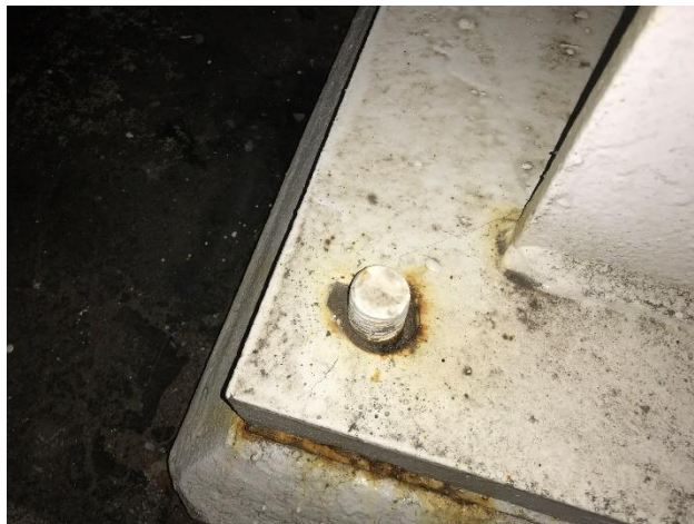
Figure 38. Missing nut at base plate
