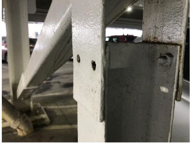
Figure 60. Missing bolt at flange plate at intermediate post splice
