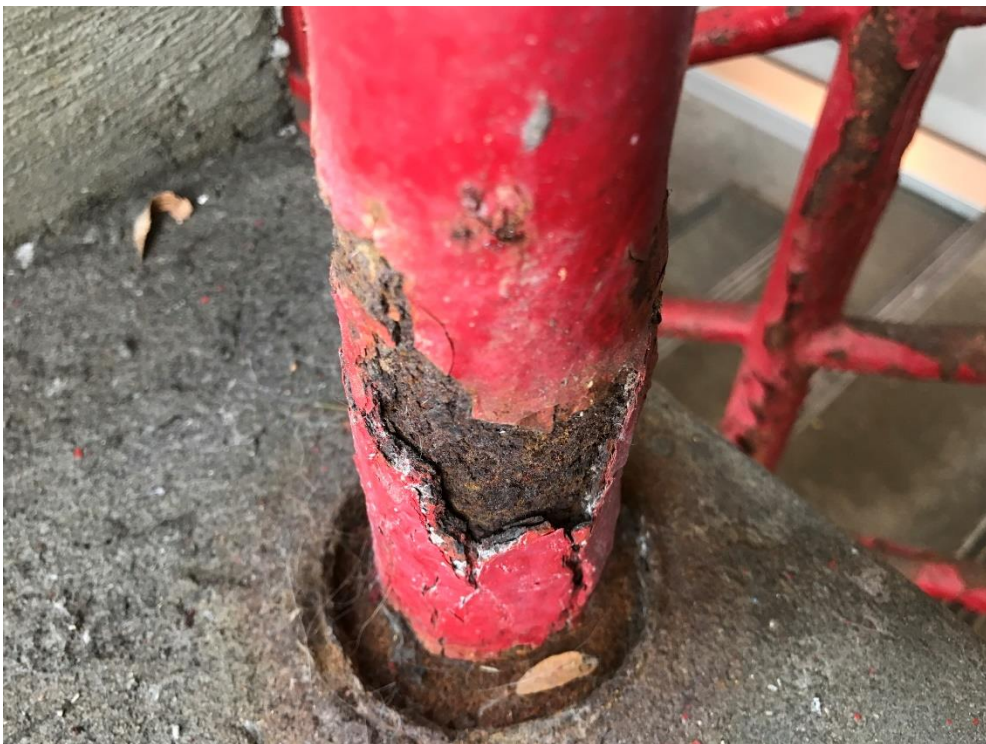
Figure 51. Corrosion at base of stairwell railing post.
