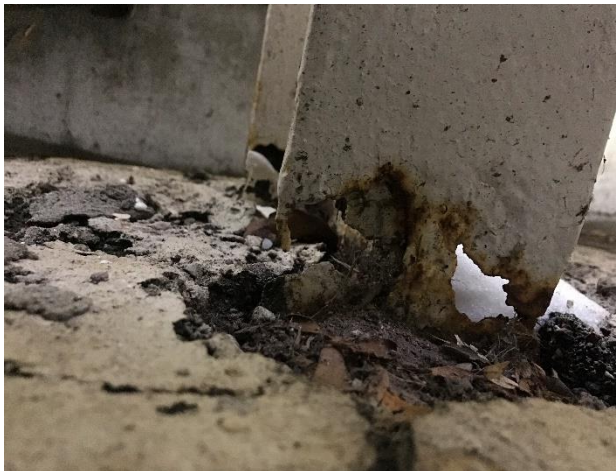
Figure 54. Severe section loss at intermediate post
