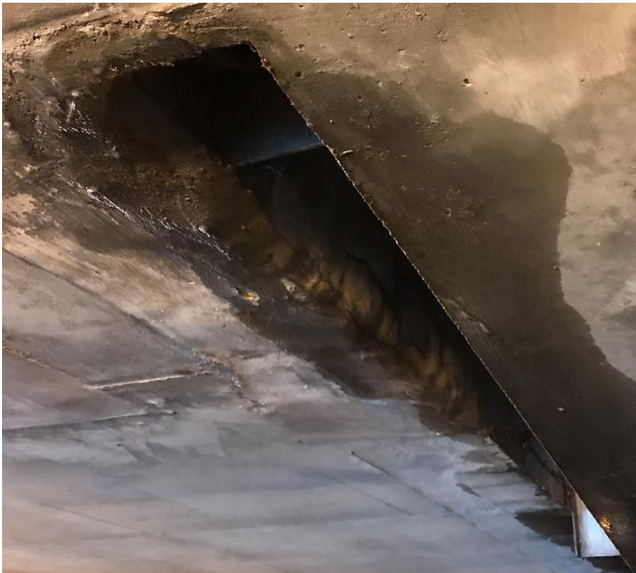
Figure 12. Unsound and cracked previous repairs at the interior slab edges.
