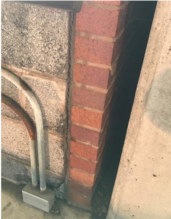
Figure 43. Cohesively failed sealant between CMU wall and brick veneer.
