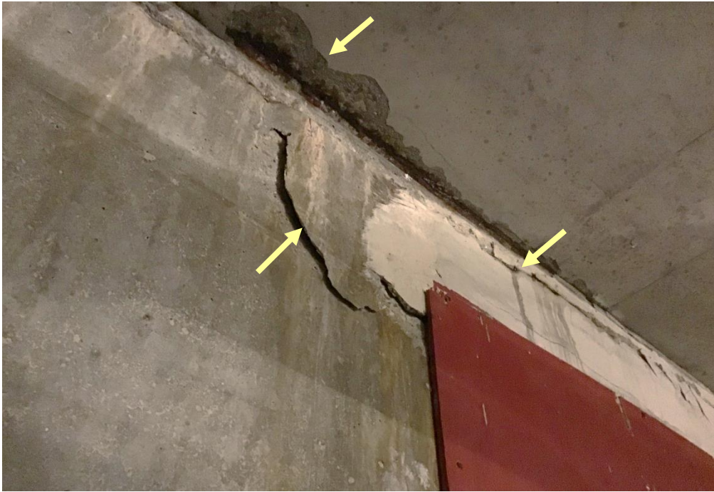
Figure 29. Concrete spall and water staining at foundation wall.
