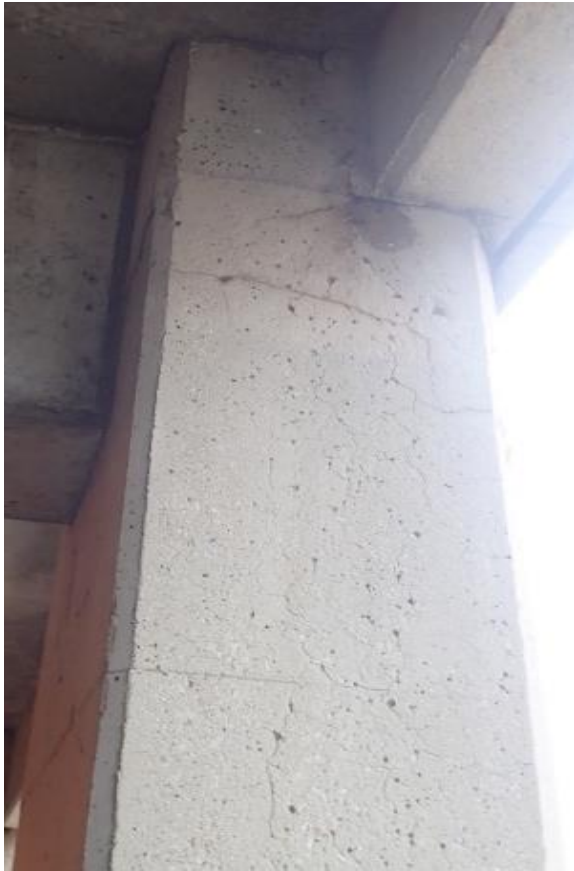
Figure 19. Shrinkage cracks on exterior column, Tier 2.
