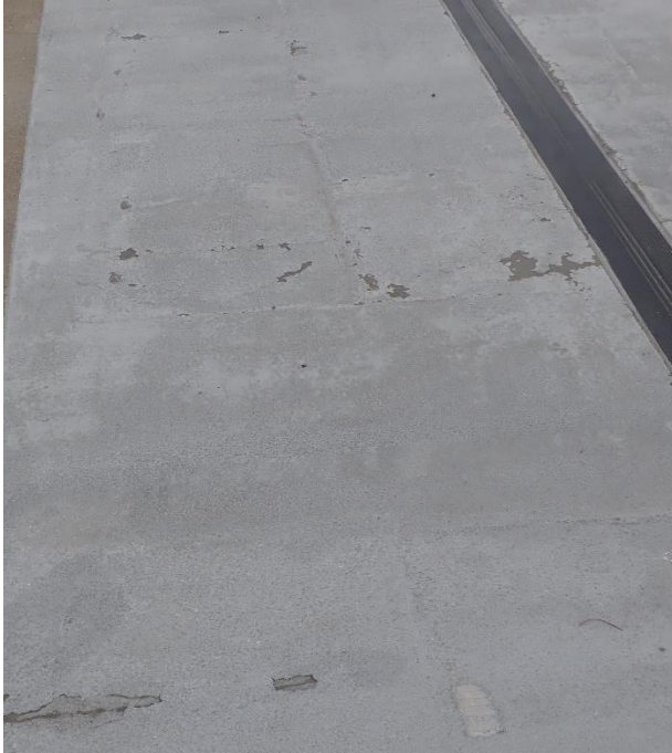
Figure 27. Worn and delaminated coating at Tier 4 expansion joint.
