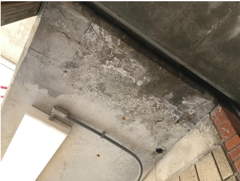
Figure 53. Cracking and efflorescence at underside of stair flight.
