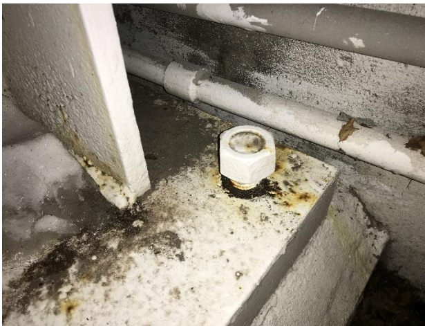
Figure 37. Loose nut at base plate
