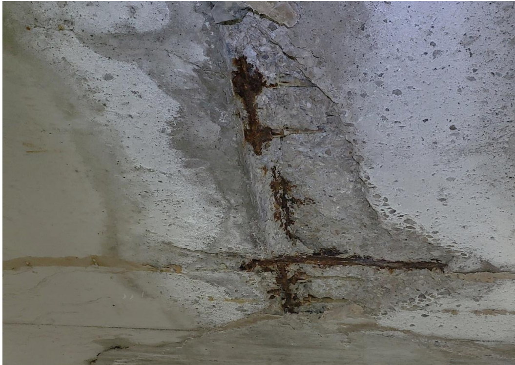
Figure 2. Spall at construction joint exposing PT tendon anchorages and an embedded conduit
