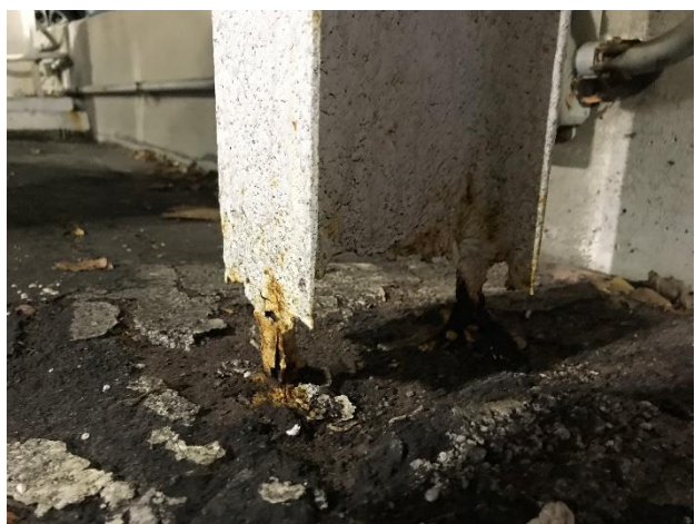
Figure 55. Severe section loss at intermediate post
