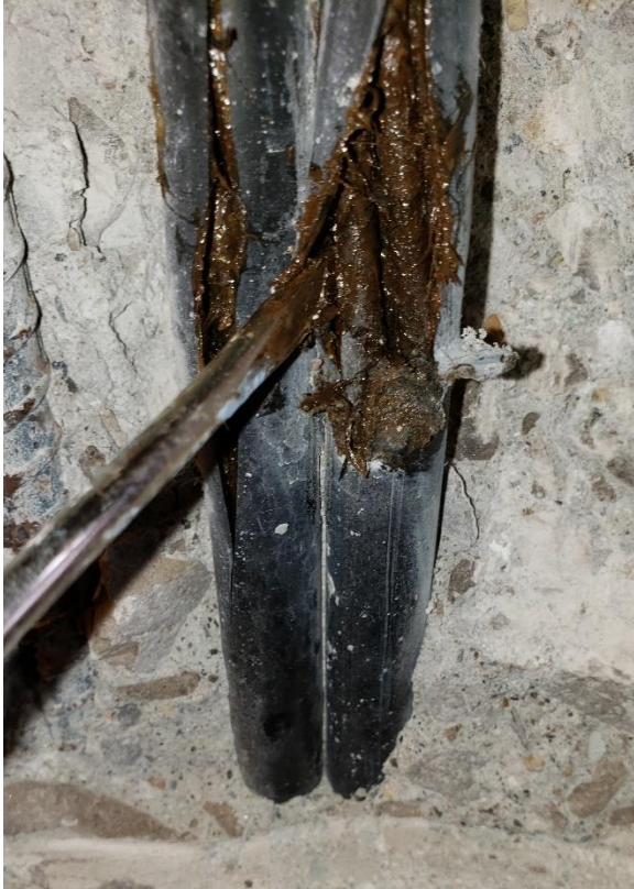
Figure 11. Exposed tendons at Inspection Opening 6 with corrosion byproducts emulsified in the grease.
