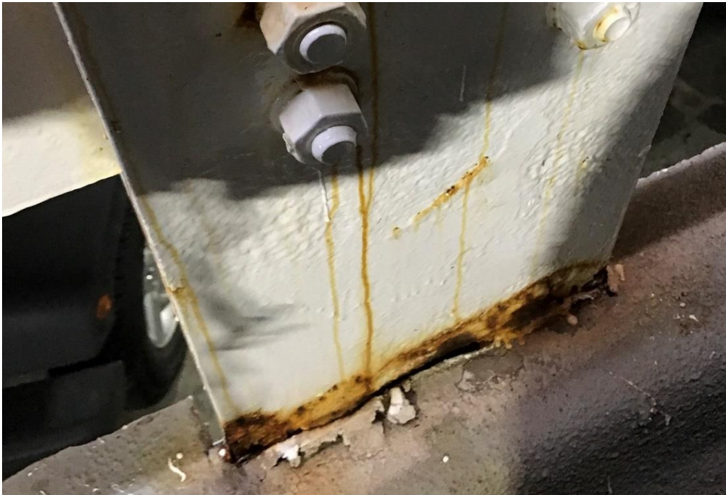
Figure 43. Corrosion where interior column contacts slab edge
