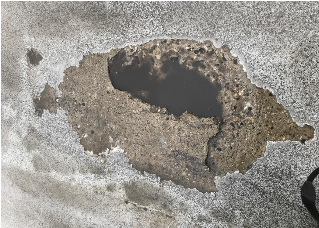
Figure 29. Spall at topside of roof level slab
