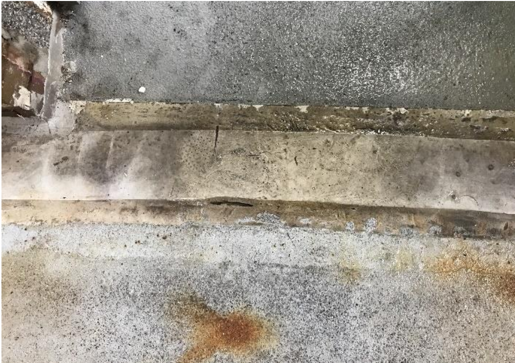
Figure 68. Failed stairwell expansion joint
