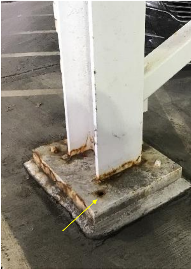
Figure 39. Missing bolt at base plate
