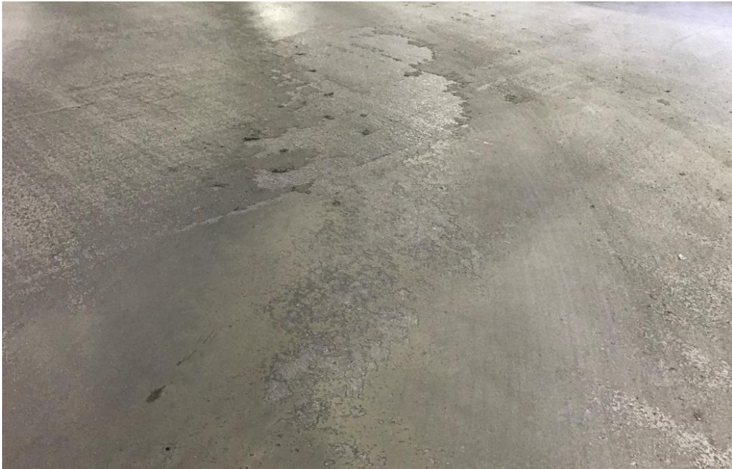
Figure 66. Worn and failed traffic-bearing membrane at Level 2 turnaround
