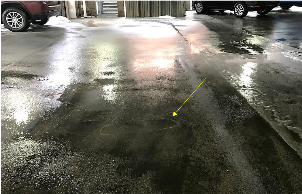
Figure 28. Delamination near drain within ponded water (indicated with arrow)
