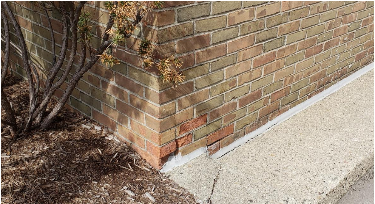
Figure 24. Spalled brick masonry at exterior of a stair tower.
