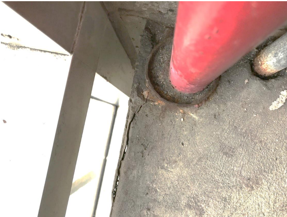
Figure 49. Spall at corroded stairwell handrail embed at landing.
