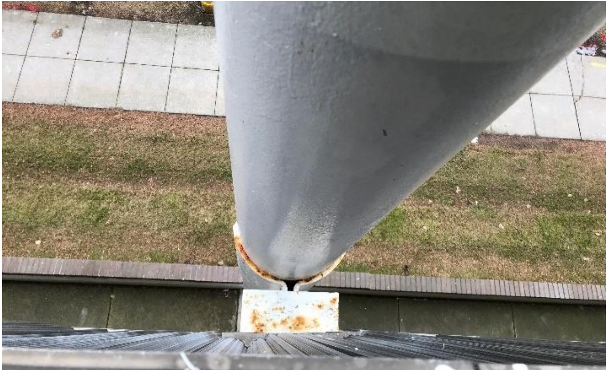
Figure 49. Corroded connection at exterior column
