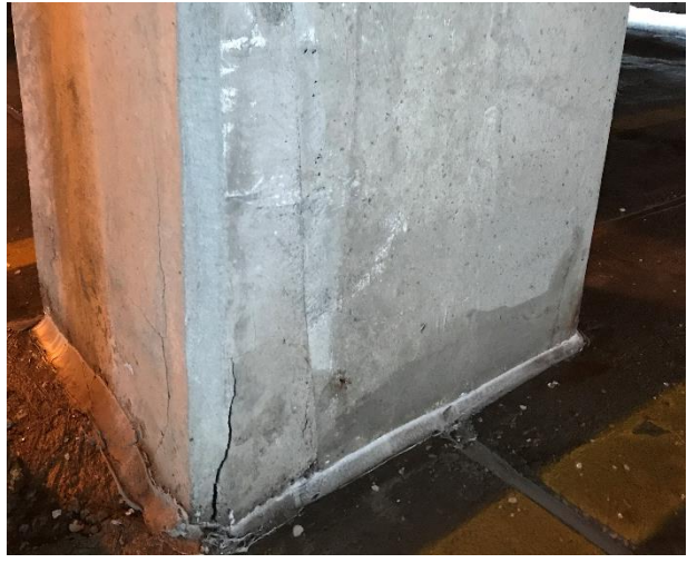
Figure 14. Cracked previous repair.
