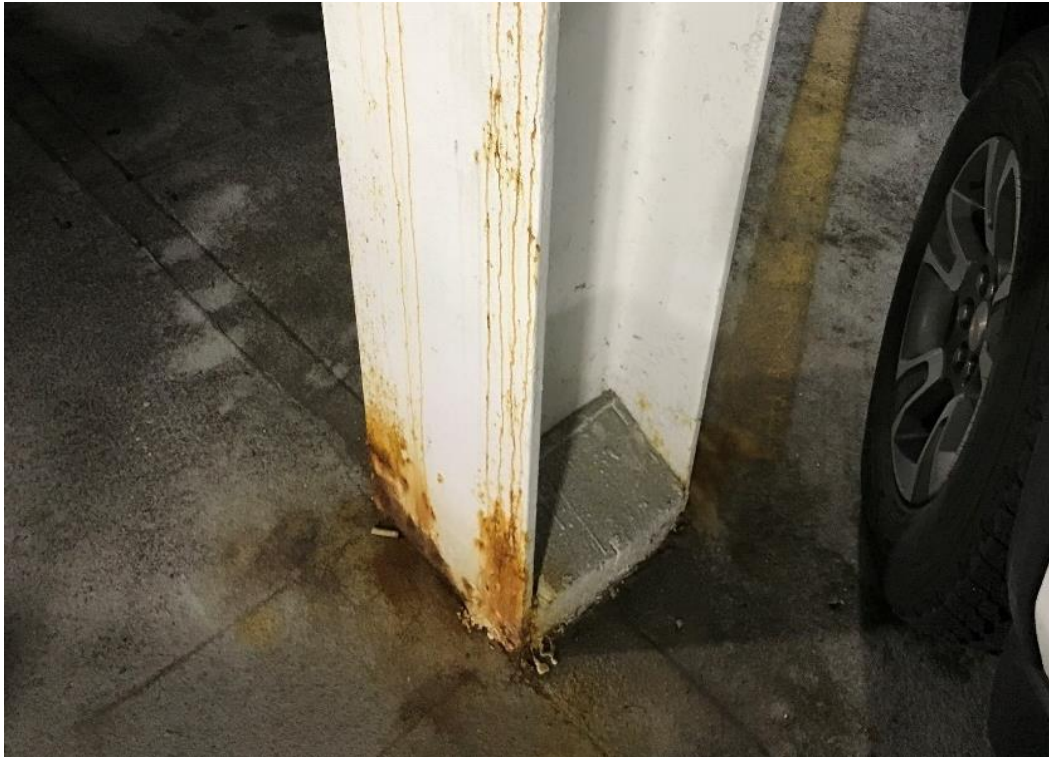
Figure 44. Corrosion at interior column base at elevated slab
