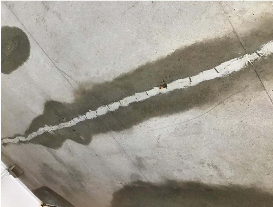
Figure 36. Moisture staining at previous repaired crack at conduit.
