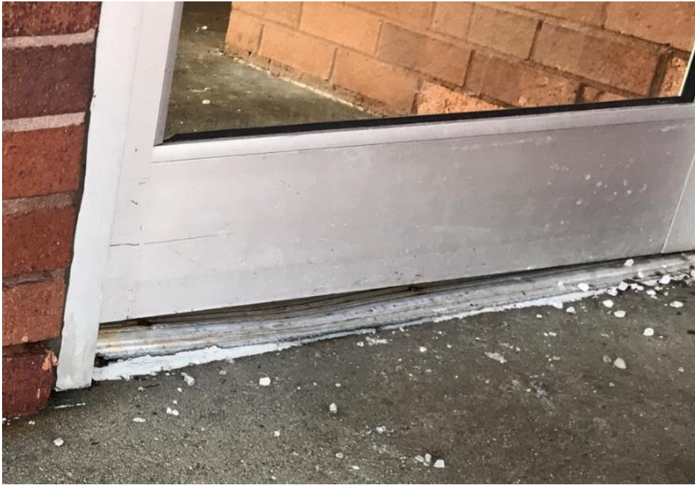
Figure 48. Deformed door threshold at stairwell entry.
