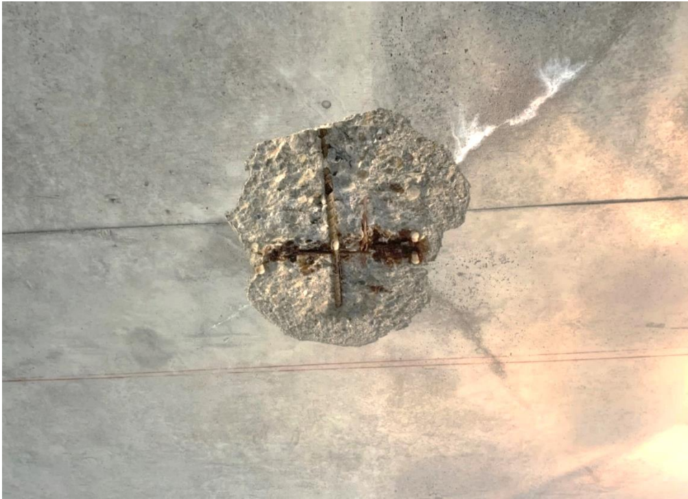
Figure 13. Exposed Tendon Location 1
