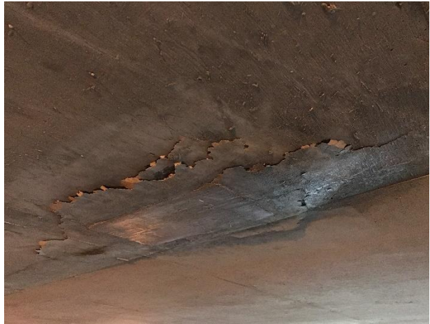
Figure 11. Unsound (delaminated) previous repair with unsound concrete extending beyond the previous repair area.
