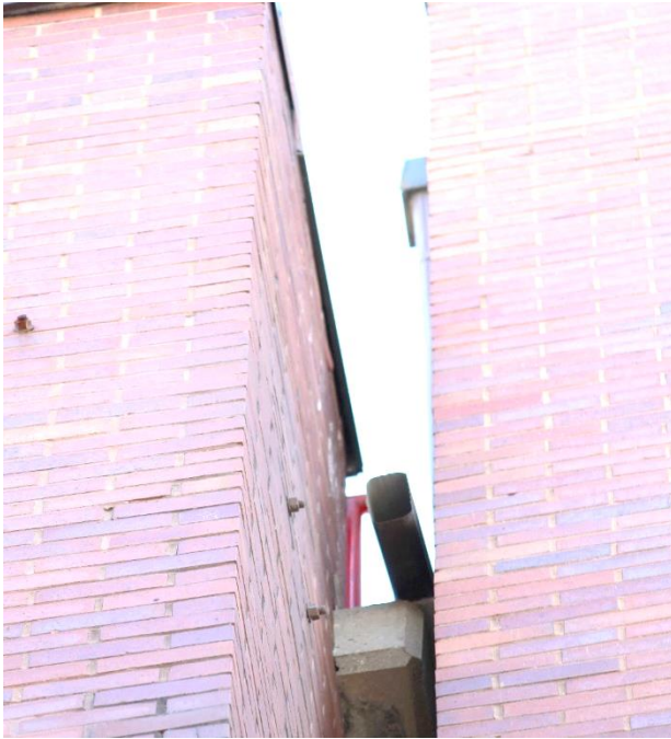
Figure 35. Stair tower roof downspout discharge.
