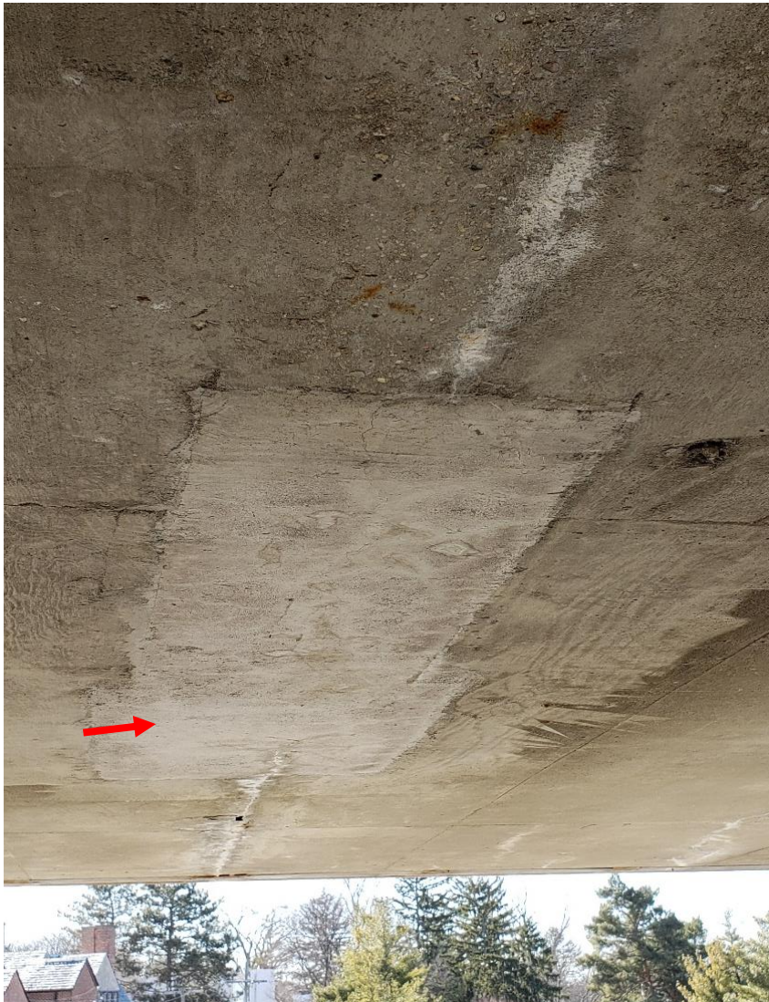
Figure 6. Previous concrete repair and unsound concrete (indicated by the arrow) in line with a crack with efflorescence.
