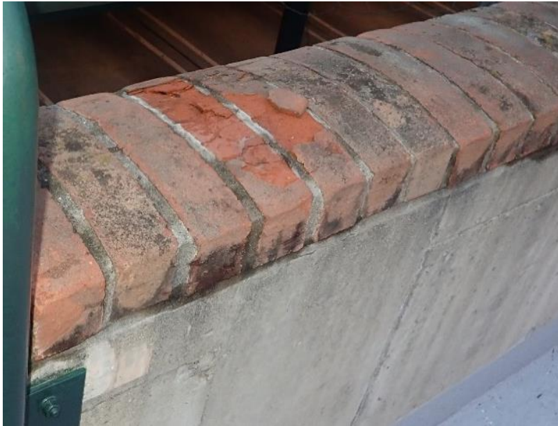
Figure 35. Cracked and spalled brick coping on concrete spandrel beam, Tier 2.
