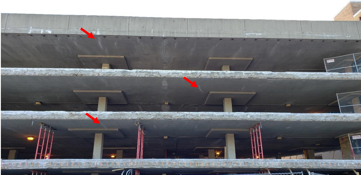
Figure 5. West elevation during slab edge repairs. Note the multiple cracks with efflorescence. A few locations are indicated by arrows. This photo was taken during the installation of the cable barrier system.
