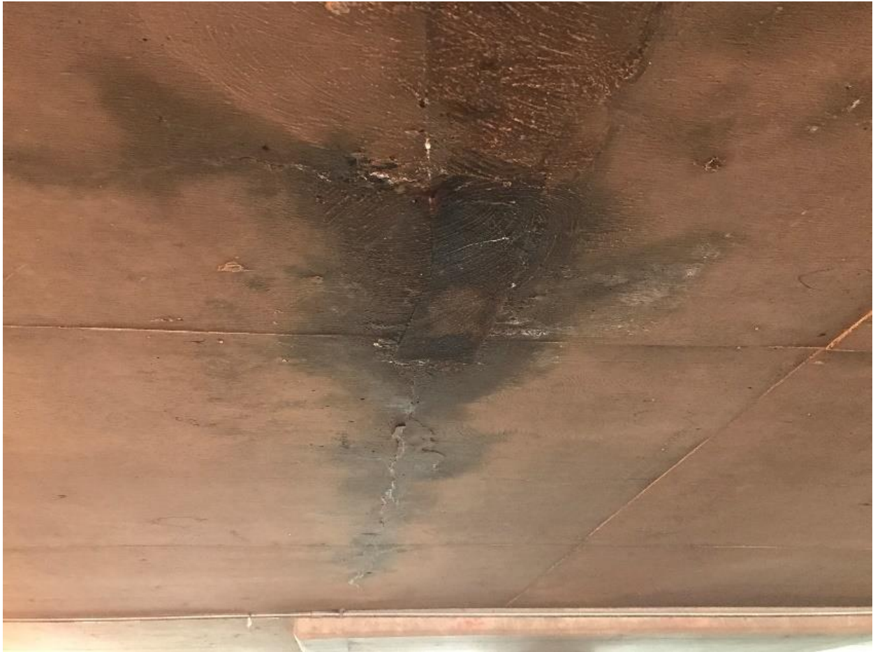
Figure 20. Active water leak at a previous repair area.
