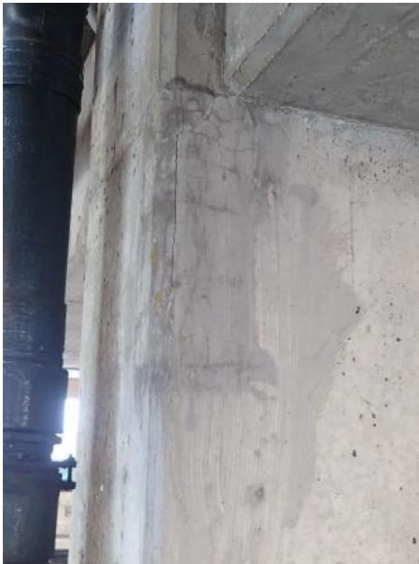
Figure 14. Unsound concrete patch at top of column, Tier 3.
