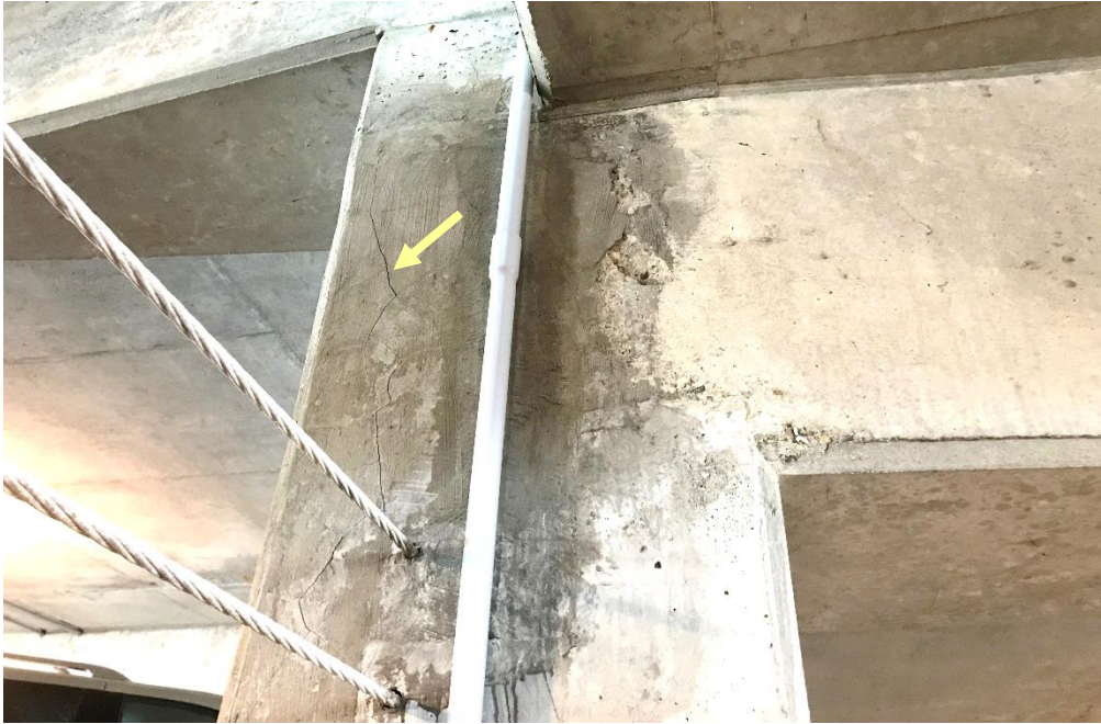
Figure 27. Deterioration within a large concrete patch repair at an interior column.
