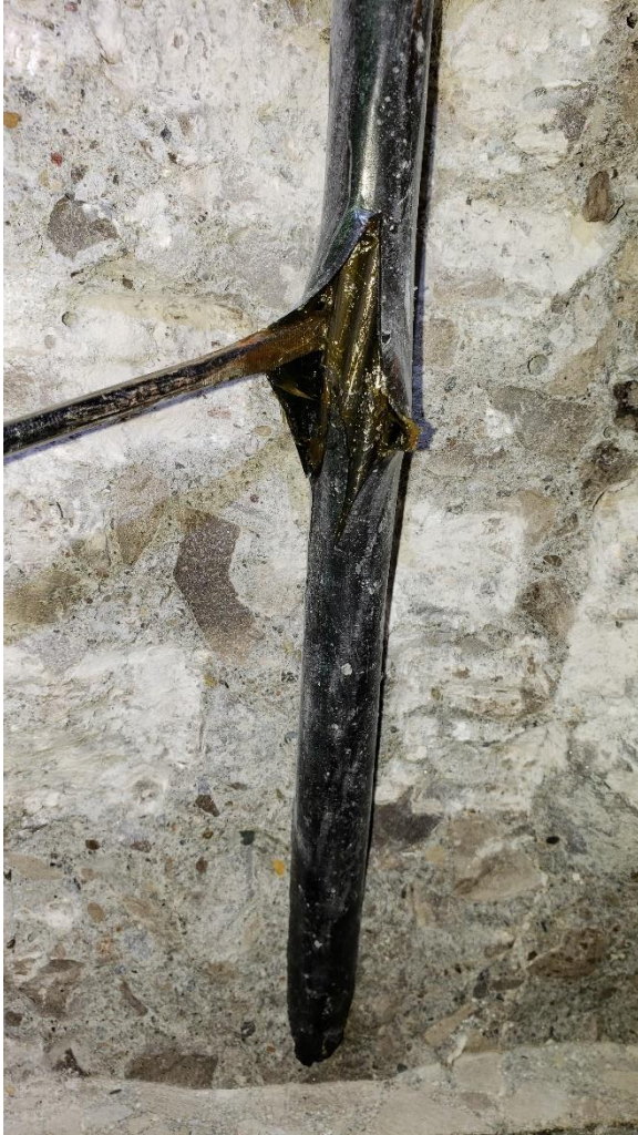
Figure 8. Typical good tendon condition at Inspection Openings 1, 2, and 4.
