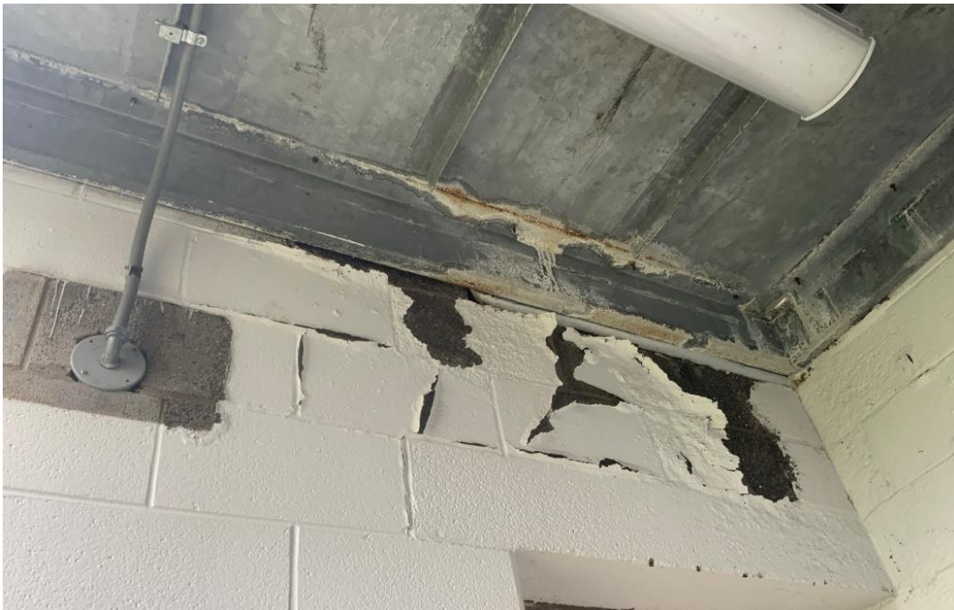
Figure 69. Failed coating at CMU stair tower wall below expansion joint seal
