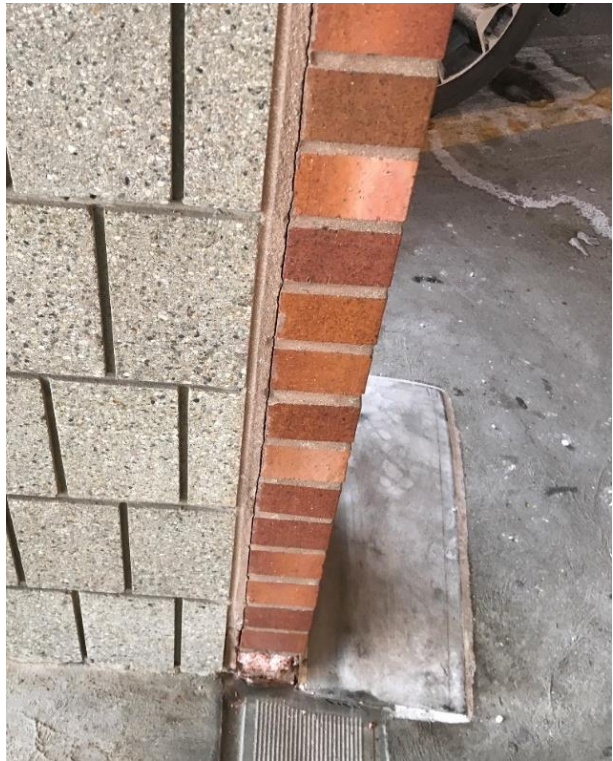
Figure 44. Typical debonded mortar joint between facade and stairwell.
