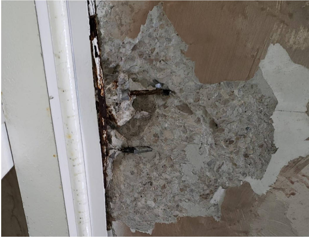
Figure 1. Spall at slab edge exposing PT temperature tendons
