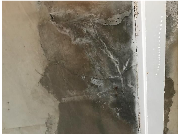
Figure 26. Previous repair exhibiting cracking and efflorescence
