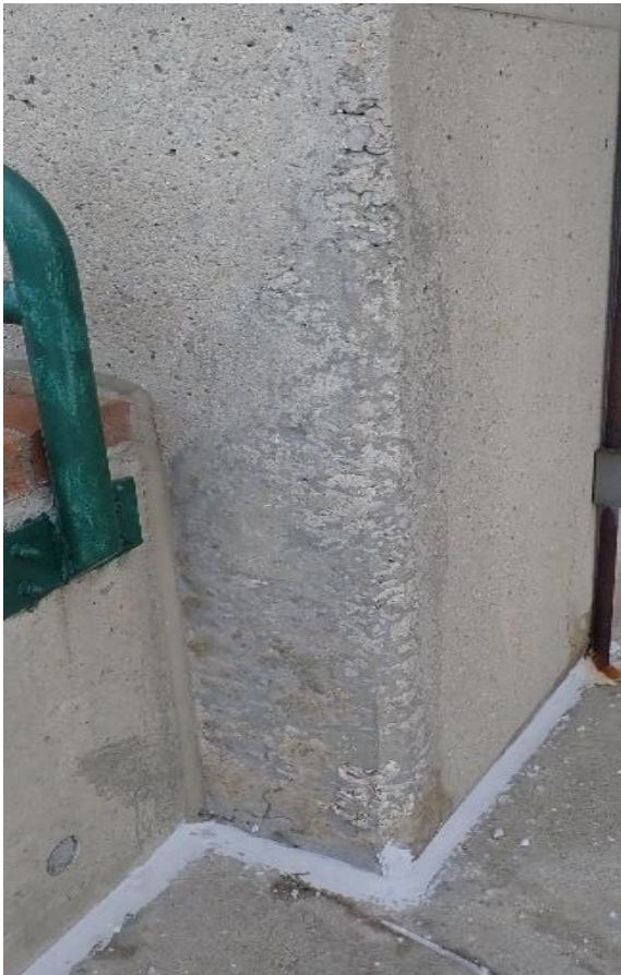
Figure 16. Isolated concrete honeycombing in concrete column.
