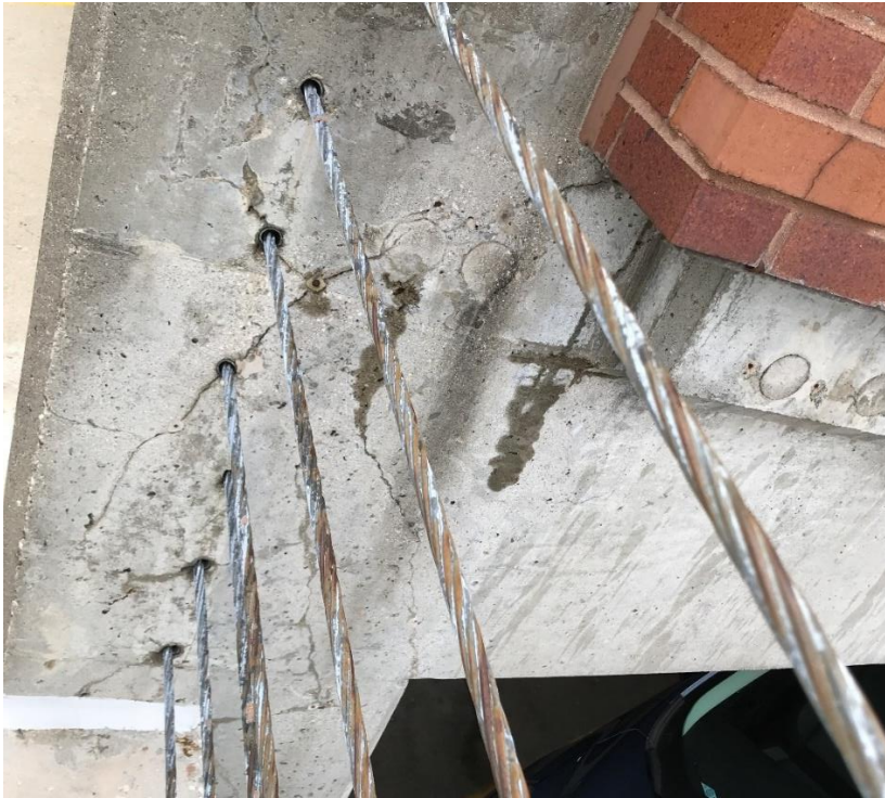
Figure 23. Cracking and water staining at a beam-column intersection.
