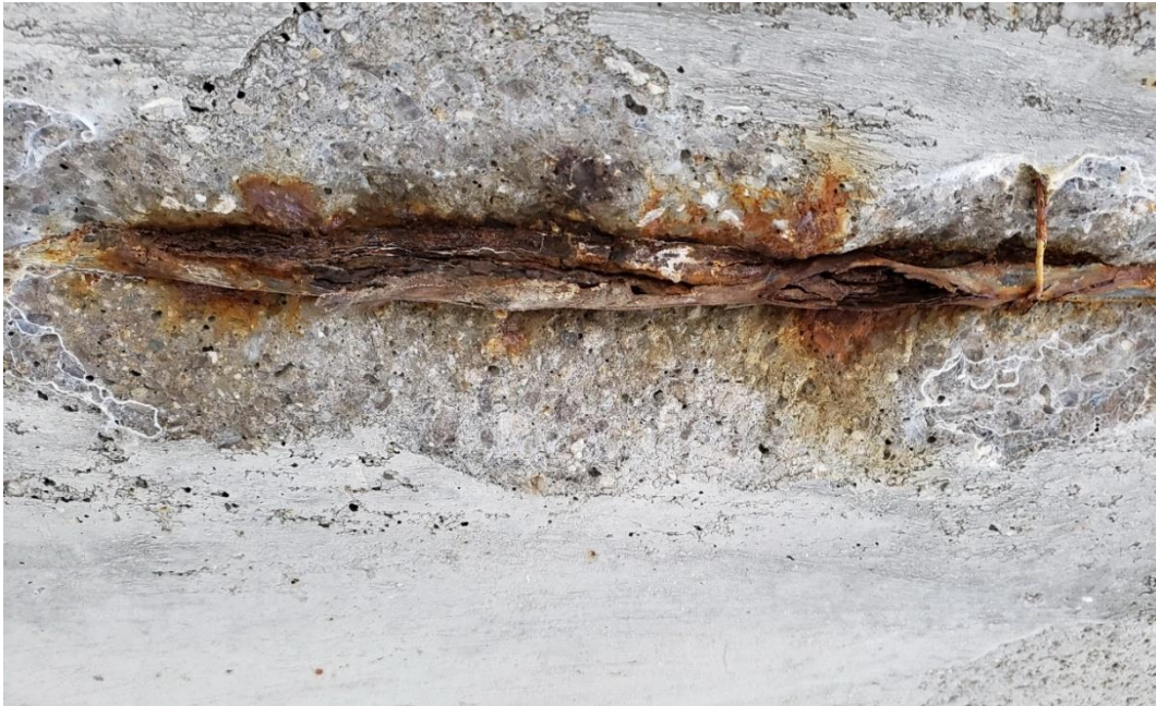
Figure 13. Exposed Tendon Location 3
