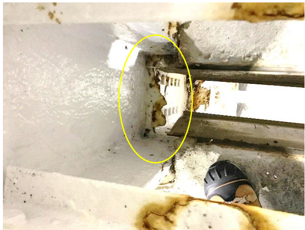
Figure 48. Nearly full section loss of top column stiffener plate
