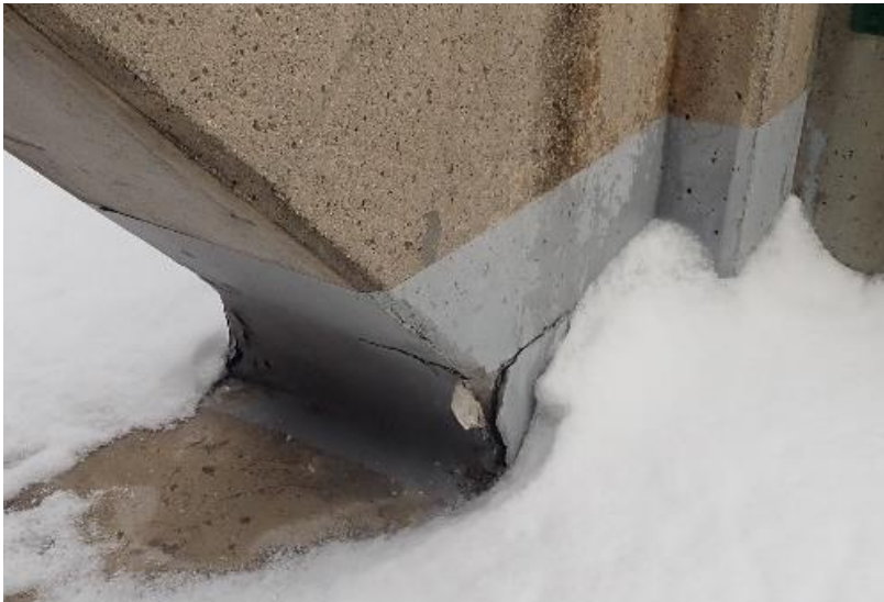
Figure 18. Delaminated coating and unsound concrete at base of inclined column supporting Tier 4.
