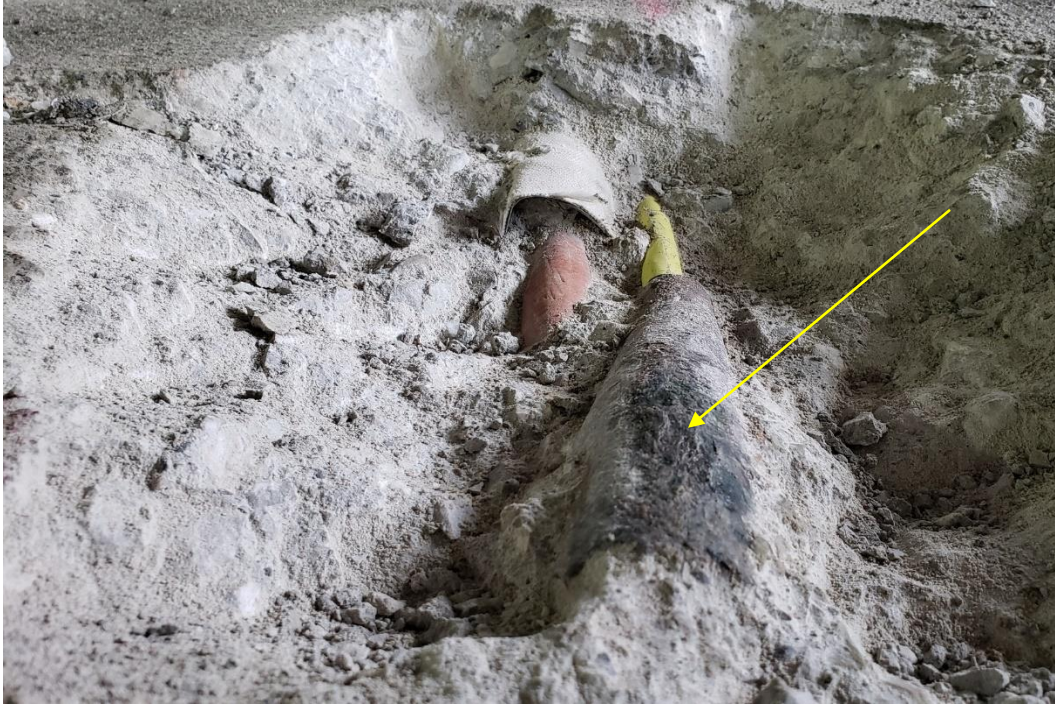
Figure 17. Inspection Opening 1. PT tendon coupler indicated by arrow.
