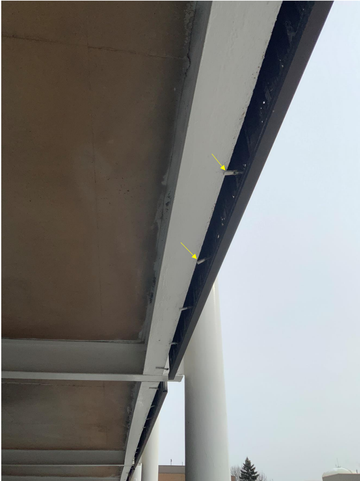
Figure 74. Failed welds and gaps at tie-backs
