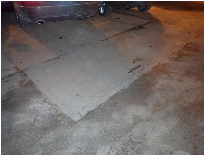
Figure 34. Unsound and cracked partial-depth concrete repair at Tier B.
