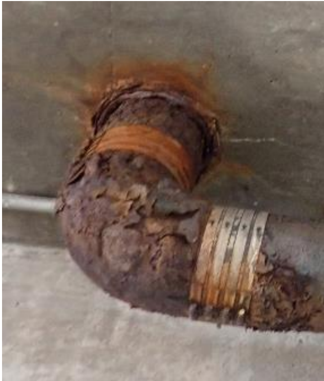
Figure 33. Corrosion product from floor drain bowl above.
