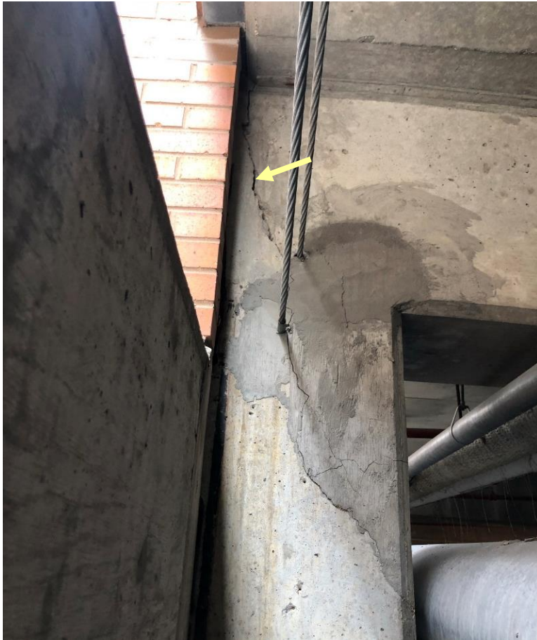
Figure 25. Cracking with column on the Lower Level.
