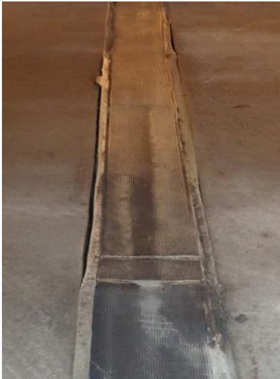
Figure 24. Adhesively failed edges of pre-molded expansion joint seal.
