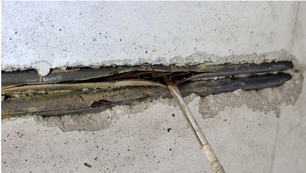
Figure 11. Exposed Tendon Location 1
