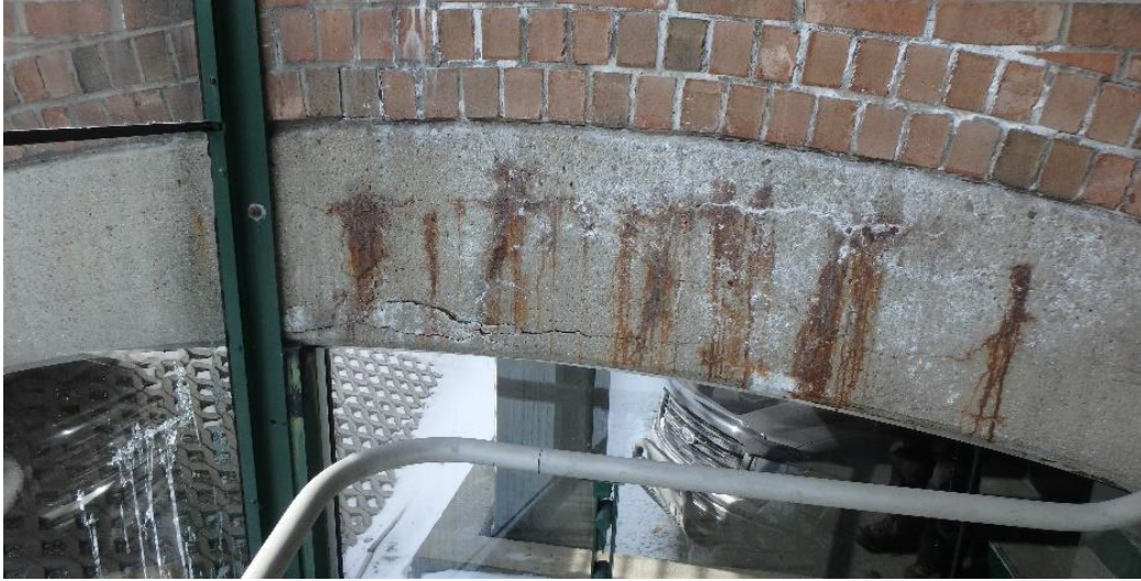
Figure 15. Typical area of unsound concrete, cracking, and corrosion and efflorescence staining on arched beam supporting pedestrian bridge.
