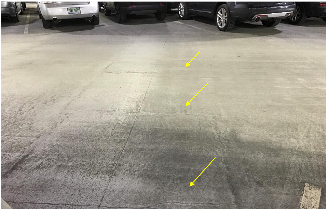
Figure 7. Evenly spaced previous crack repairs at Level 3 construction joint, in line with PT tendons
