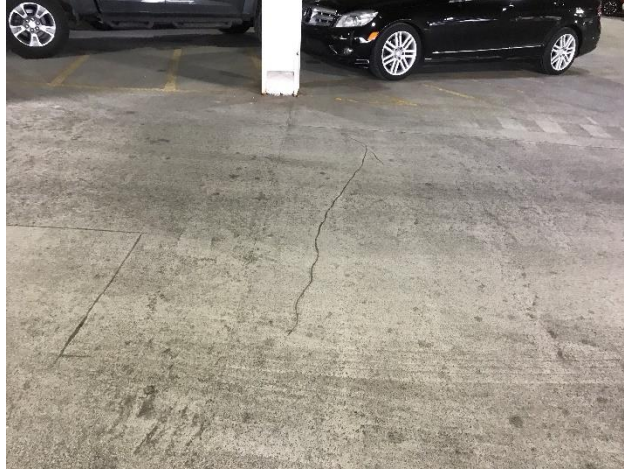
Figure 34. Previously sealed cracks
