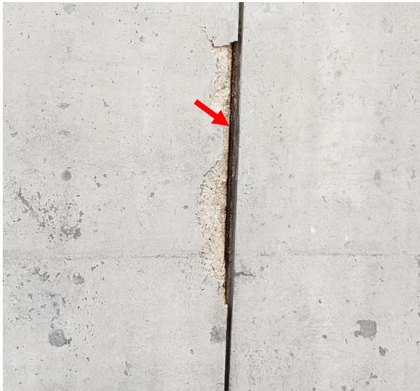
Figure 15. Spall at an exterior wall joint with an exposed corroded reinforcing bar indicated by the arrow.
