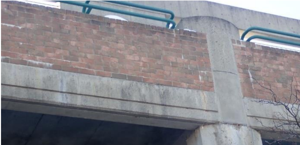
Figure 37. Efflorescence, staining and eroded mortar joints, west elevation.
