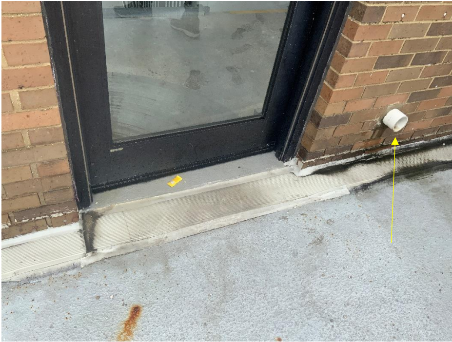
Figure 70. Roof drain outlet above expansion joint
