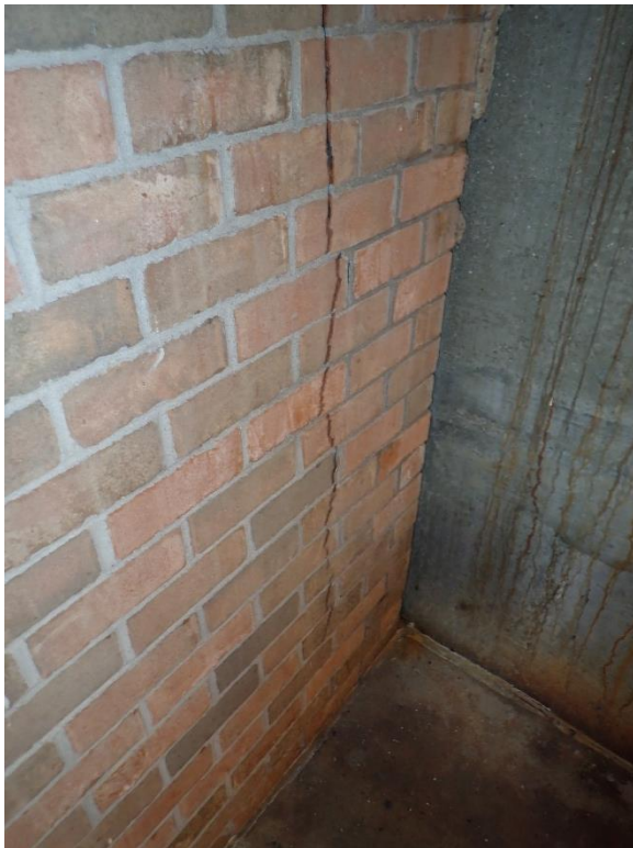
Figure 38. Vertical crack between southeast stairwell common wall and deck, Tier A.
