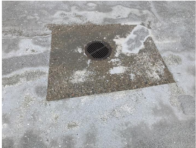
Figure 24. Previous repair at roof drain
