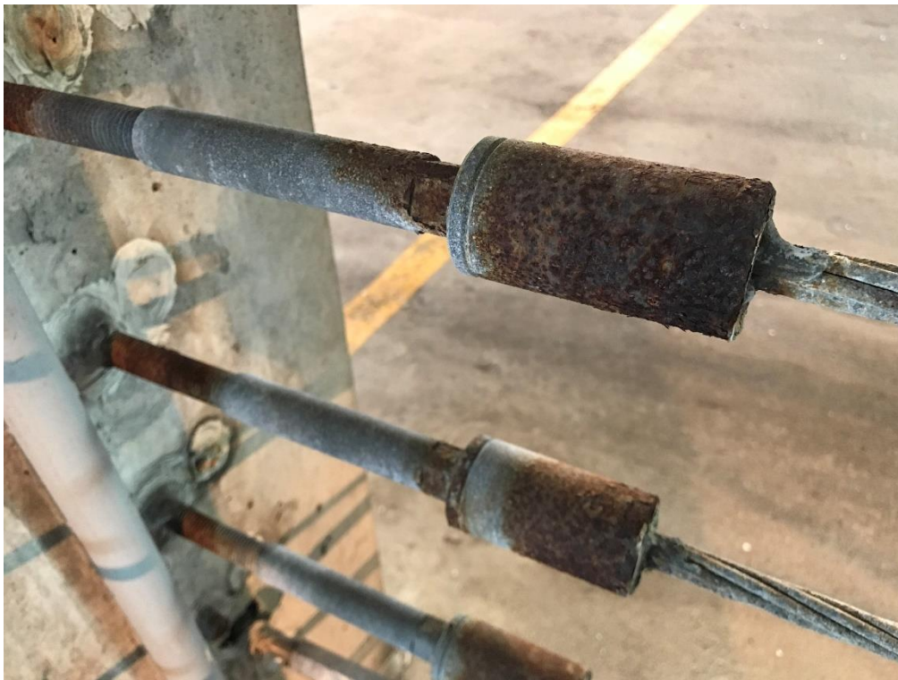
Figure 55. Corrosion of vehicle barriers and splice couplers.
