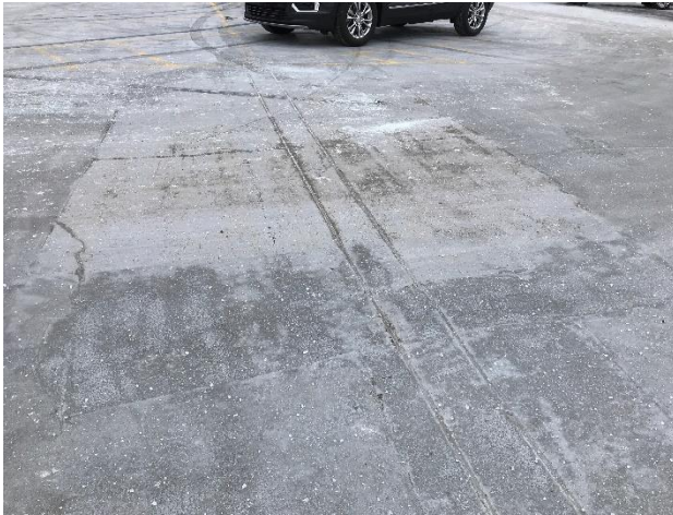
Figure 23. Previous repair at construction joint
