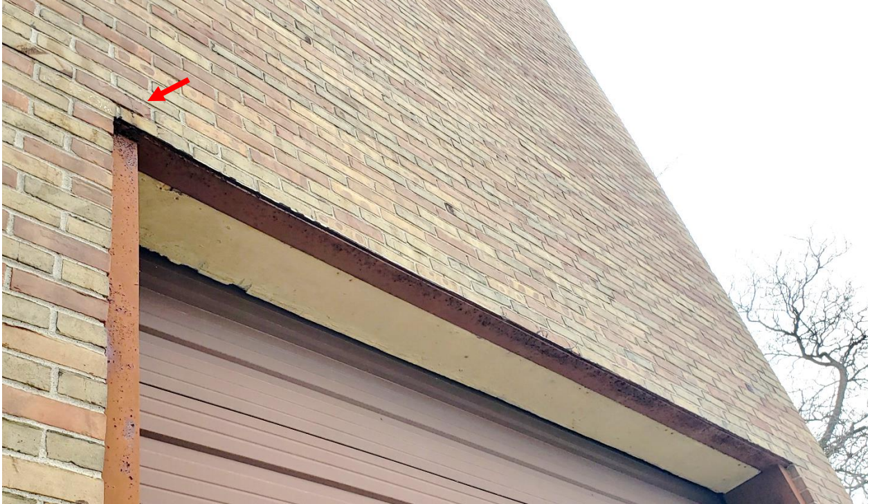
Figure 23. Corroding steel lintel and cracked brick masonry at ends (indicated by the arrow).
