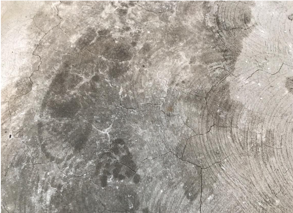
Figure 52. Crazing cracking at Level 7 stairwell landing surface.
