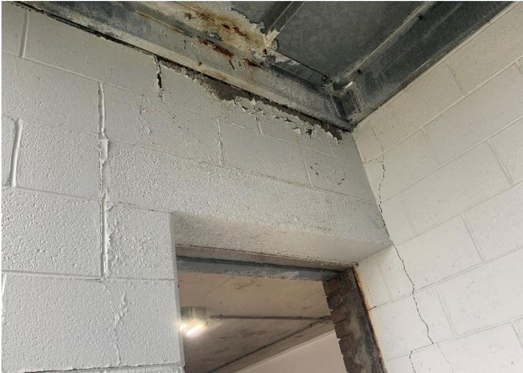
Figure 80. Cracks in CMU stair tower walls near corroded steel
