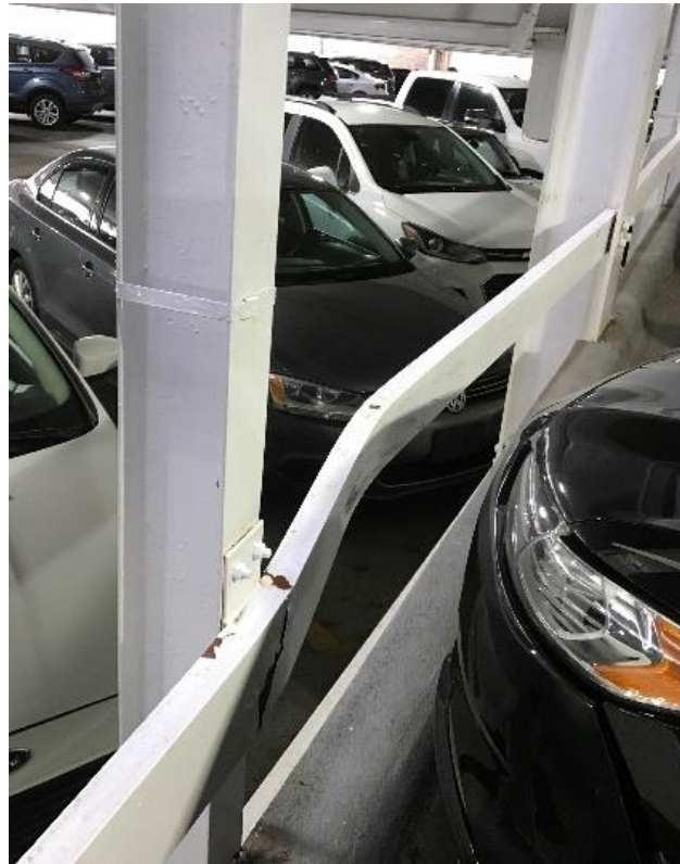
Figure 64. Vehicle impact at guardrail
