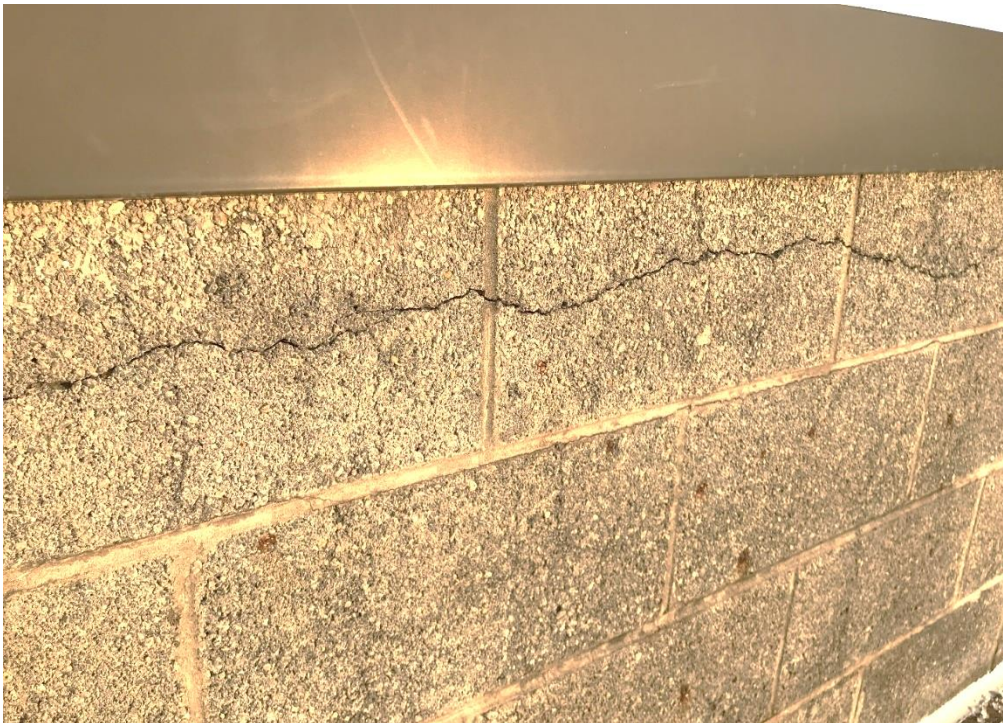
Figure 28. Cracking at CMU facade wall prior to recent coating of wall surface.
