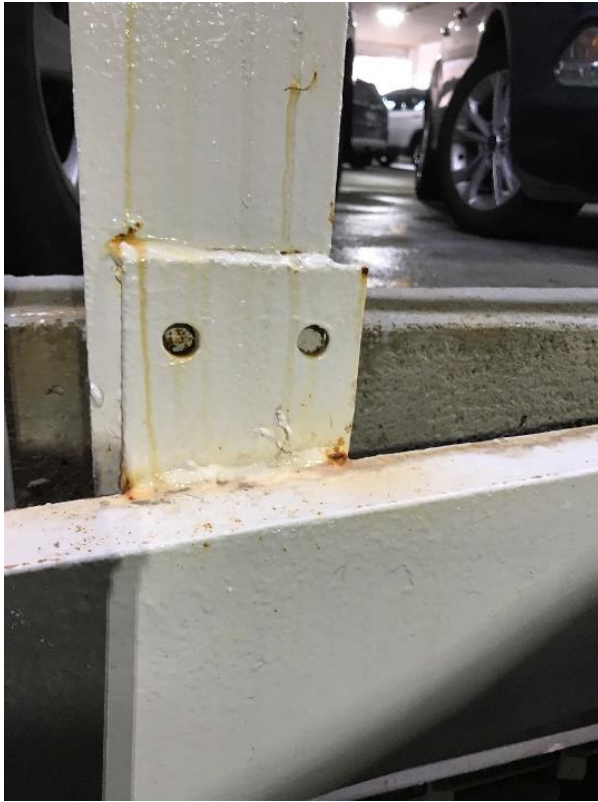
Figure 63. Missing bolts at channel to post connection, but welds present
