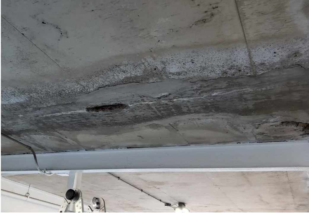
Figure 3. Spall at a previous repair exposing PT tendon
