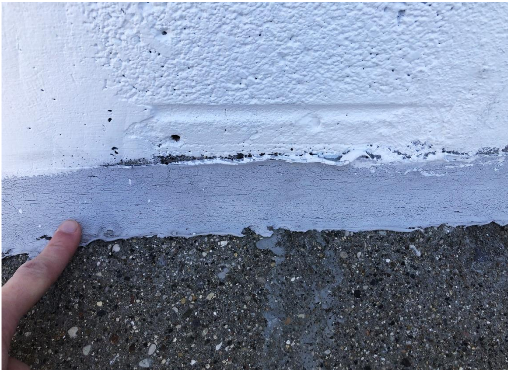
Figure 20. Water staining at perimeter joint between slab and wall intersection.
