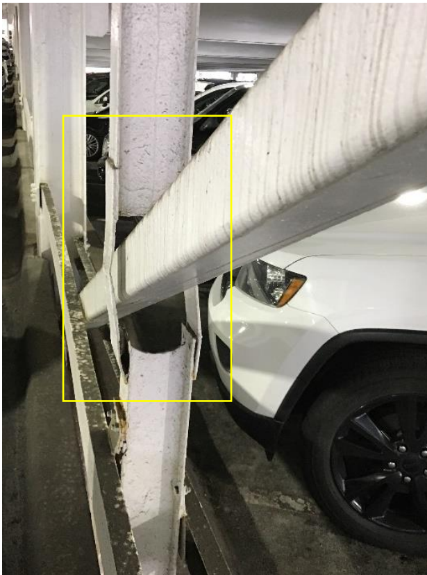
Figure 57. Deformed intermediate post splice
