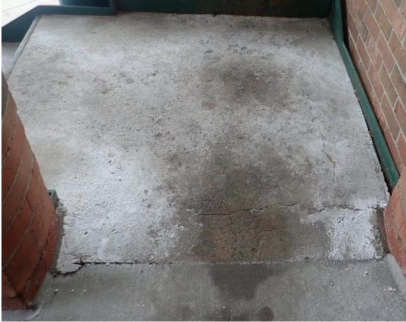
Figure 39. Cracked and eroded concrete stair landing.
