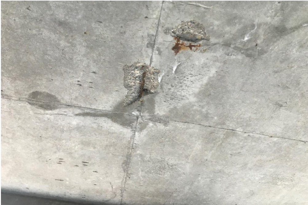
Figure 5. Exposed, corroded mild reinforcement at spall in underside of slab between beams.
