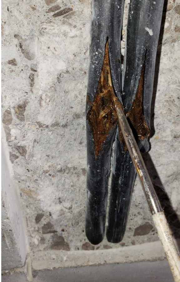
Figure 10. Exposed tendons at Inspection Opening 5 with corrosion byproducts and emulsified grease.
