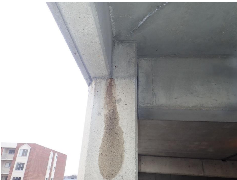
Figure 20. Active water infiltration where spandrel beam bears on column.
