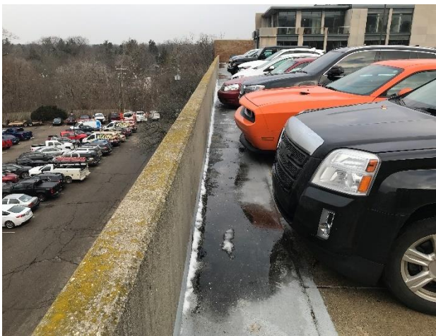
Figure 18. Ponding water on roof slab at a concrete curb.
