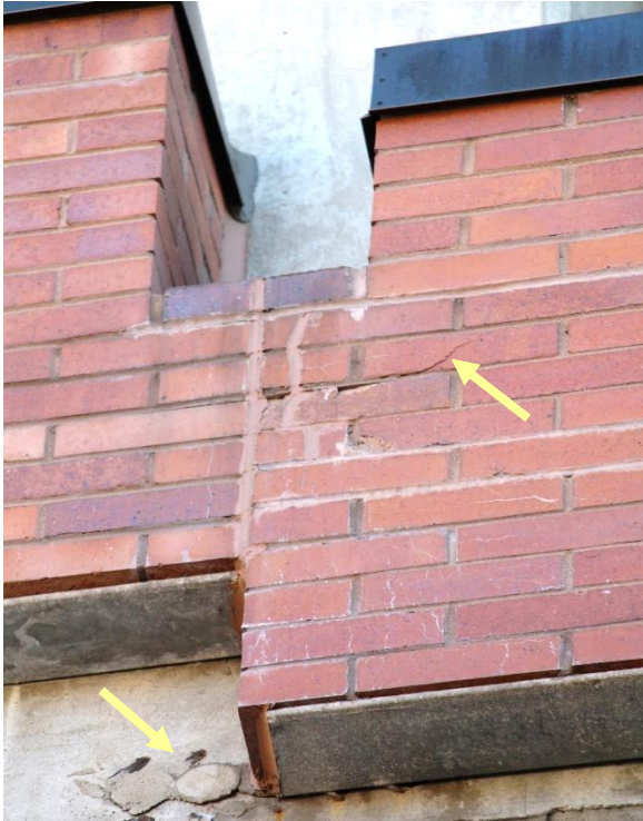
Figure 39. Brick distress at vertical discontinuity. Note shrinkage cracks around slab grout pockets.
