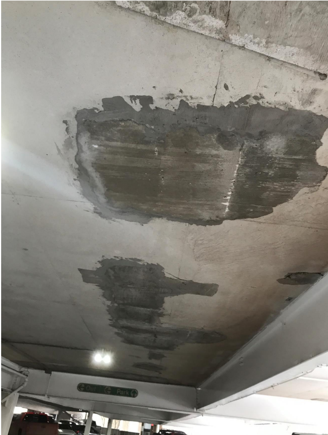
Figure 5. PT intermediate anchorage repairs at a construction joint, as viewed from the underside of Level 4
