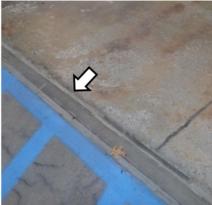
Figure 25. Arrow indicates adhesively failed pre-molded expansion joint seal near elevator shaft.
