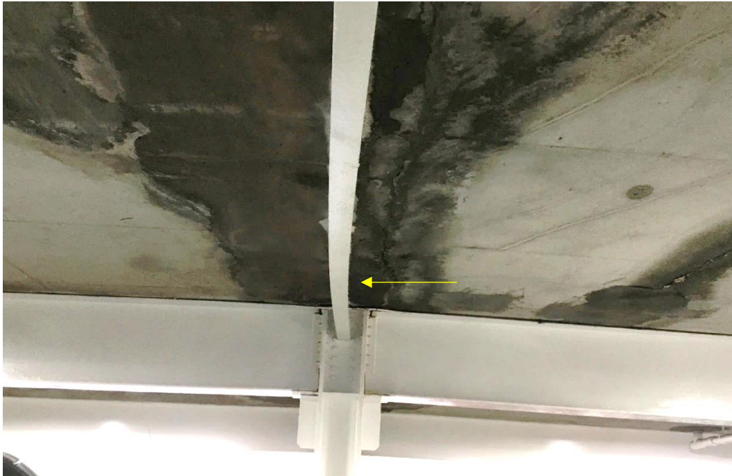
Figure 53. Laterally deformed steel beam
