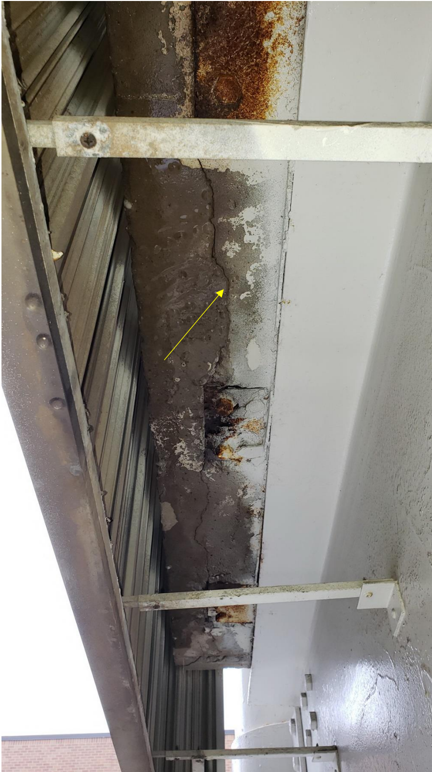
Figure 32. Cracked concrete at slab edge
