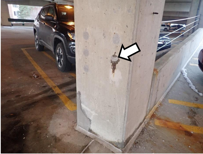
Figure 41. Arrow indicates grease staining from grout pocket for vehicle barrier cable.
