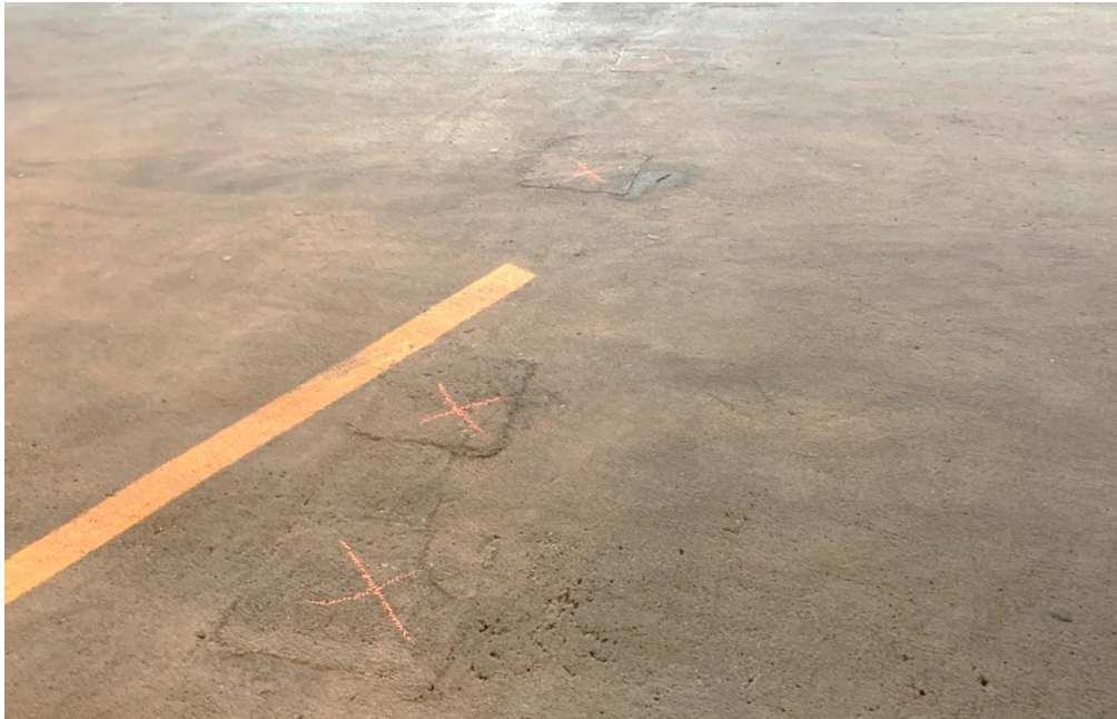
Figure 3. Unsound previous repairs along the top of a beamline.
