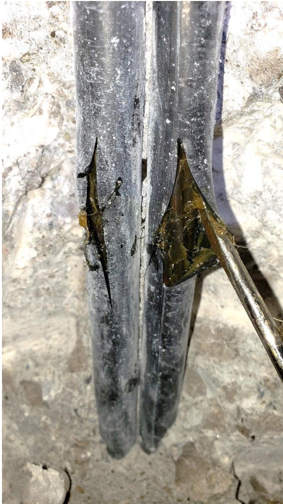
Figure 9. Exposed tendons at Inspection Opening 3.
