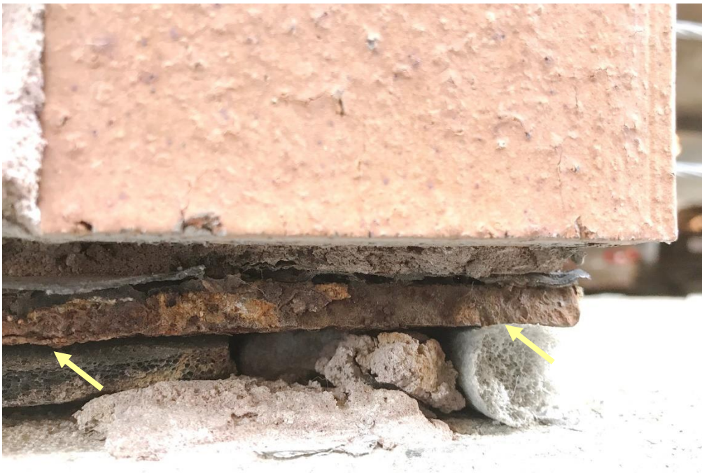
Figure 30. Steel corrosion and section loss of shelf angle near grade.
