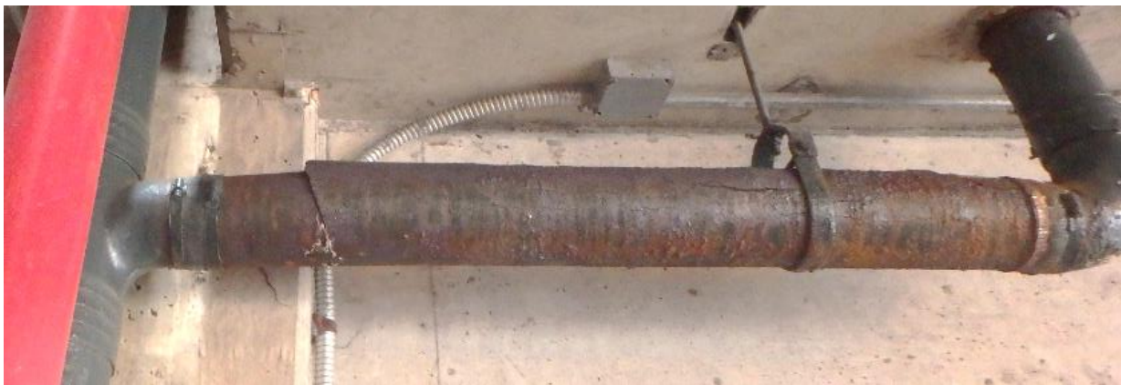
Figure 32. Cracked floor drainage pipe with corrosion product.
