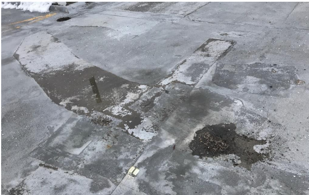
Figure 65. Traffic-bearing membrane failure at previous concrete repair
