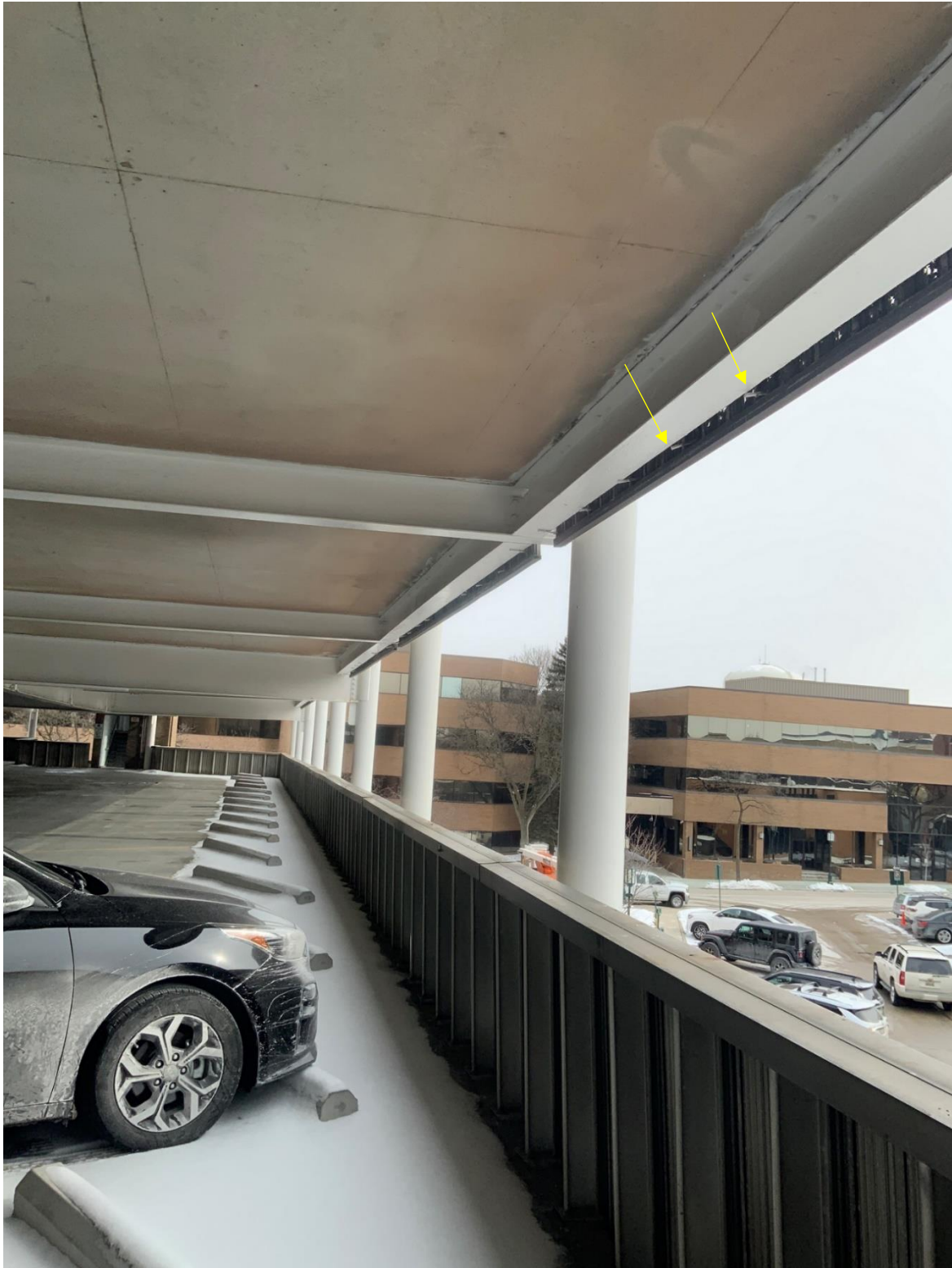
Figure 73. Facade panels tilted inward and failed tie-backs.
