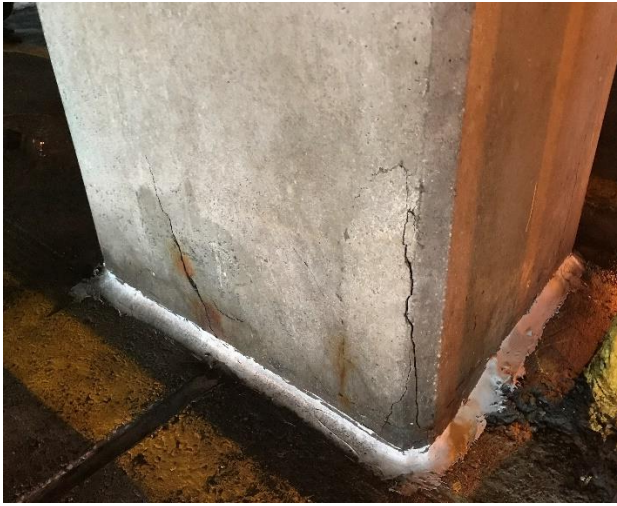
Figure 13. Unsound concrete at column corners.
