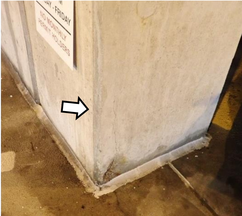
Figure 17. Arrow indicates crack with adjacent unsound concrete near column bottom.
