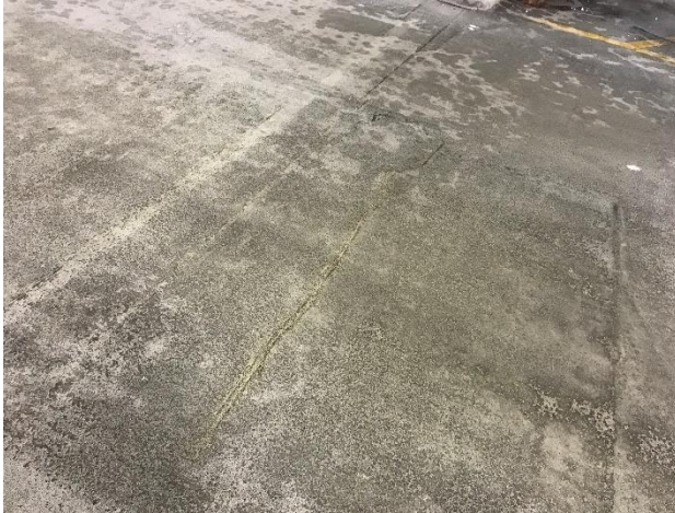
Figure 33. Previously sealed cracks
