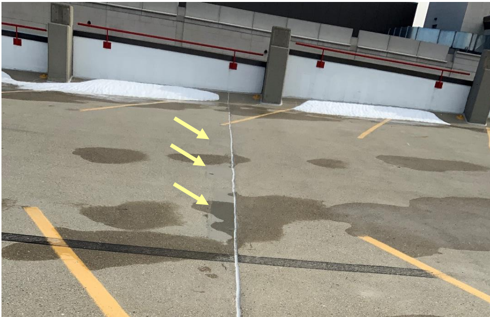
Figure 2. Previous partial-depth concrete repairs at topside of Level 7 construction joint.
