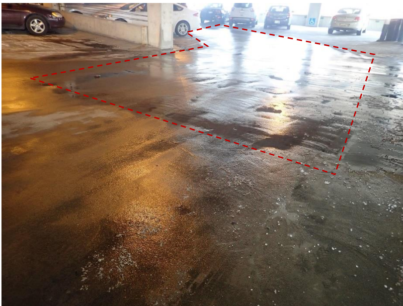
Figure 30. Dashed line indicates standing water observed at Tier 2.
