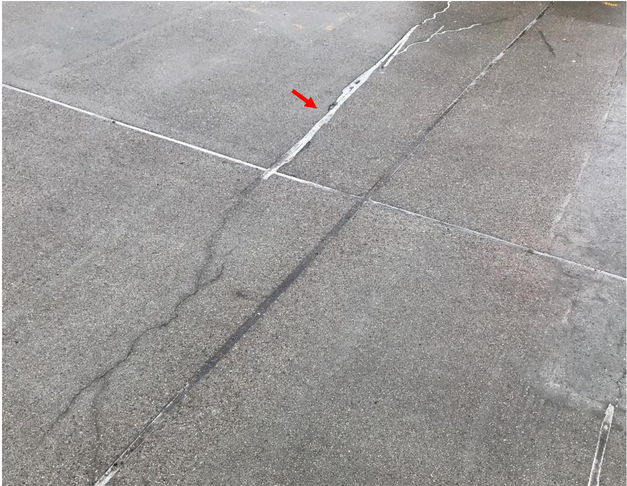
Figure 9. A crack propagating beyond an existing sealed crack. Note a location adhesion failure indicated by the arrow.
