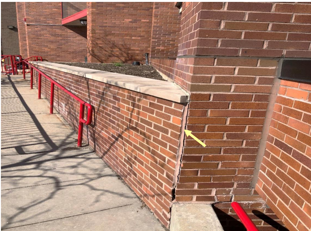
Figure 45. Debonded mortar joint at southwest stairwell entry ramp.
