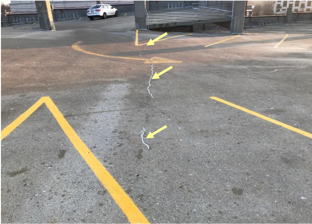
Figure 8. Crack in slab at along beam line.
