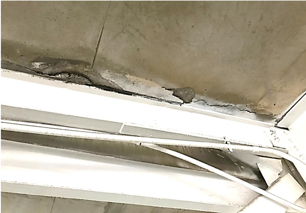
Figure 6. Progressive deterioration at slab edge repair. Note that mild steel and temperature and shrinkage PT anchorages are in this region.
