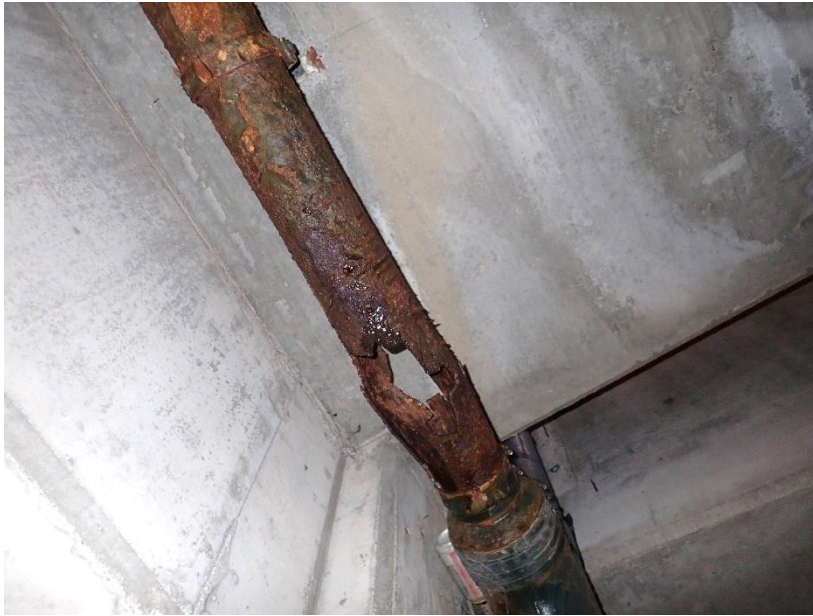
Figure 31. Through-corroded floor drainage pipe.
