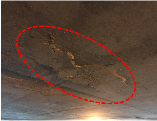
Figure 1. Unsound (delaminated) concrete on a slab underside.
