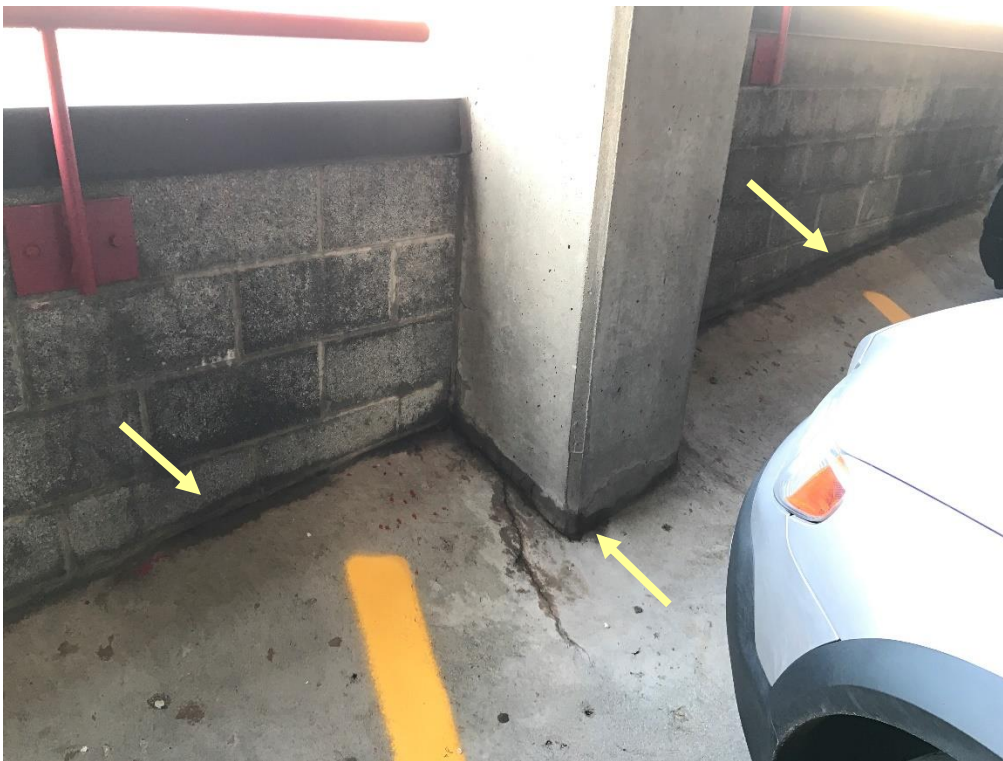
Figure 9. Isolated water staining and cracking in the slab near a perimeter column.
