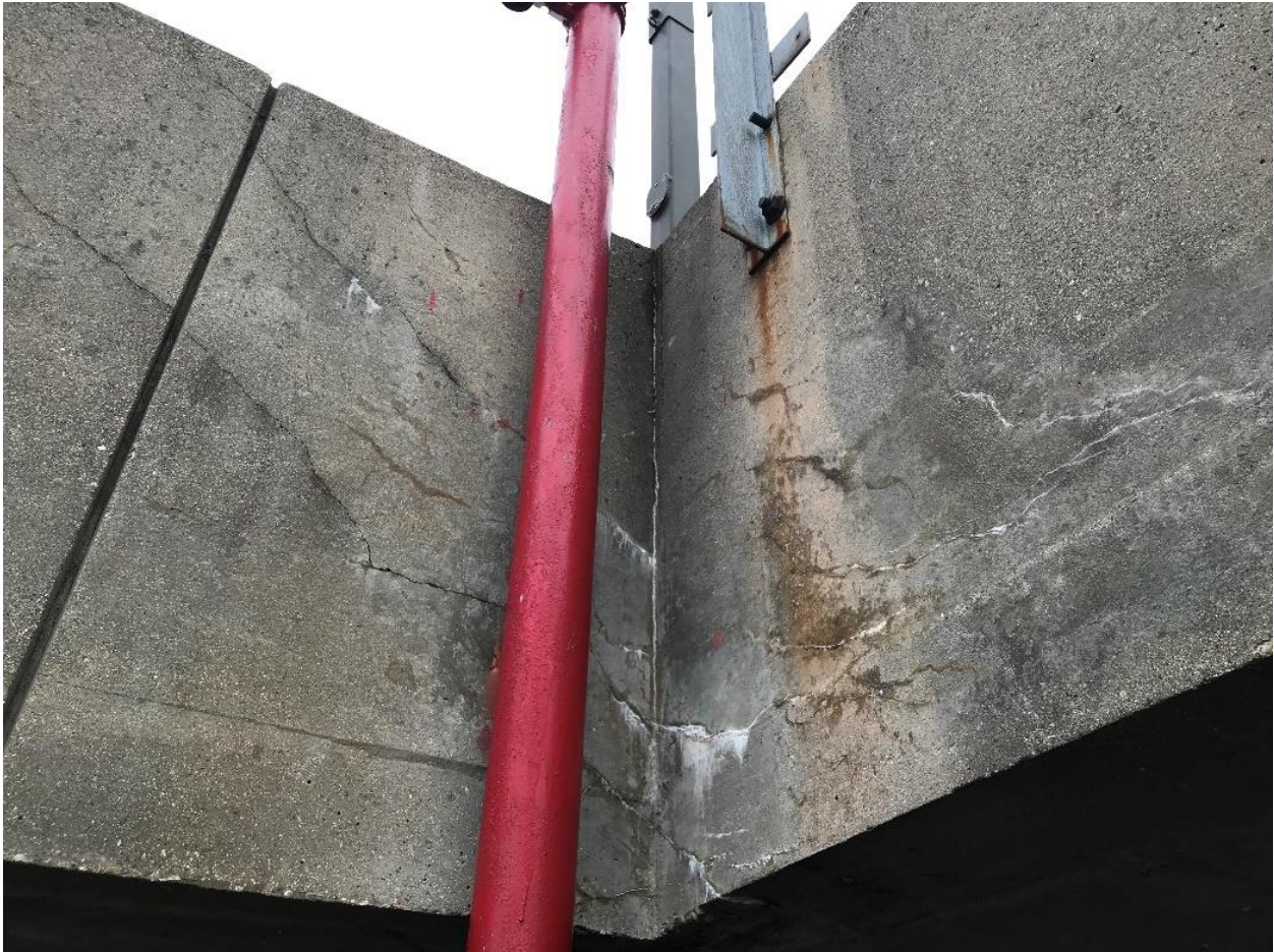
Figure 17. Cracking with efflorescence at the wall corner above the top ramp.
