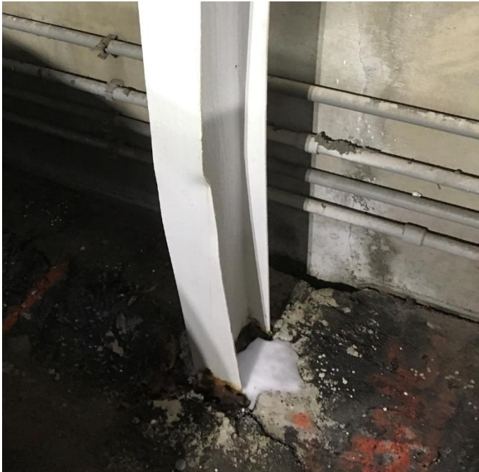
Figure 56. Vehicle impact deformation at intermediate post
