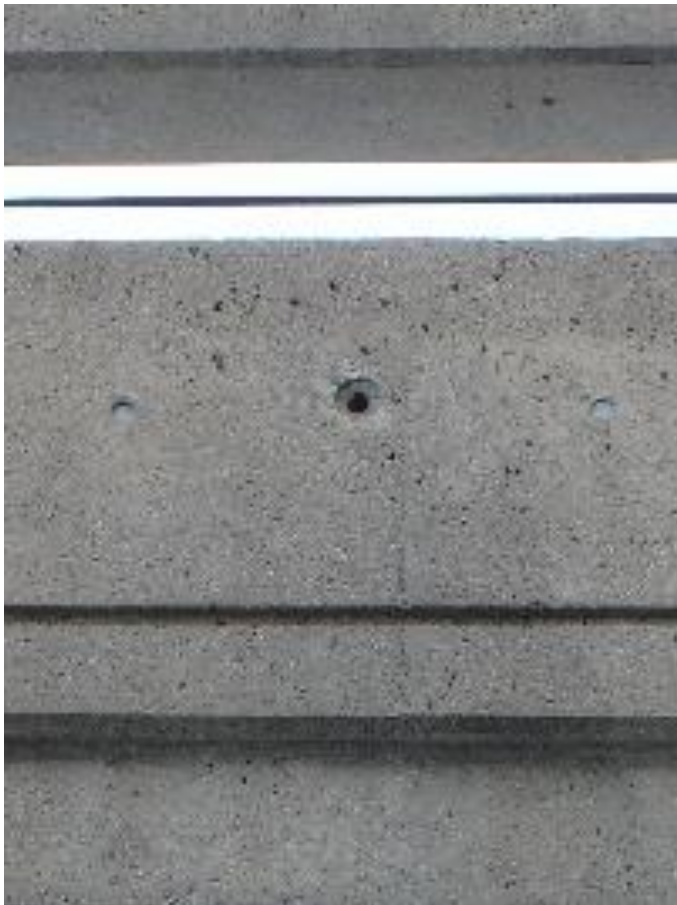
Figure 6. Isolated missing grout from grout pocket for slab PT anchorage.
