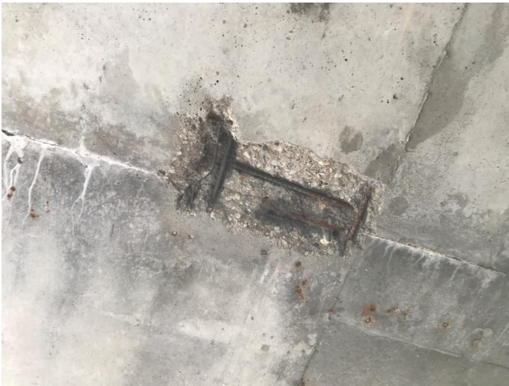
Figure 6. Exposed, corroded mild reinforcement within spall at construction joint. Note efflorescence and water staining along joint.
