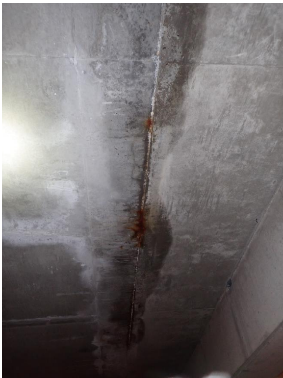
Figure 26. Efflorescence, moisture, and corrosion staining on the underside of a construction joint.
