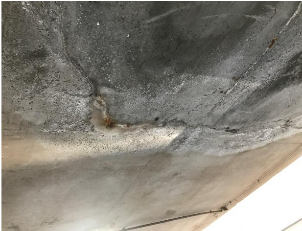
Figure 25. Previous repair exhibiting cracking, efflorescence, and corrosion staining
