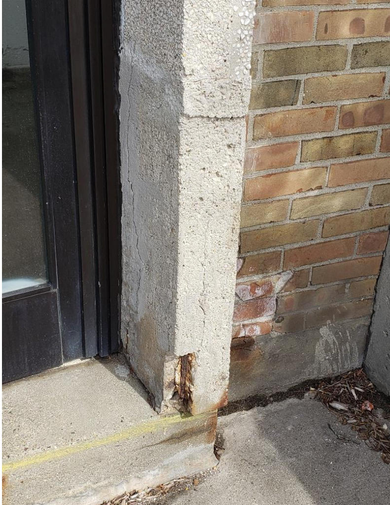
Figure 25. Cracked and spalled concrete panel at entrance door.
