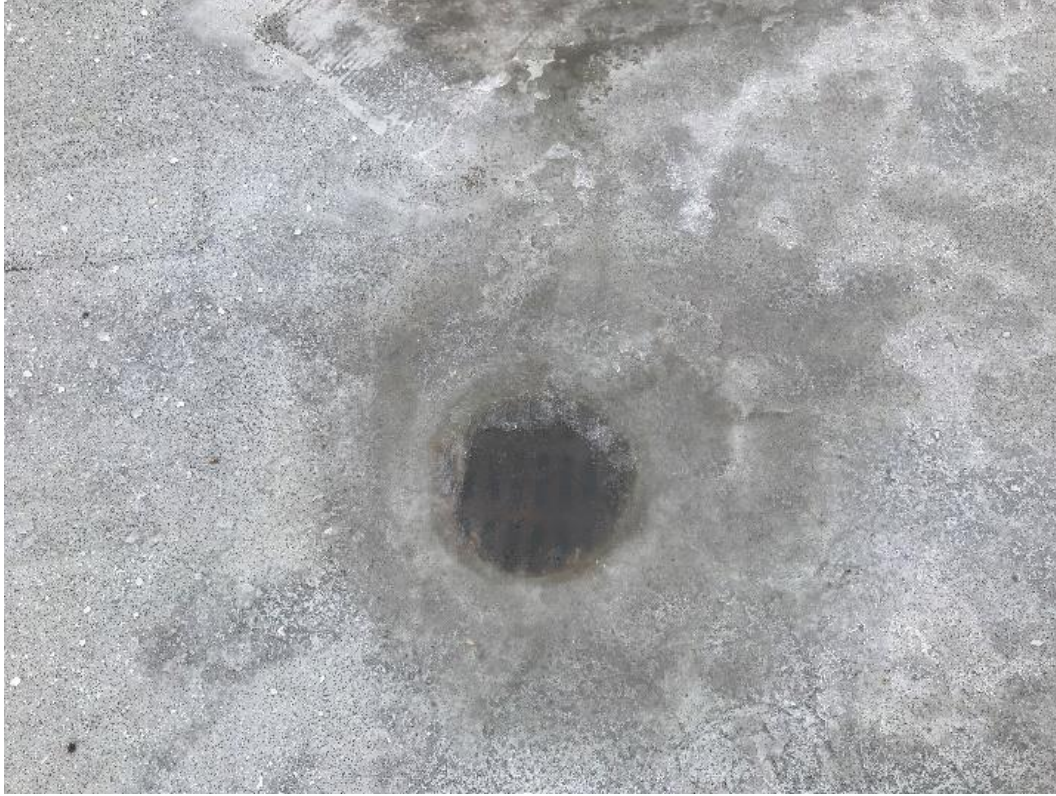
Figure 72. Clogged drain and standing water
