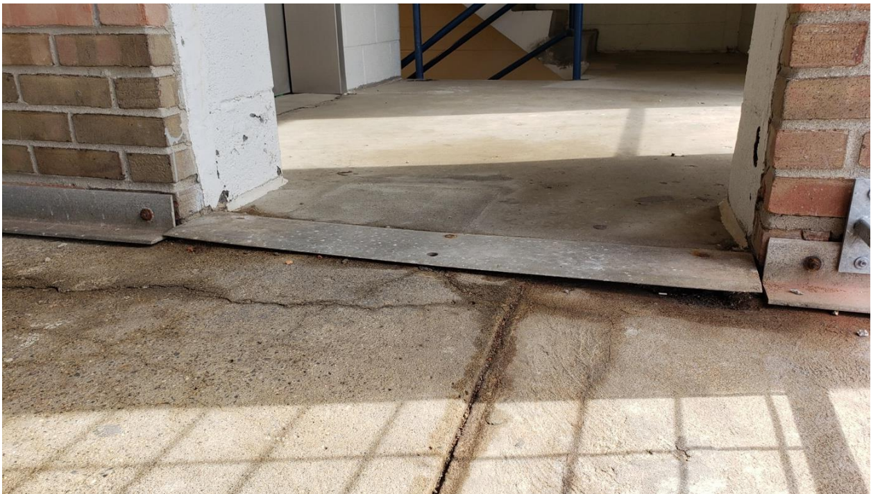
Figure 28. Loose cover plate with gap.
