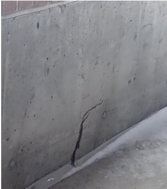
Figure 23. Crack and unsound concrete on perimeter wall, north bay of Tier 1.
