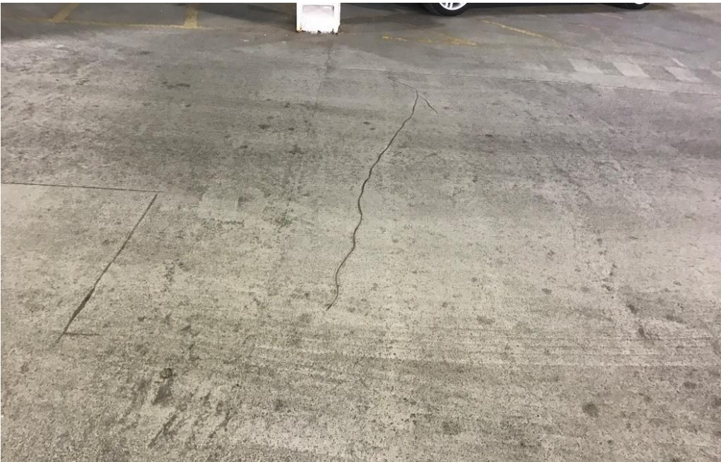
Figure 67. Sealed crack covered by traffic-bearing membrane
