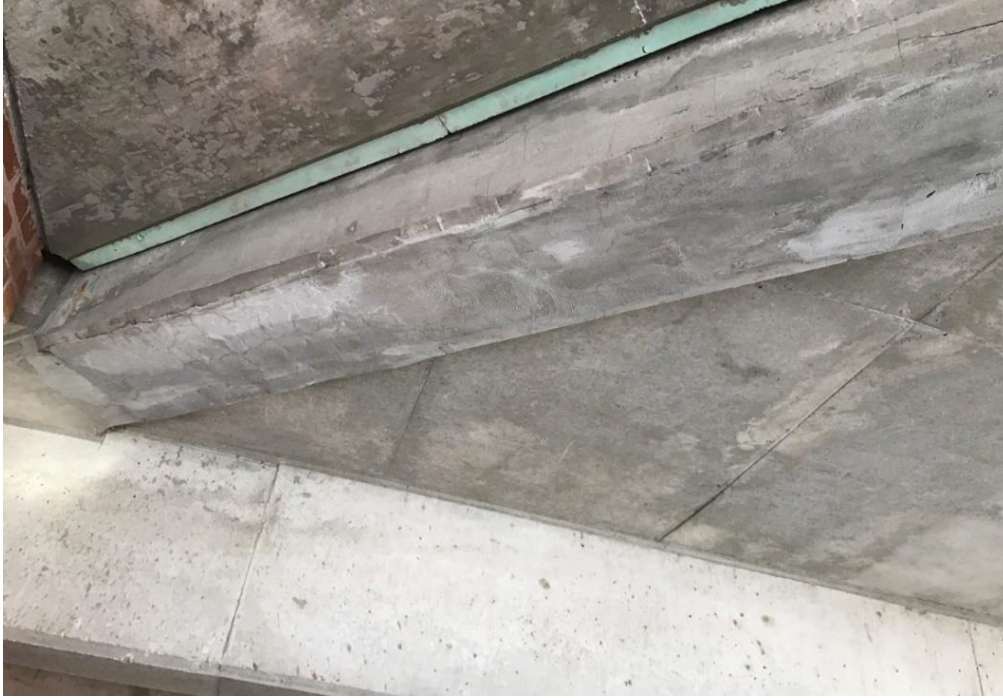
Figure 21. Deterioration at edge beam near southwest stairwell.
