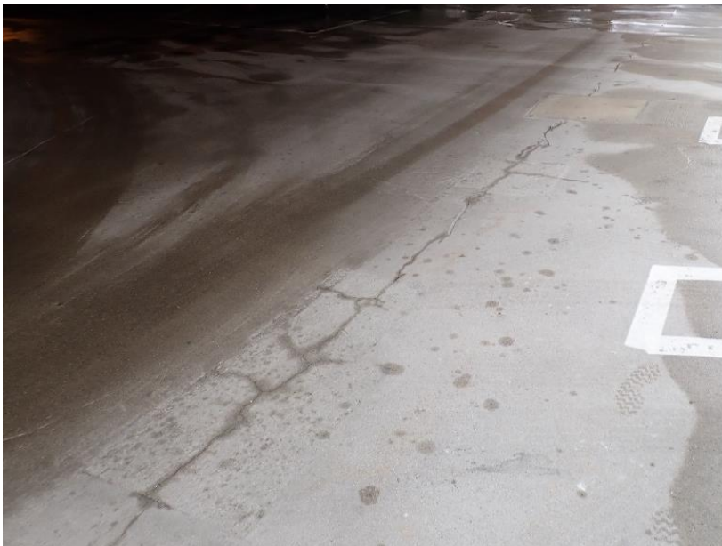
Figure 4. Isolated cracks in line with transverse temperature and shrinkage reinforcing steel, and penetrate previous repair areas.
