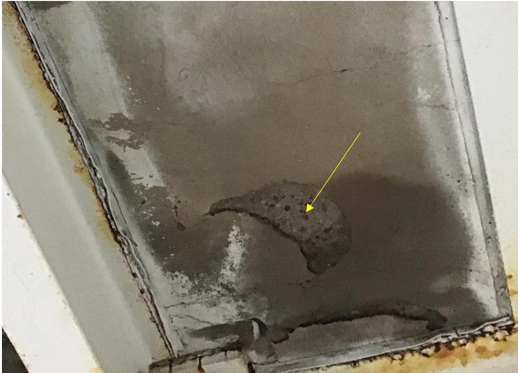
Figure 30. Spall at underside of slab
