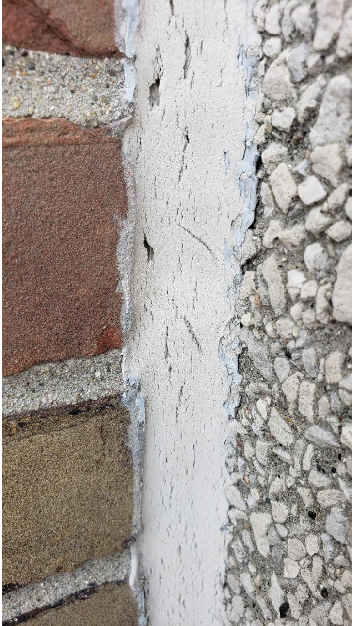
Figure 26. Cohesive and adhesive failure of cove seal.
