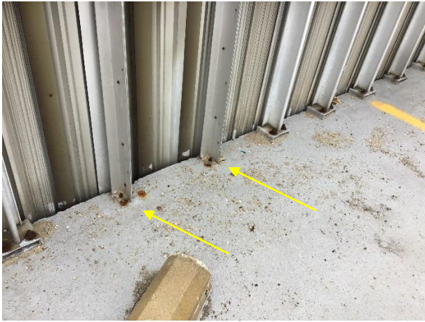
Figure 77. Missing base plates and anchors
