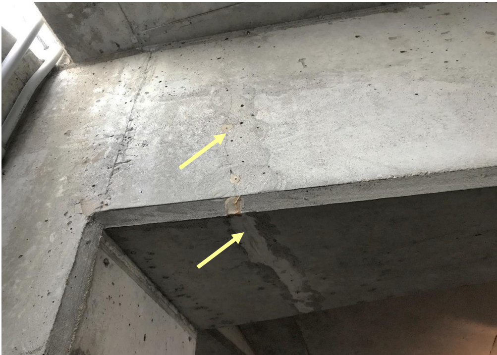
Figure 22. Previous epoxy injection repair at isolated crack at beam end.
