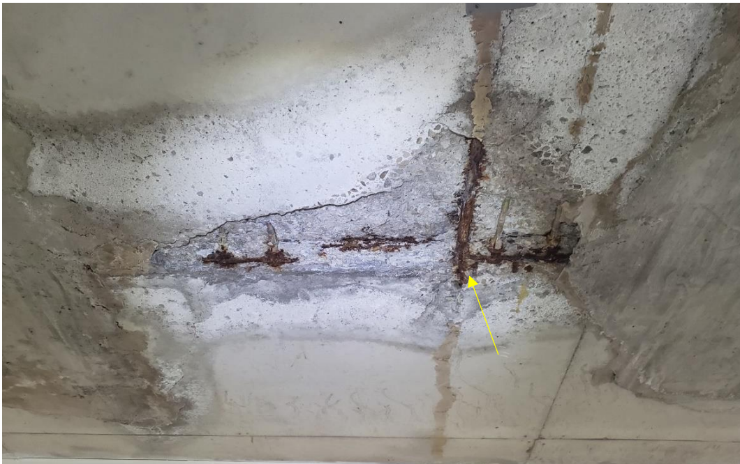
Figure 14. Exposed Tendon Location 4. Conduit indicated by arrow.
