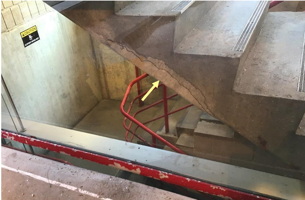
Figure 54. Delamination of previous concrete repair at underside of stair flight.
