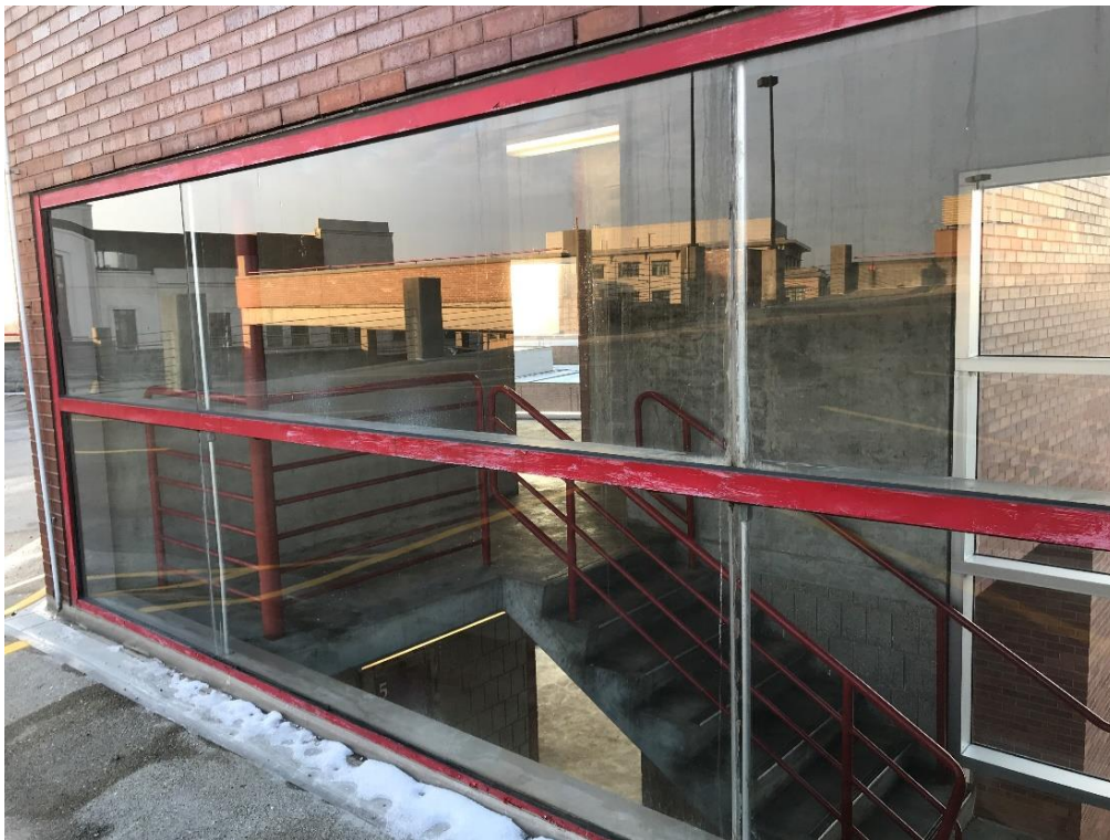
Figure 47. Deteriorated coating, perimeter sealant, and glazing at stairwell storefront.
