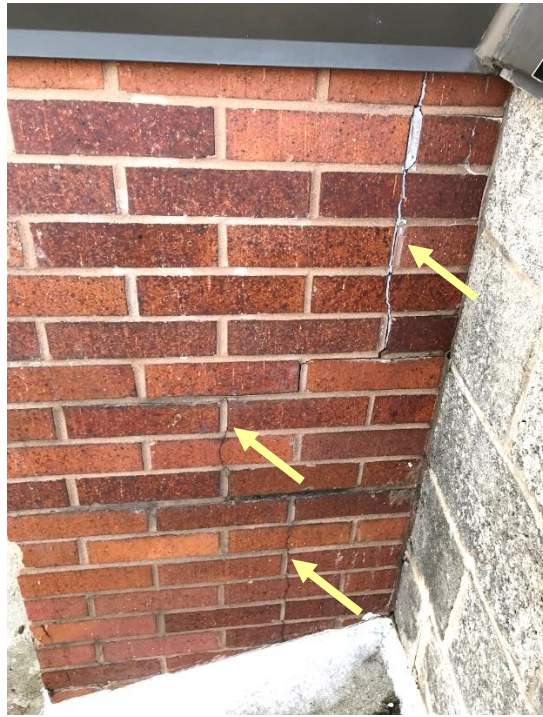
Figure 38. Cracking in brick veneer.
