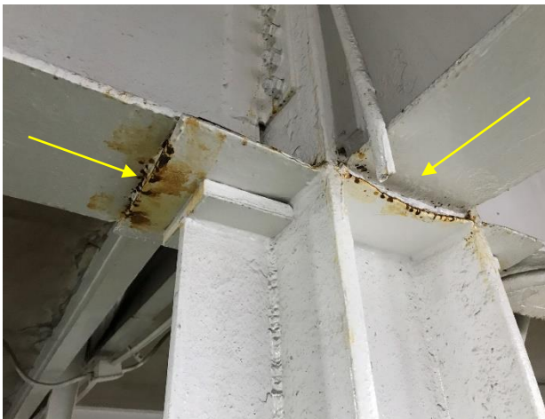
Figure 47. Corrosion byproduct buildup within moment connection
