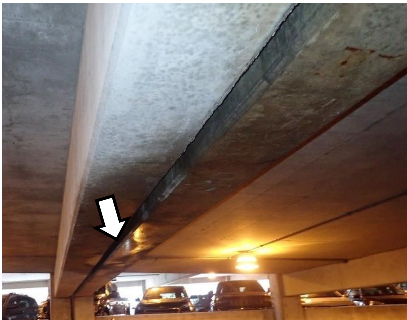
Figure 12. Water infiltration and corrosion staining at the underside of a deteriorated expansion joint.
