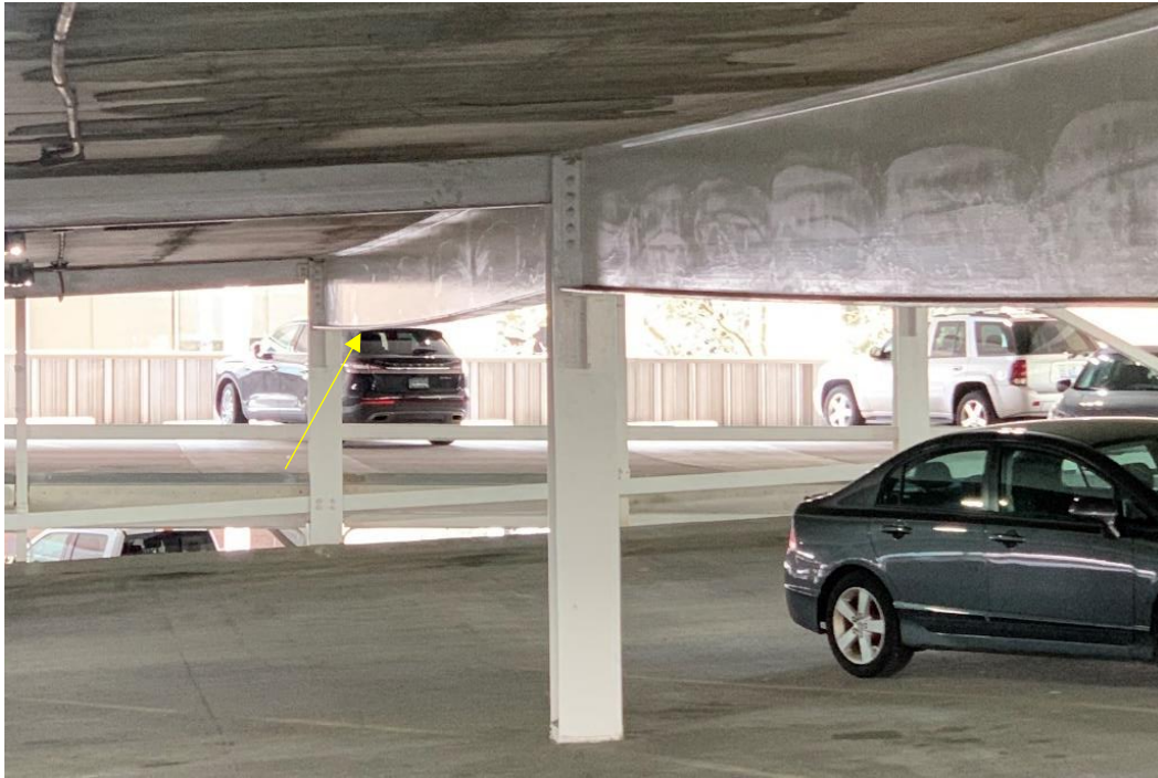
Figure 51. Deflected steel beams
