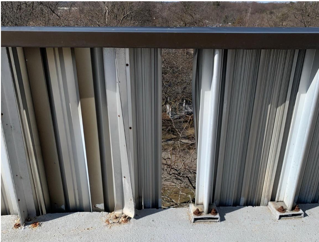
Figure 79. Opening in facade panels at roof level
