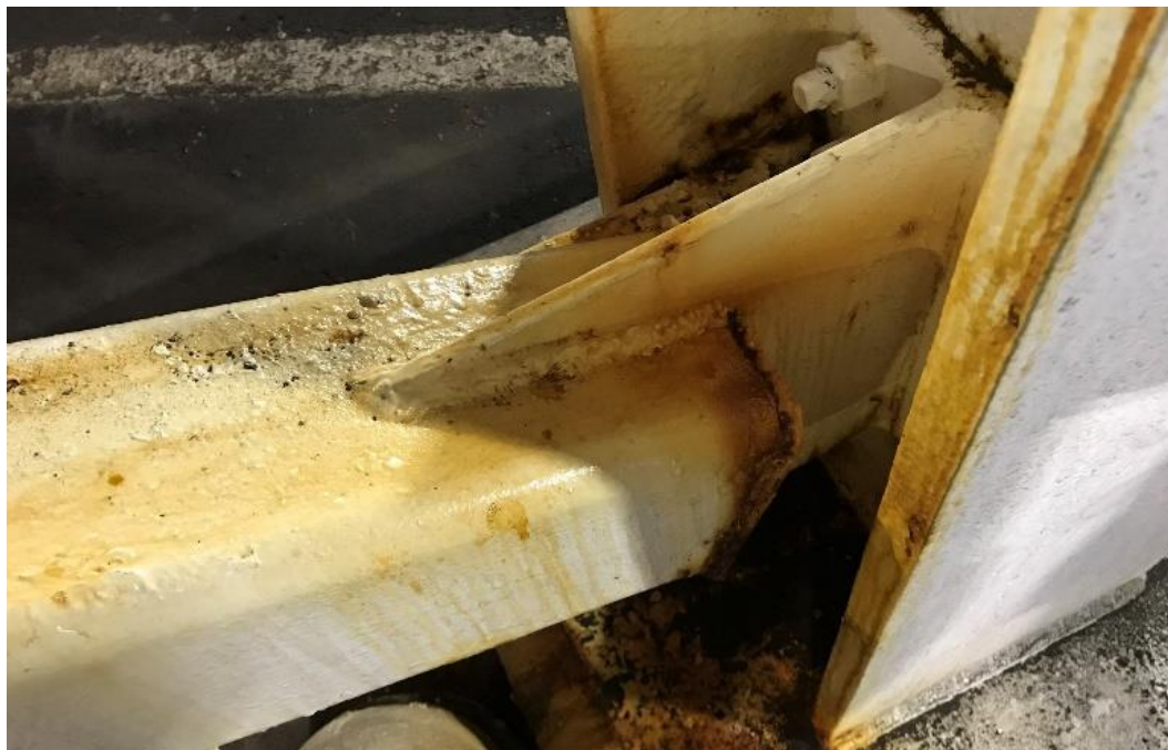
Figure 50. Corroded diagonal bracing connection
