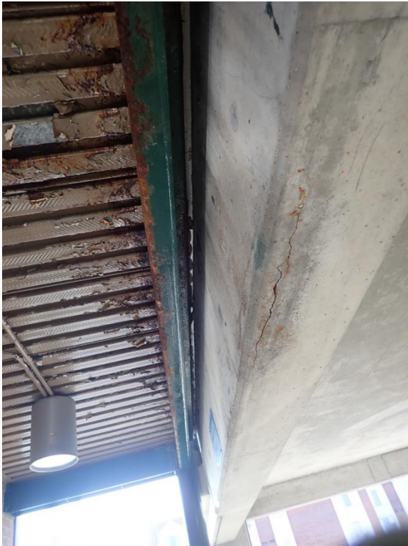
Figure 1. Peeling paint and corroded steel deck on underside of slab at elevator entryway, Tier 2. Note concrete beam distress near region of water penetration.
