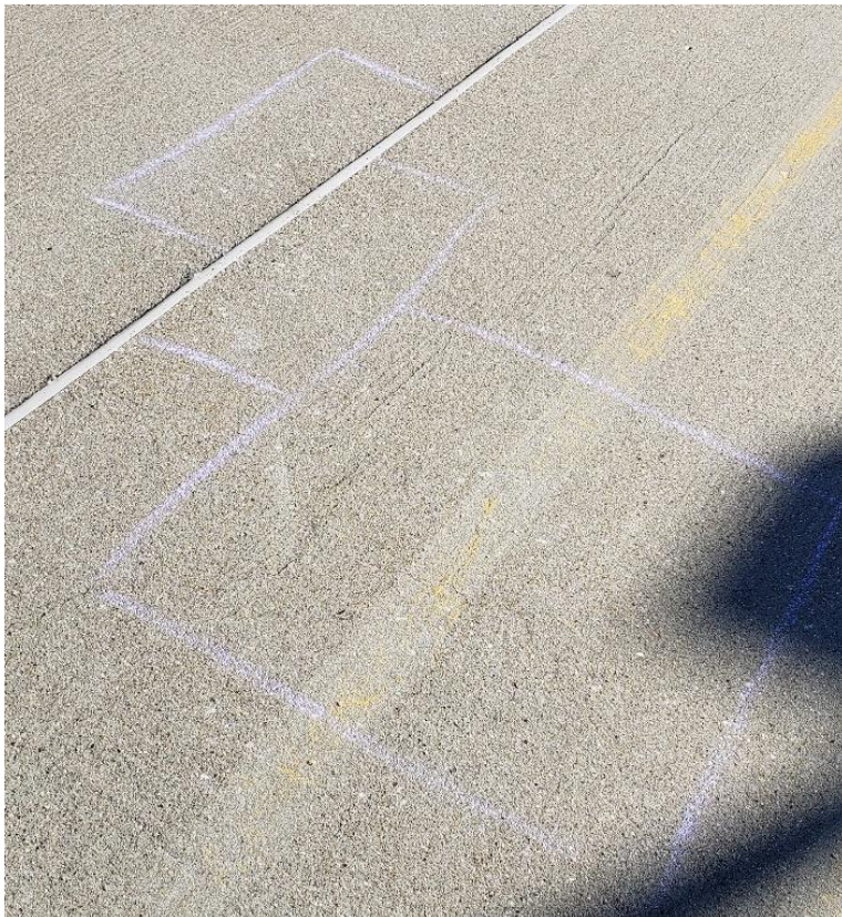
Figure 3. Unsound (delaminated) concrete outlined in chalk. Note that there are no visible indications of concrete deterioration.
