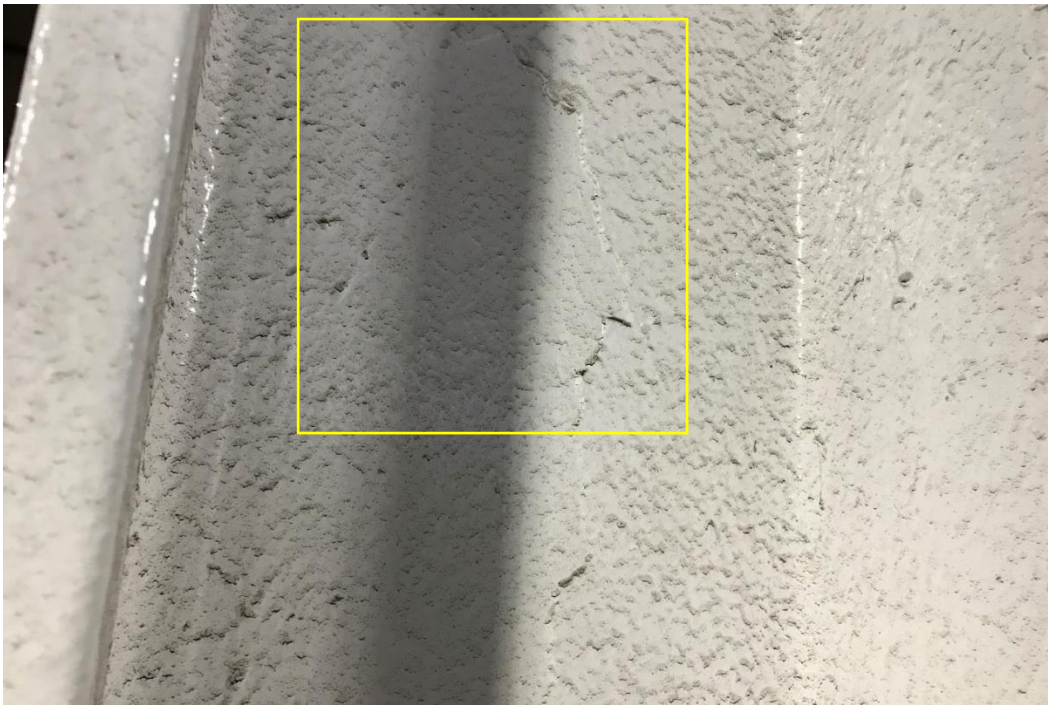
Figure 52. Uneven surface below coating at steel member
