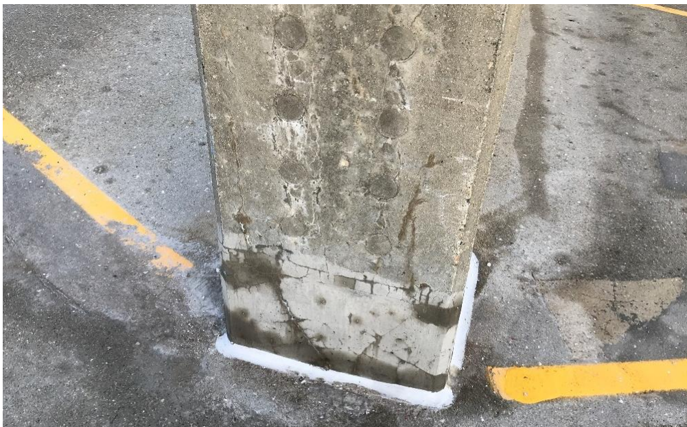
Figure 26. Debonded grout pockets, water staining, and efflorescence within column at vehicle barrier cable anchors. Note unsound concrete patch repair and standing water at base.
