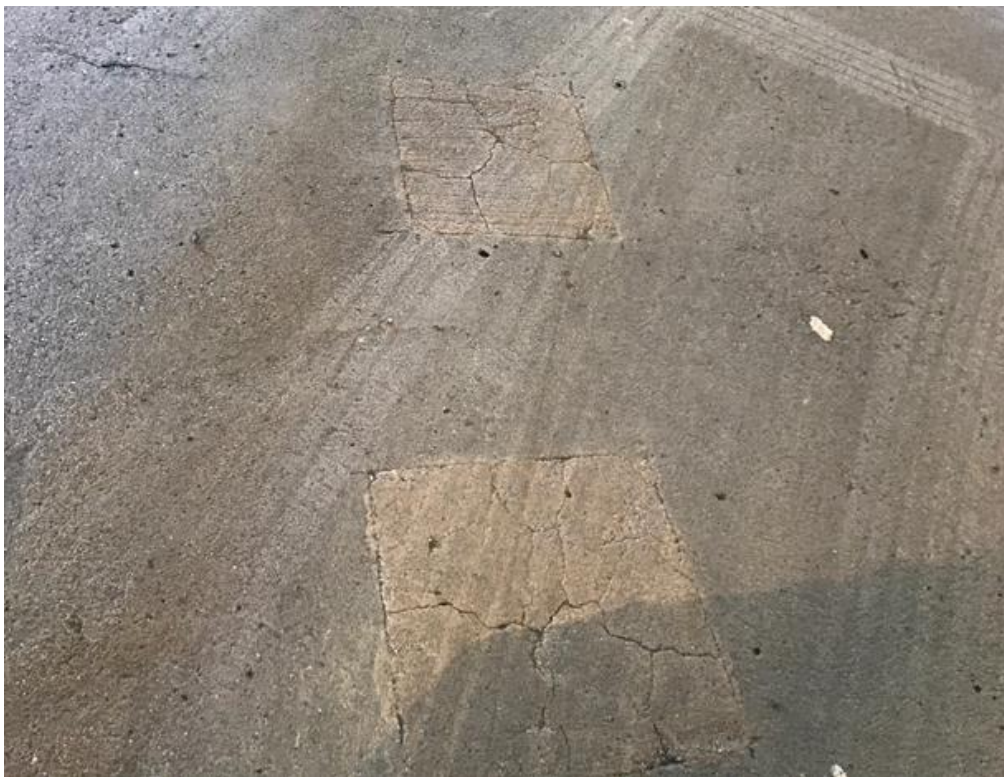
Figure 4. Unsound previous repairs along the top of a beamline.
