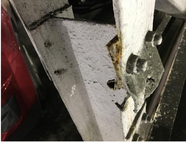
Figure 59. Corroded flange plate at intermediate post splice
