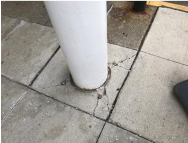
Figure 41. Concrete sidewalk distress at corroded exterior pipe column base
