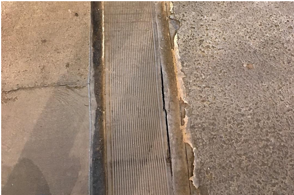
Figure 18. Failed expansion joint seal at the transition between the slab on grade and the elevated PT structural slab.
