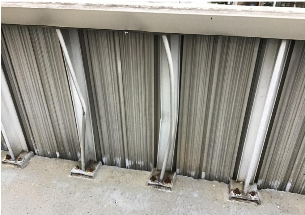
Figure 76. Vehicle impact at facade panel posts
