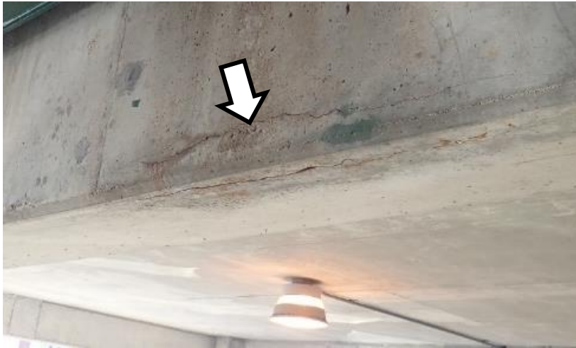
Figure 13. Arrow indicates delamination on beam.
