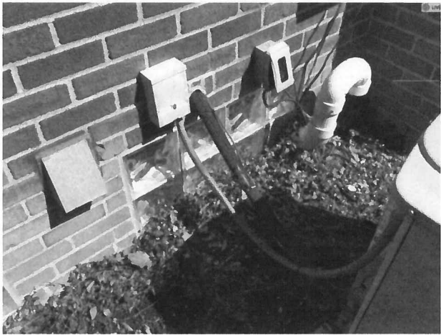
Furnace air intake
