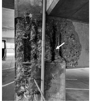
Figure 10. Exposed corroded reinforcing steel and diagonal concrete crack.
