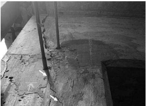
Figure 11. Cracks throughout concrete at Column 11A. Crack propagates through original concrete above as indicated with red arrow. Note the displacement across the crack in the original concrete where the concrete material has spalled.
