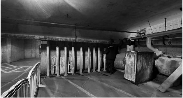
Figure 2. Shoring posts installed at the west end of the Level 1 beam supported by Column 10A.
