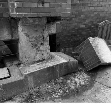
Figure 3. Brick veneer removed from the base of Column 10A. A steel shelf angle supporting the brick veneer indicated with red arrow.
