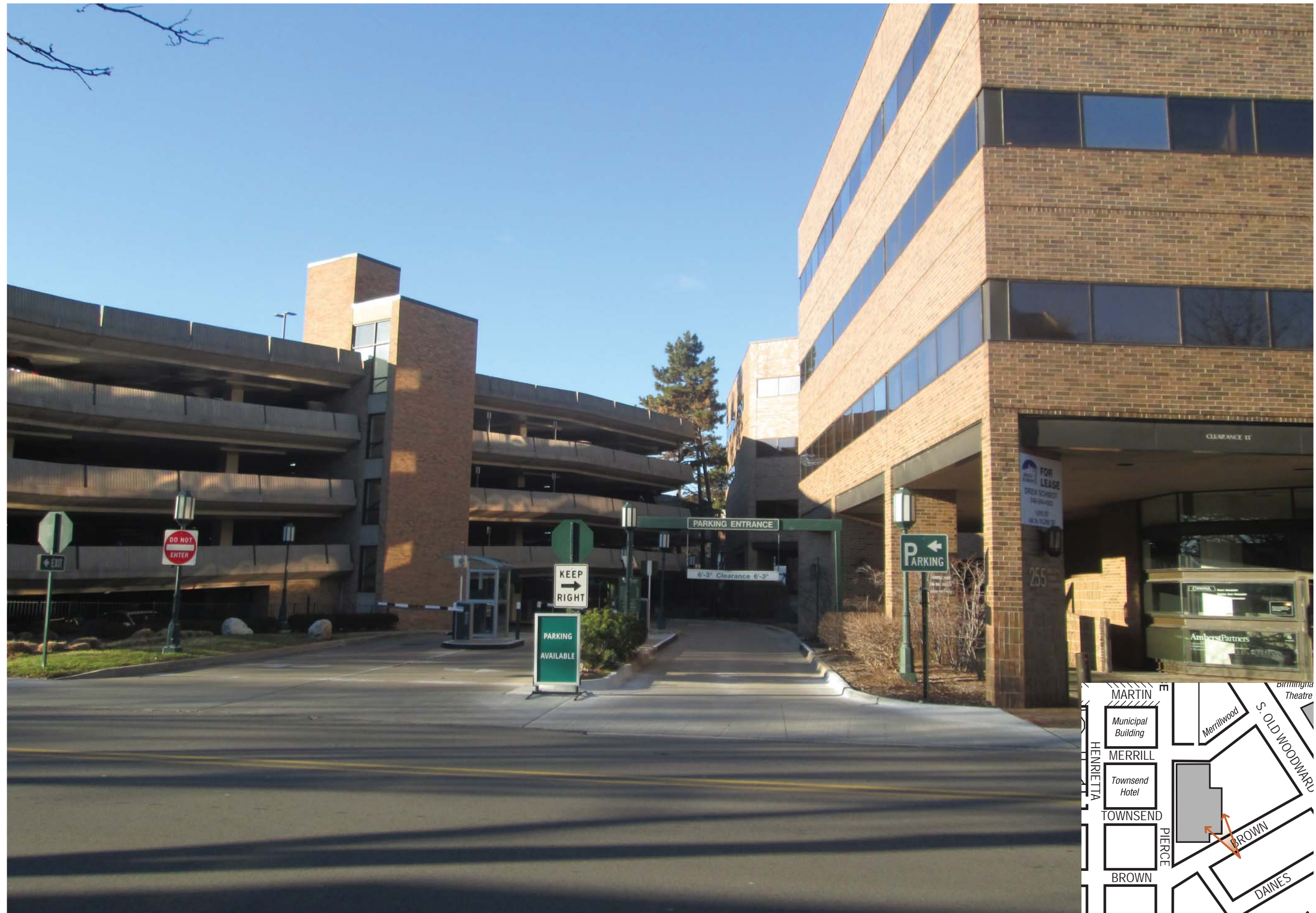
Existing View: South Entry at Brown Street
