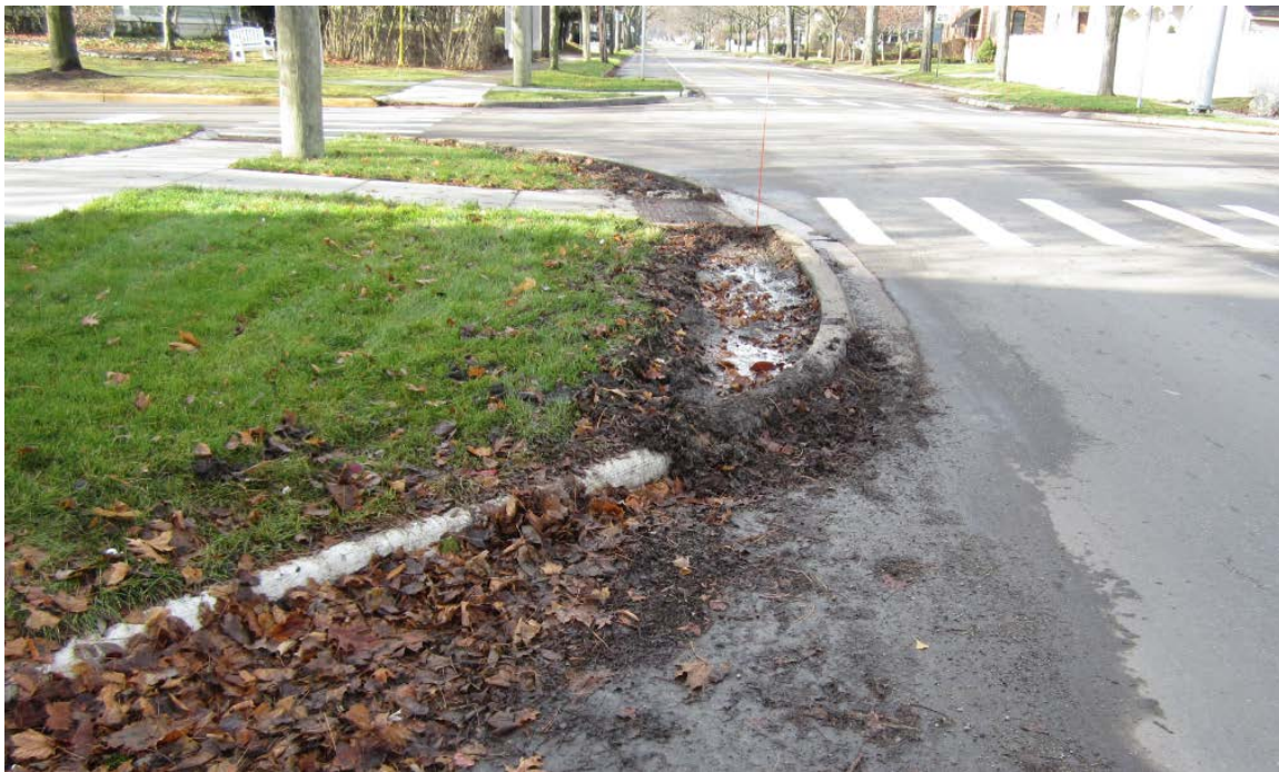
Figure 14 Close up of bump-out. Notice tire tracks have eroded grass and created rut as vehicles have difficulty navigating turns.
