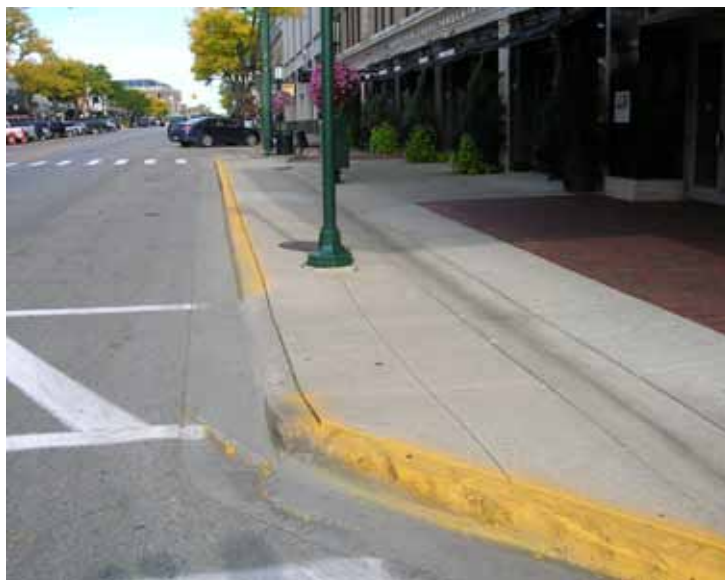
DRAINAGE SWALE IN WALK
