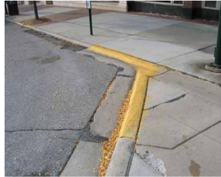
NO POSITIVE DRAINAGE AT INSIDE CORNERS
