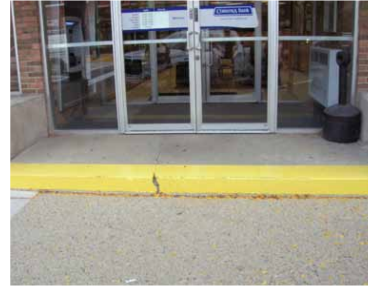
NUMEROUS INACCESSIBLE THRESHOLD CONDITIONS
