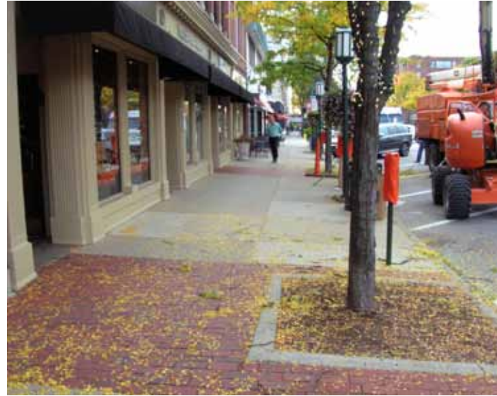
FLUSH TREE PLANTERS ALLOW FOR DE-ICING SALTS TO INUNDATE
