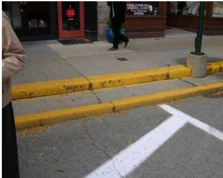
DOUBLE CURBS TO BE CORRECTED WITH NEW STREET DESIGN
