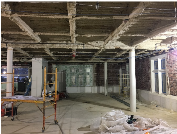
Brick restored to the original color
