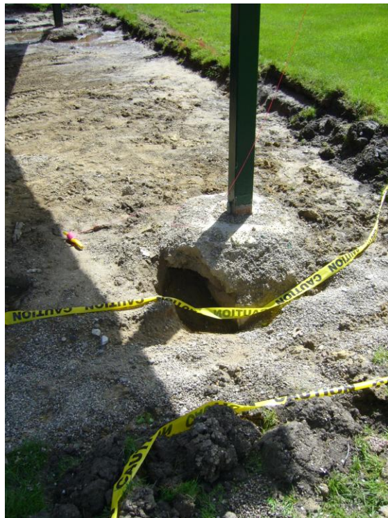
Springdale Pavilion – Typical Column Foundation
