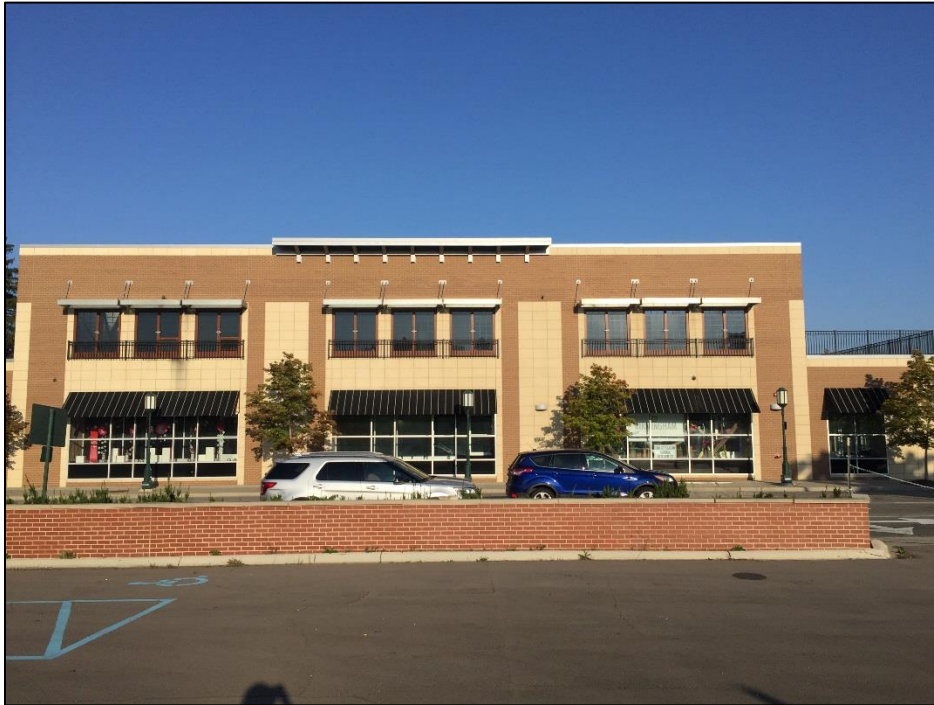
PHOTO NO. 3: View of the north-adjointing commercial retail building and Mobil 1.
