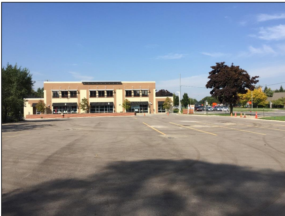
PHOTO NO. 2: View of the north portion of the site.
