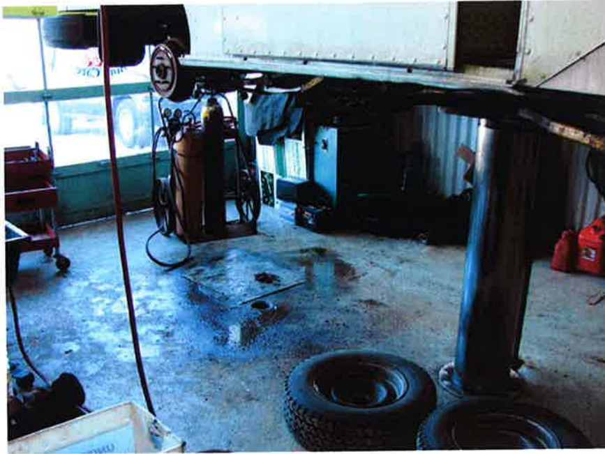
PHOTO NO. 13: Surface staining near an open floor drain and hydraulic hoist within the Property building.
