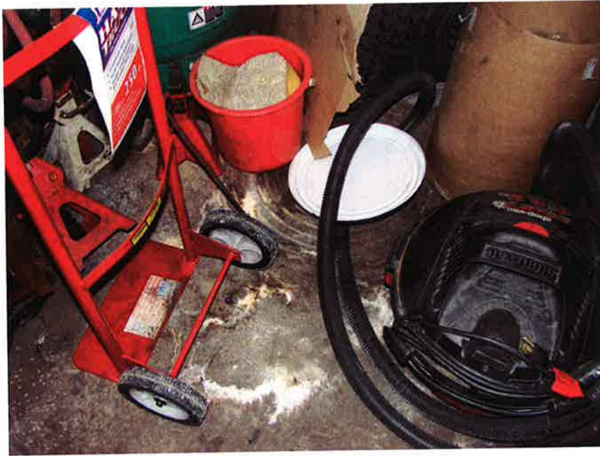
PHOTO NO. 15: Chemical residue on the concrete floor surface near a manhole, located within the Property building.
