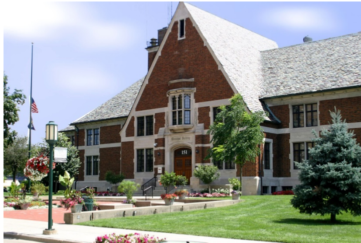
Municipal Building, 151 Martin, Birmingham, MI 48009
