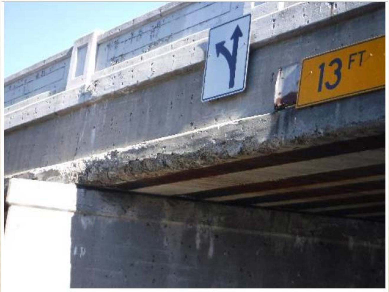
Concrete Deterioration- Slab Wall
