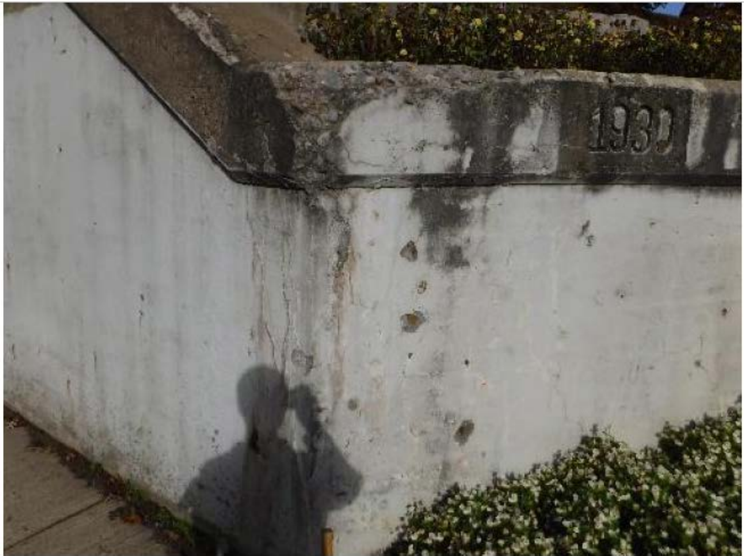
Concrete Deterioration- Bridge Retaining Wall
