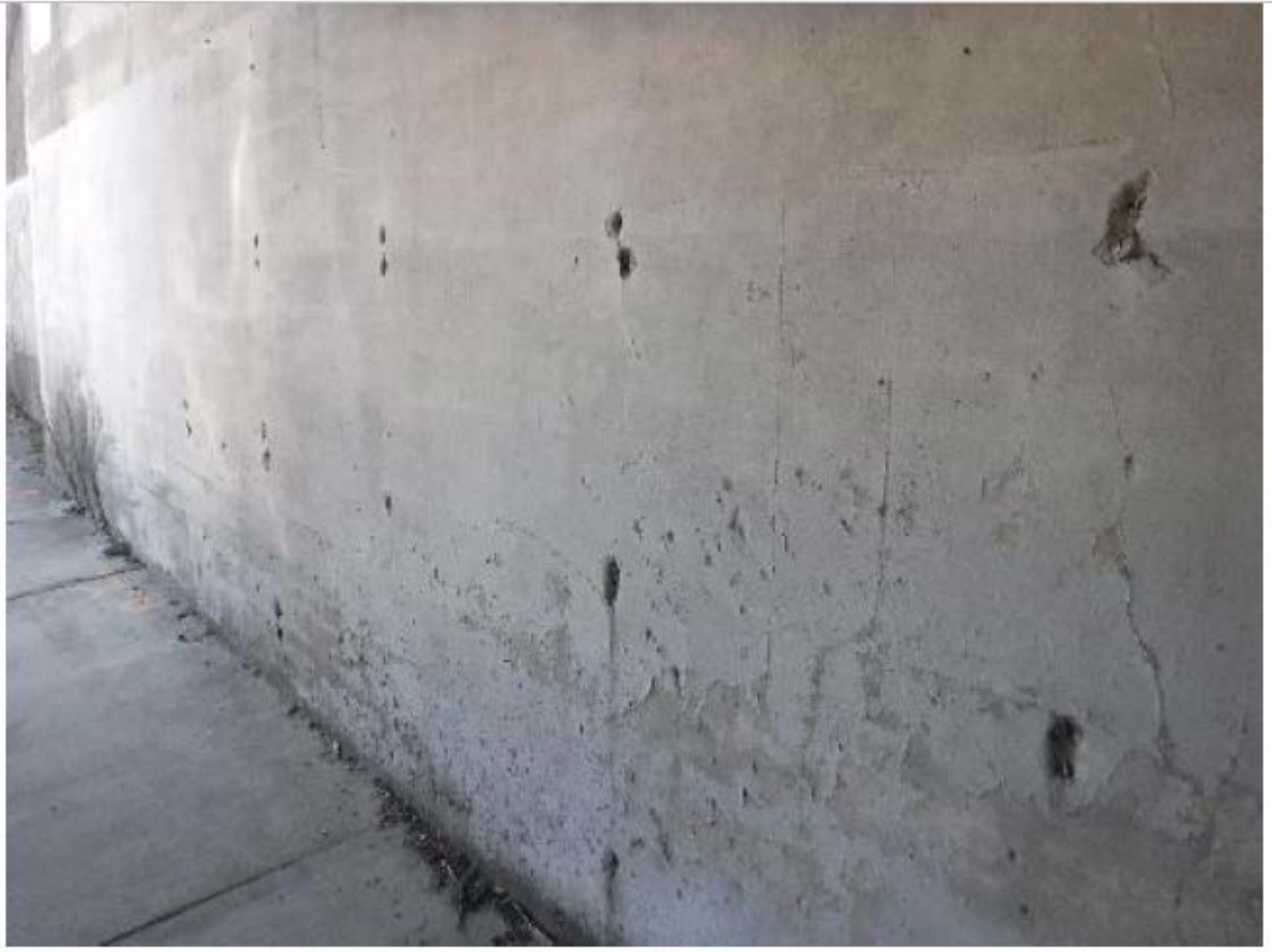
Frequent concrete spalling/rust staining at shallow steel
