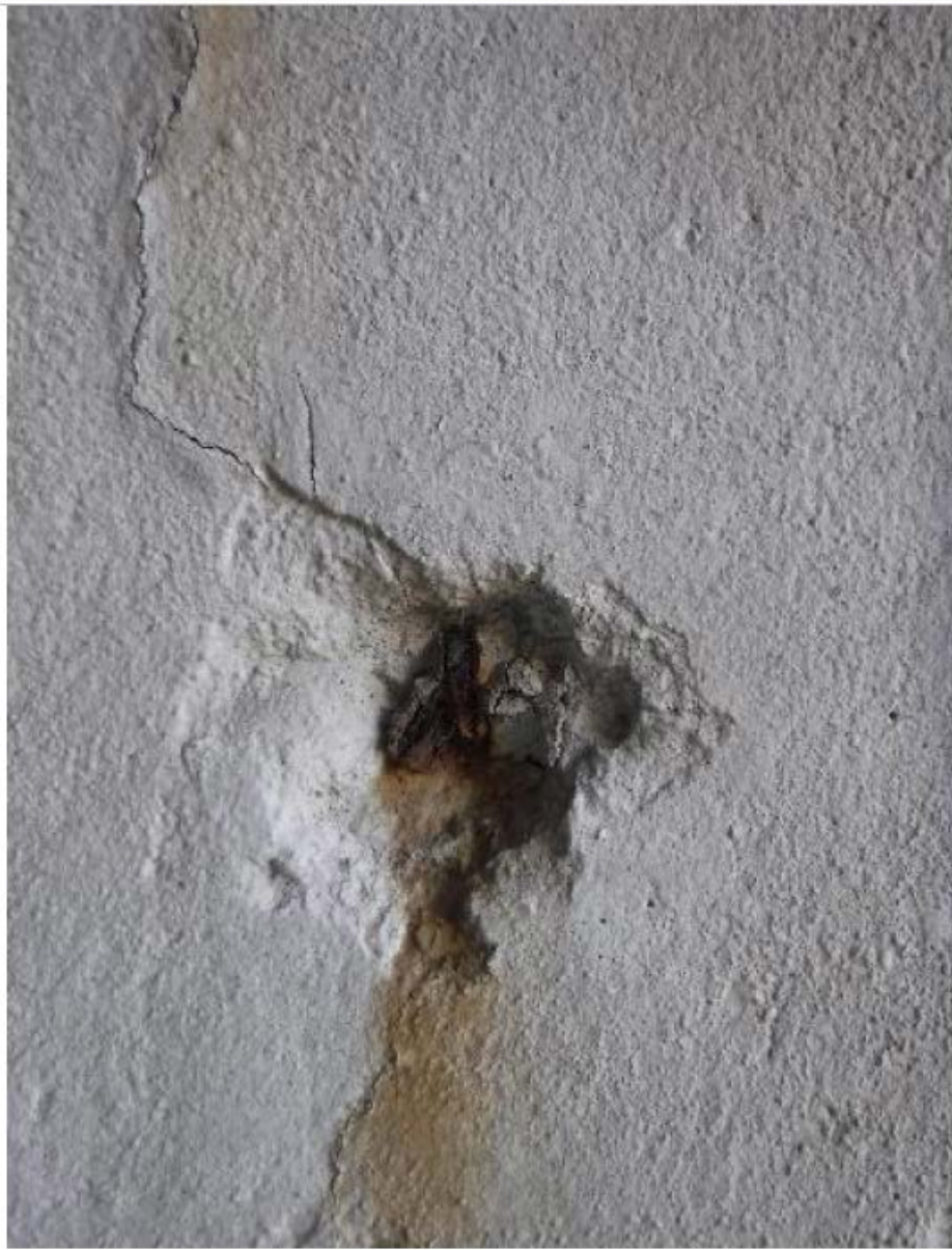
Close Up of Spalling/Rust Staining
