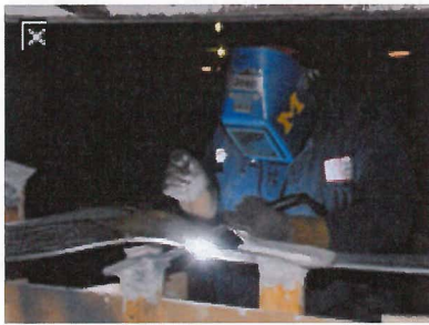
Welding sections on both sides.
