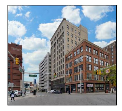
Colasanti is currently acting as construction manager for the Clark Lofts project. 35 W. Grand River is a 10-story 40,000 square foot building. Our scope of work for this project consists renovation of the apartment units located on floors 3-10 which will include demolition, new interior framing and finishes, existing window replacement, upgrade to all MEP systems, roofing, hazardous material abatement and exterior façade restoration
