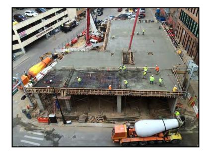
Colasanti Specialty Services was selected as the concrete contractor for the new 28 West Grand River Micro Loft project located in downtown Detroit. Colasanti formed, placed and finished all of the cast-in-place concrete for the 218 unit thirteen story loft apartment project.
