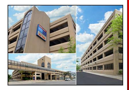
Colasanti was selected as the construction manager for the 1,200 car Lothrop Street Parking Structure renovation project located in downtown Detroit. Our scope includes cast in place concrete deck restoration, new security cameras, blue light phone system and card access, new light fixtures, new parking control equipment, new elevator's, new plumbing and heating and cooling units, replaced overhead doors and new way finding signage, paint and new IT network for the structure.
