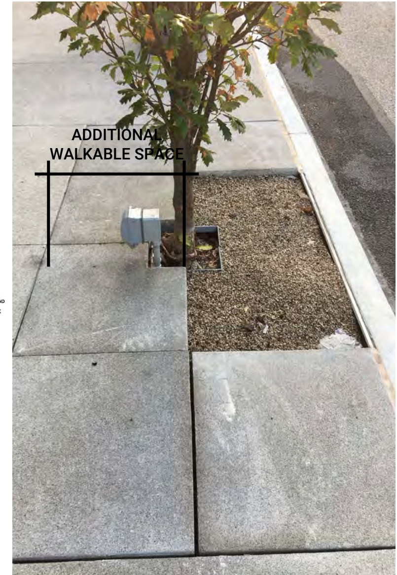
Proposed tree grate detail (above) and constructed tree grate (right)
