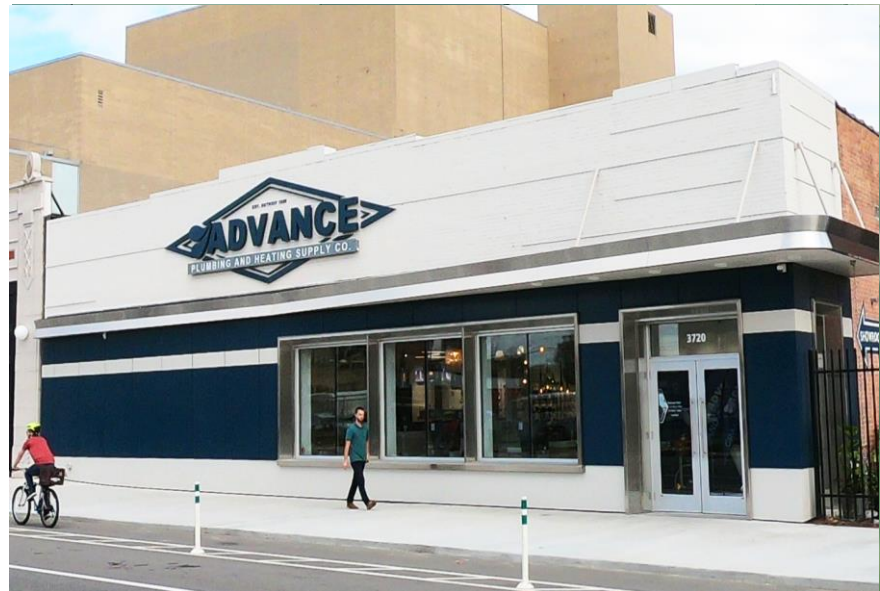
Painted Cement Fiber Board Rainscreen/Siding
