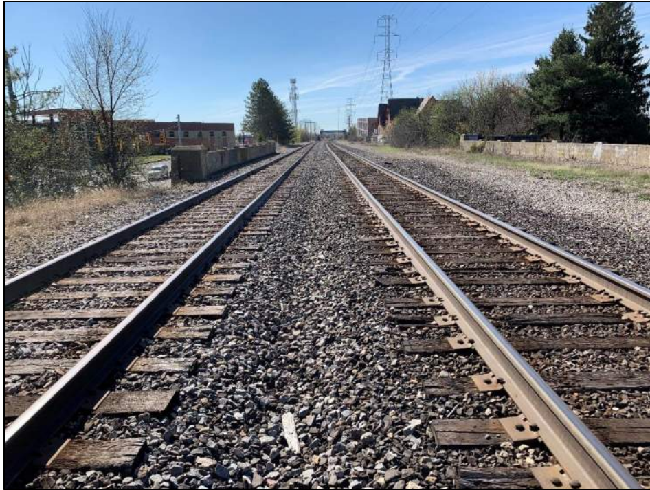
Shallow swale in ballast between tracks, looking south
