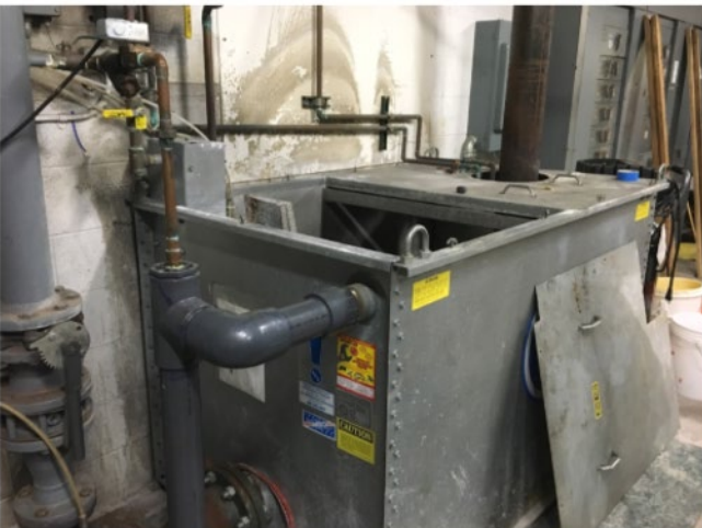
Cooling tower holding tank
