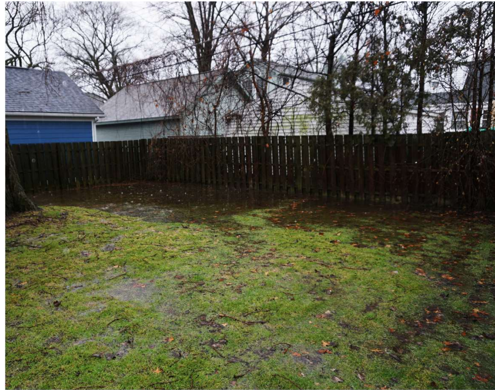
1680 S. Bates routinely floods
