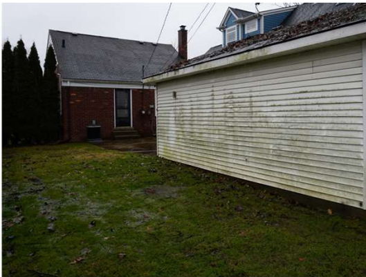
The garage is covered with mold.
