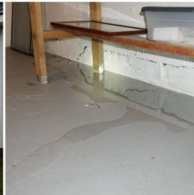
There are large cracks in the foundation and extensive leaking in the basement.
