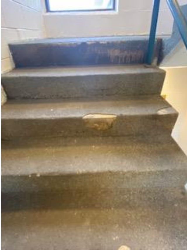
Pierce Stair Tread and Riser Repairs
