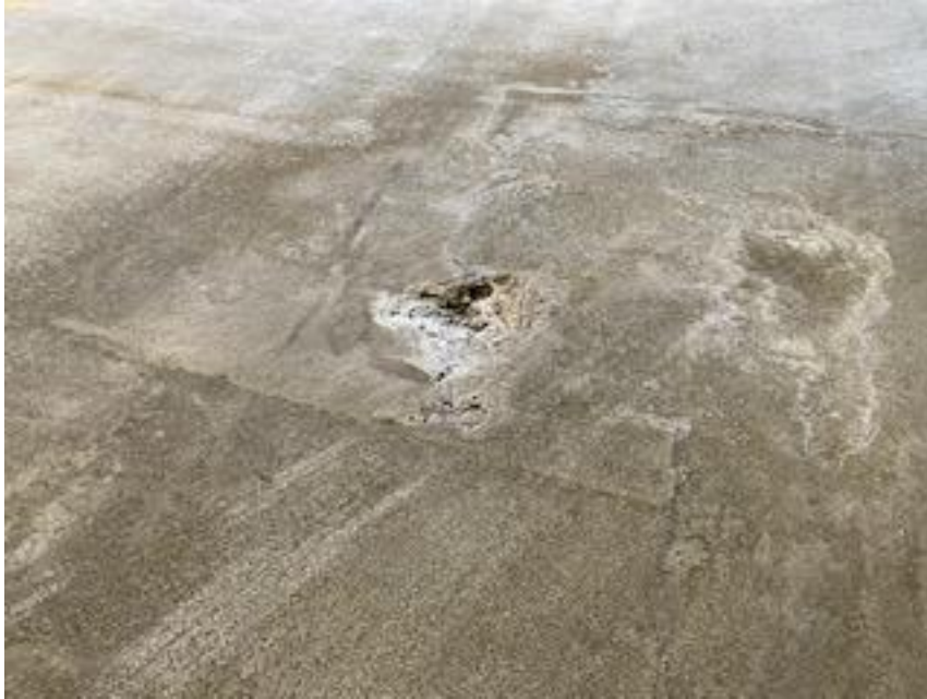
Floor Delamination's
