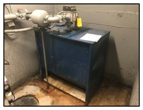
VIEW OF ELEVATOR HYDRAULIC EQUIPMENT AND SUMP PUMP (LOWER LEFT) IN SOUTHWEST TOWER OF SUBJECT BUILDING
