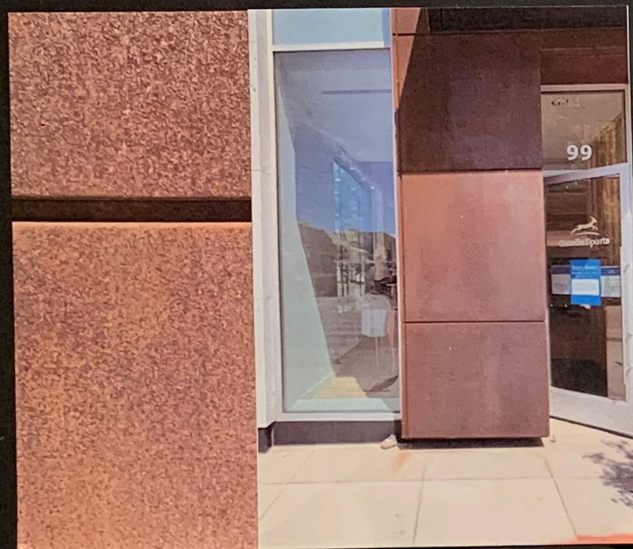
SEALED RUSTED STEEL VERTICAL SHAFT ENCLOSURE
