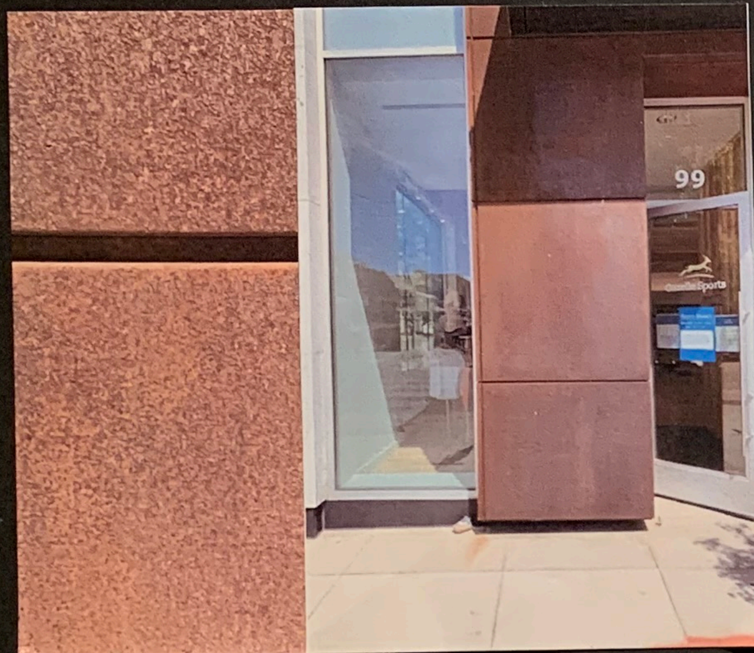
SEALED RUSTED STEEL VERTICAL SHAFT ENCLOSURE
