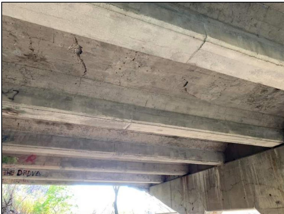
Deck delamination in east span
