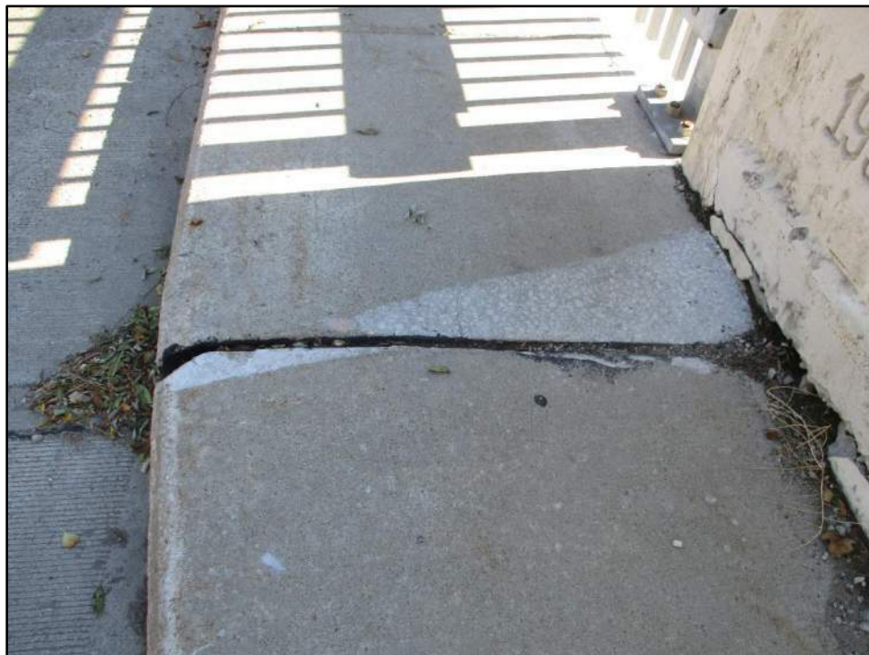
Sidewalk deterioration at abutment
