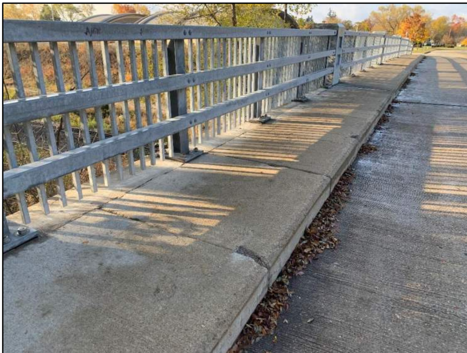
Spalling of south sidewalk
