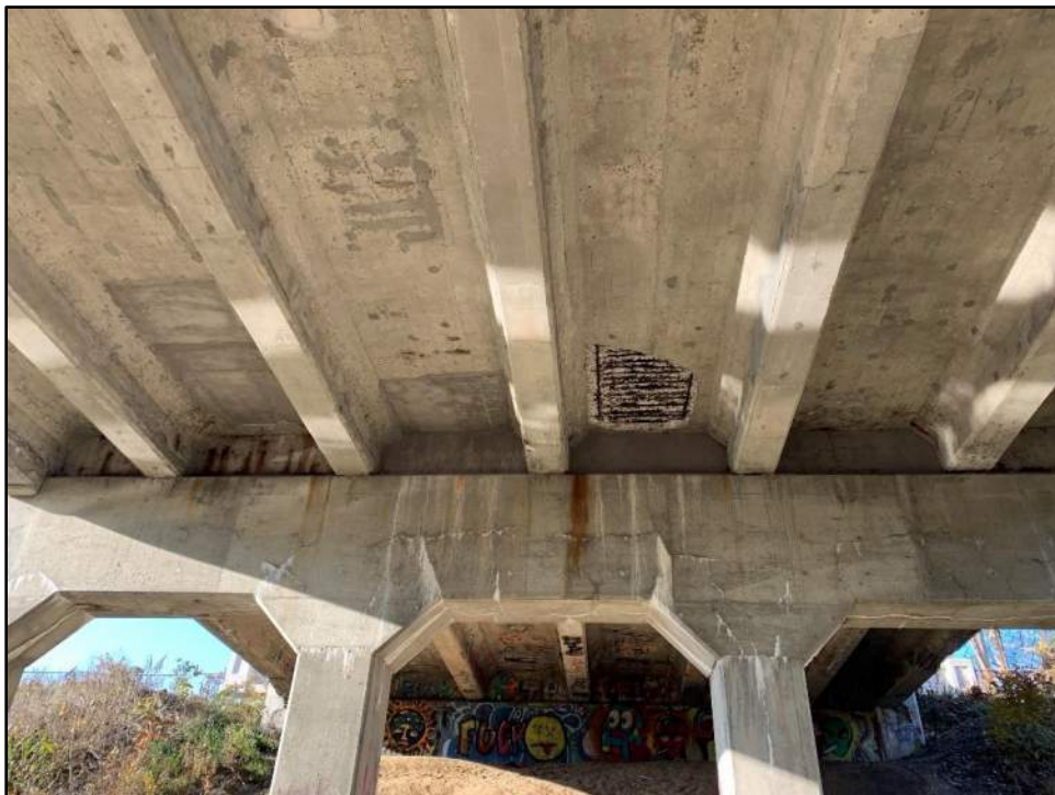
Deck spalls with exposed rebar and pier cracks in west center span
