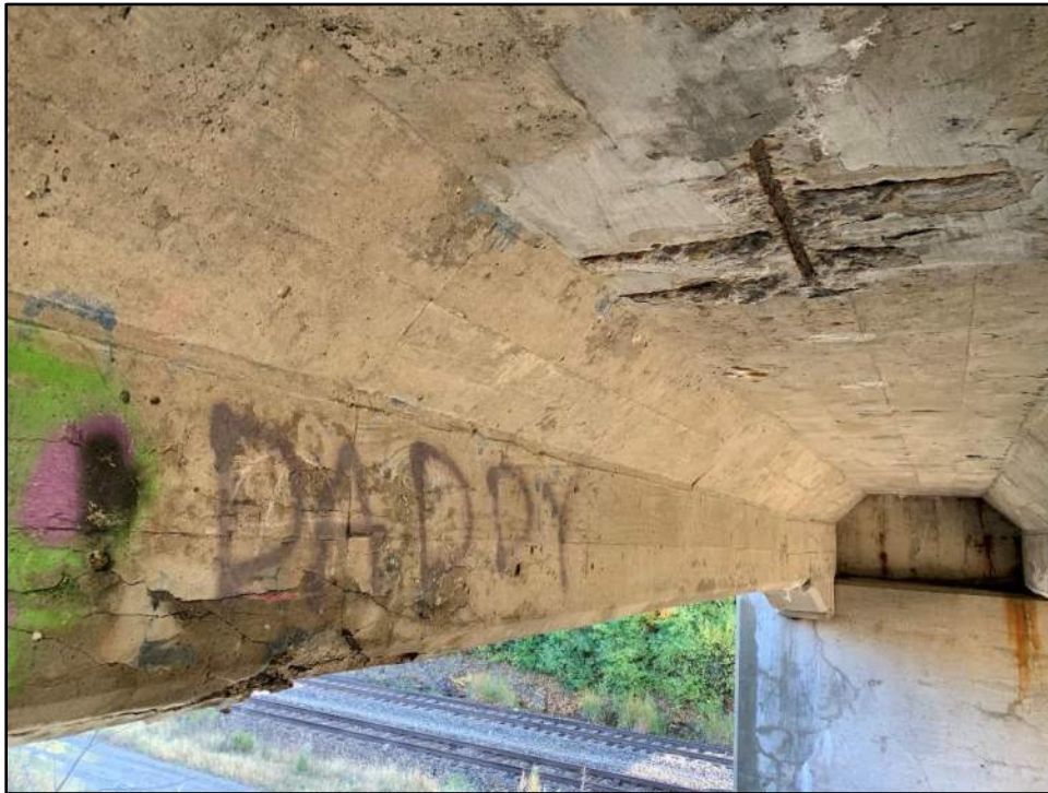
Deck spalls with exposed rebar, beam cracks and diaphragm deterioration in west span
