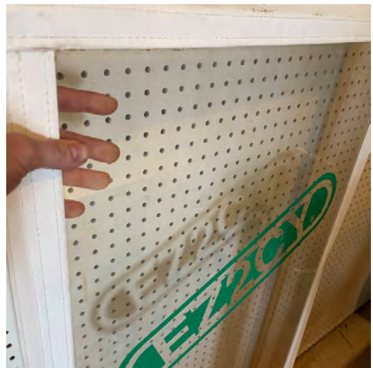
CLEAR VINYL SHEET (EZ2CY) IN CANVAS BORDER ATTACHED TO METAL FRAME
