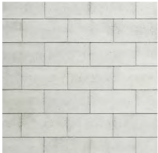
WHITE PAINTED CONCRETE MASONRY UNITS, ON ALLEY ELEVATION
