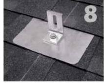
washer. Using a 1/4-inch socket on an impact gun, Follow all the directions of the rack manufacturer drive prepared lag bolt through L-foot until L-foot as well as the module manufacturer. NOTE: Make sure top of L-Foot makes solid contact with racking
