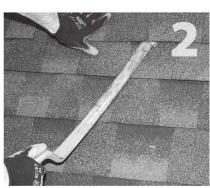
Carefully lift composition roof shingle with roofing Insert flashing between 1st and 2nd course. Slide bar, just above placement of mount. Remove nails as required. See "Proper Flashing Placement" on
