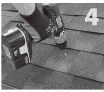
Using drill with 7/32" bit, drill pilot hole into roof and rafter, taking care to drill square to the roof. Do not use mount as a drill guide. Drill should be 'long style bit', aka 'aircraft extension bit' to drill a 3" deep hole into rafter.
