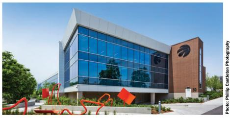
BioSteel Centre in Toronto features AviProTek® bird-friendly glass by Walker Textures® glass, acid-etched on tinted Optiblue® glass and Solarban® R100 glass. Trulite was the glass fabricator.
