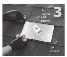
up so top edge of flashing is at least 3/4" higher than the butt-edge of the 3rd course and lower flashing edge is above the butt-edge of 1st course. Mark center for drilling.
