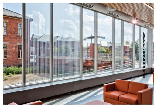
The bird-friendly glass in the Humber College Centre for Entrepreneurship in Toronto was fabricated by Trulite. The project incorporates AviProTek® bird-friendly glass by Walker Textures® glass, acid-etched on tinted Solarban® 70XL glass.
