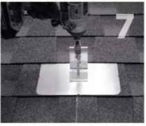
Prepare lag bolt or structural screw with sealing You are now ready for the rack of your choice. can no longer easily rotate. DO NOT over-torque. NOTE: Structural screw can be driven with T-30 hex
