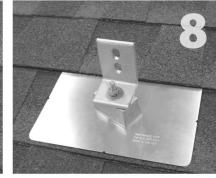
Insert EPDM rubber washer over hanger bolt into Using the rack kit hardware, secure the racking (L-foot) to the mount using torque specs from racking manufacturer. If racking manufacturer does not specify torque setting, tighten to 13 ft.-lbs.
