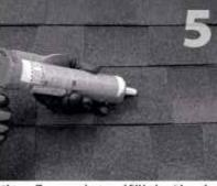
If attaching with lag bolt use a 1/32 bit (Lag). Use a Clean off any sawdust, and fill hole with sealant Place L-foot onto elevated flute and rotate L-foot to
