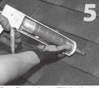
Clean off any sawdust, and fill hole with sealant compatible with roofing materials.
