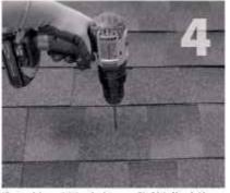
%" bit (ST) for attaching with the structural screw. compatible with roofing materials. Drill pilot hole into roof and rafter, taking care to drill square to the roof. Do not use mount as a drill guide. Drill a 2" deep hole into rafter.
