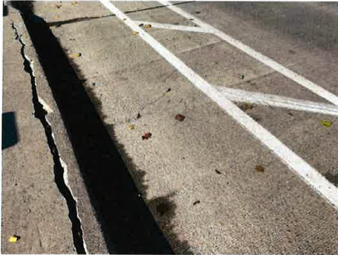
Document Name: IMG_2093.JPG Category: Deck Span Number: Comments: Crack at back on curb, South Sidewalk
