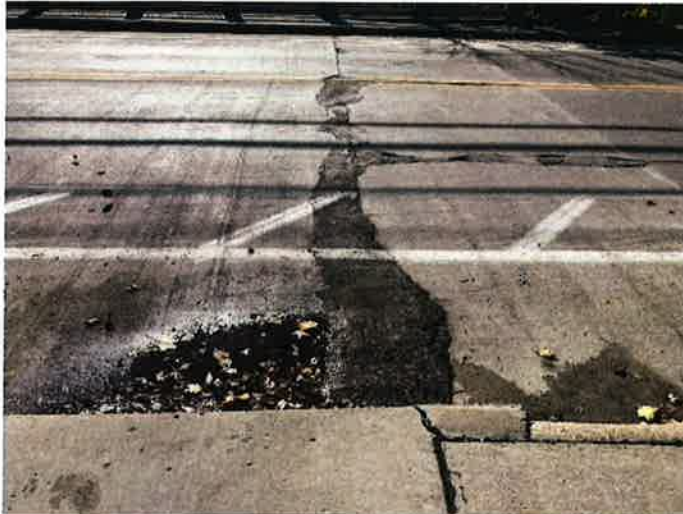
Document Name: IMG_2100.JPG Category: Deck Span Number: Comments: Ponding Water at Curb NW Quadrant Near Abutment
