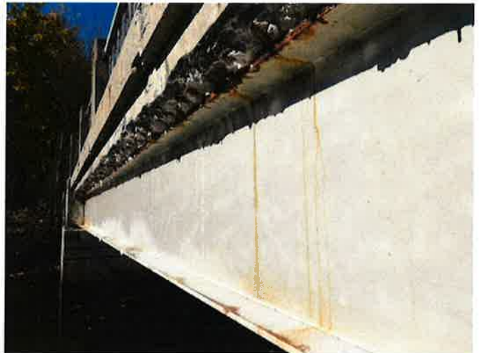
Document Name: IMG_2113.JPG Category: Deck Span Number: Comments: Spalling and Efflorescence, North Deck Fascia
