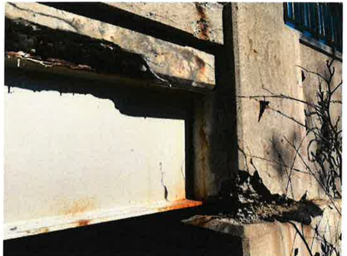
Document Name: IMG_2114.JPG Category: Superstructure Span Number: Comments: Spall in SE Corner of Headwall
