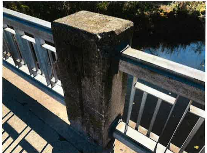
Document Name: IMG_2106.JPG Category: Railing Span Number: Comments: Spall at 2nd Railing Post, SW Quadrant
