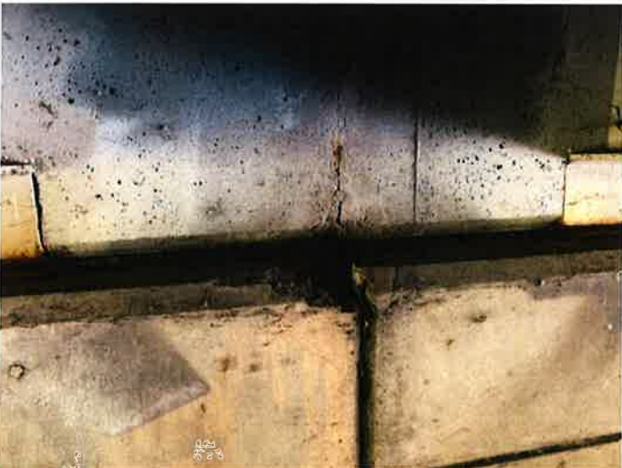
Document Name: IMG_2117.JPG Category: Substructure Span Number: Comments: Spall Near Construction Joint, East Abutment
