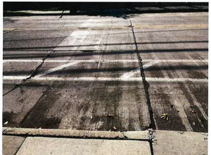
Document Name: IMG_2094.JPG Category: Approach Span Number: Comments: Cracks and Spalls, East Approach Pavement
