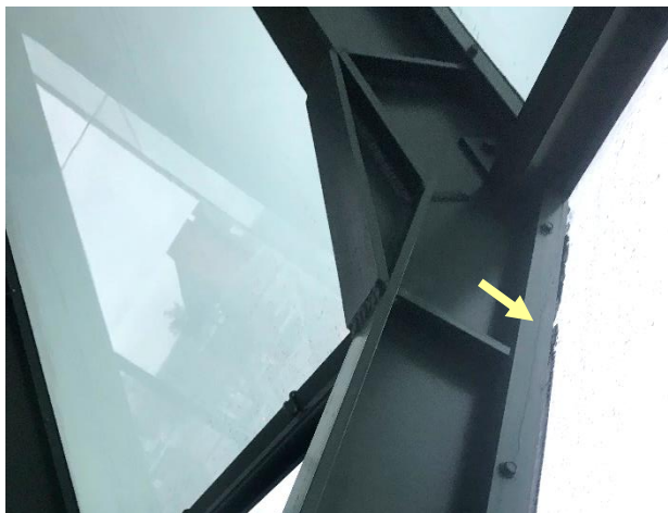
Figure 11. Water tracking down glazing column.
