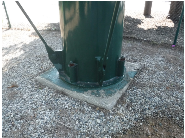
5) The leg foundations are in good condition with no deterioration.
