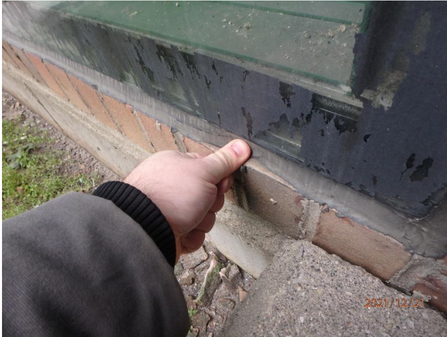
Figure 18. Adhesive failure of sealant at elevator shaft curtainwall.
