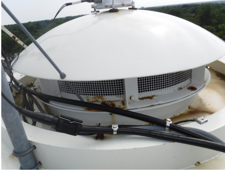
34) Coating failures on the roof vent.
