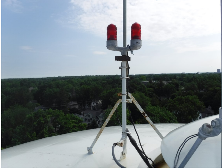
37) The double aviation light appears to be in good condition.
