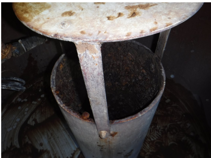
60) The fill/draw pipe enters the bottom of the riser and has a deflector plate over the pipe. The pipe and plate are in good condition.
