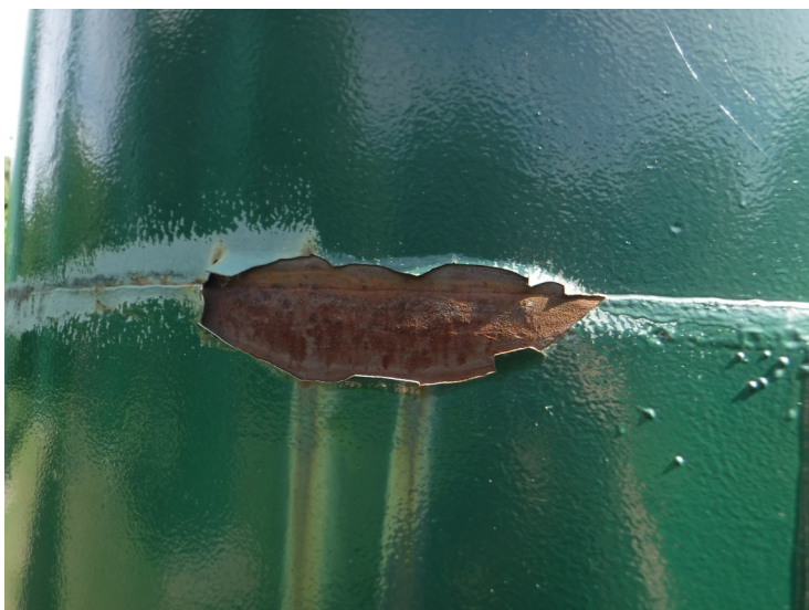
15) Spot coating failure with rust undercutting on a leg weld seam.
