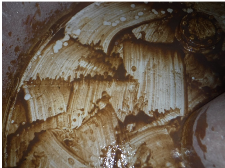
59) The bottom of the riser is in good condition overall with no coating failures.
