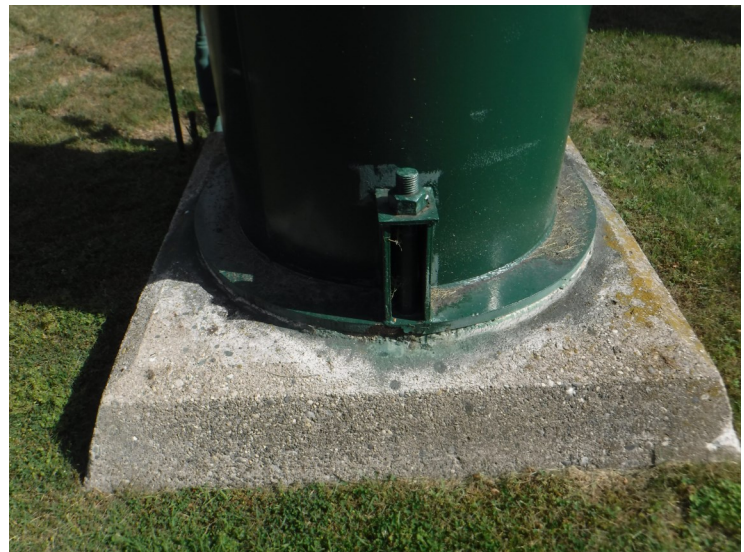
8) Typical leg anchor bolt that is in good condition.
