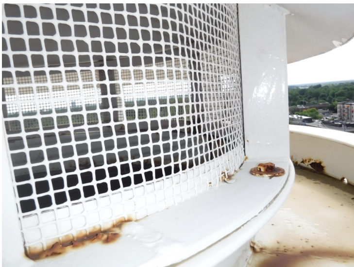
36) There is no rain shield on the vent.
