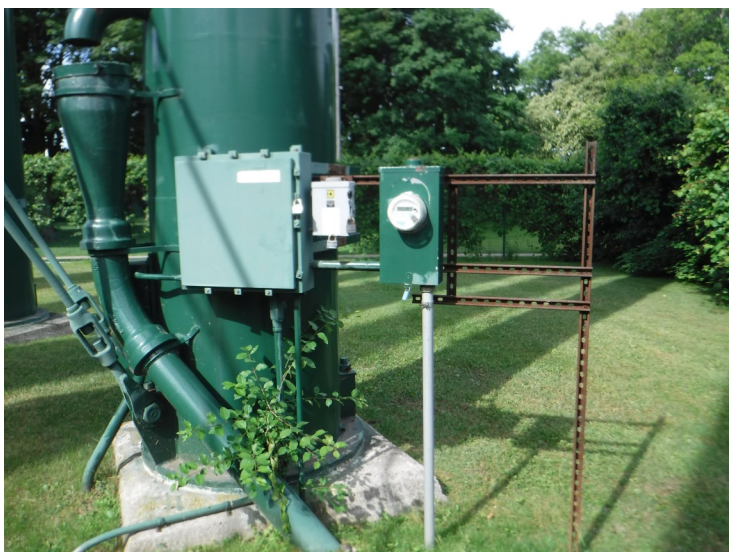
12) The overflow pipe routes underground.
