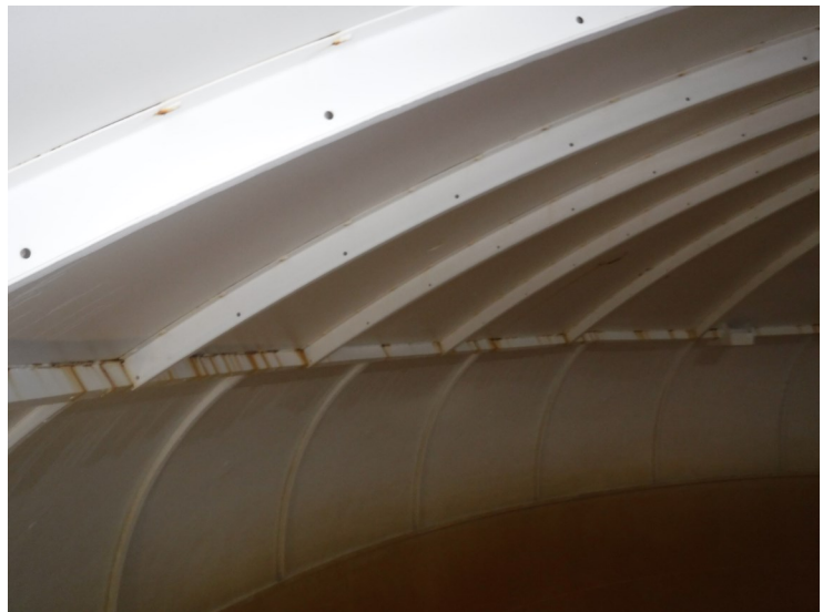
38) Coating failures on the wet interior roof.
