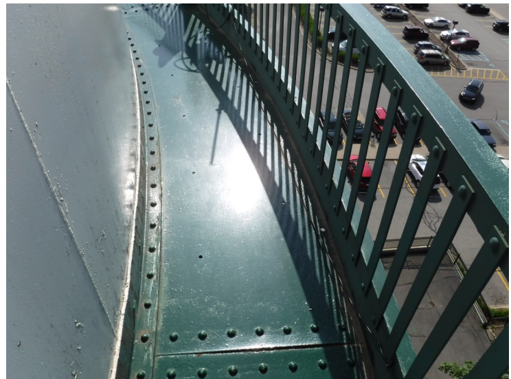
20) The coating on the balcony is in good condition with no significant deterioration.
