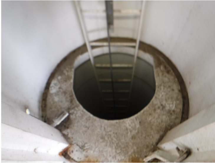
34) The top platform in the leg is in good condition.
