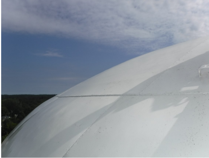
31) The roof coating is in good condition overall with minor failures.
