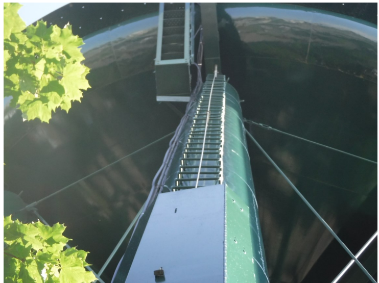
14) The leg ladder is in good condition. The ladder is equipped with a fall prevention device.
