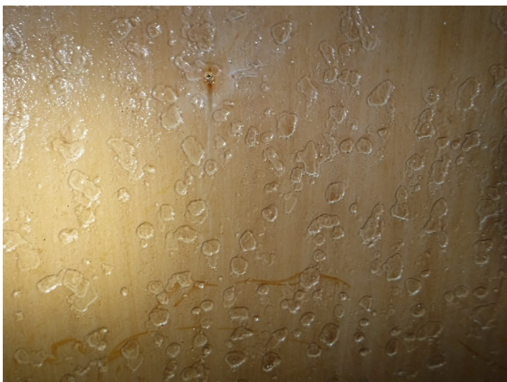
57) Small pinhole coating failure in the riser.
