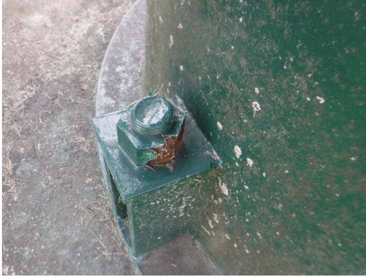
4) Spot coating failure on an anchor bolt.
