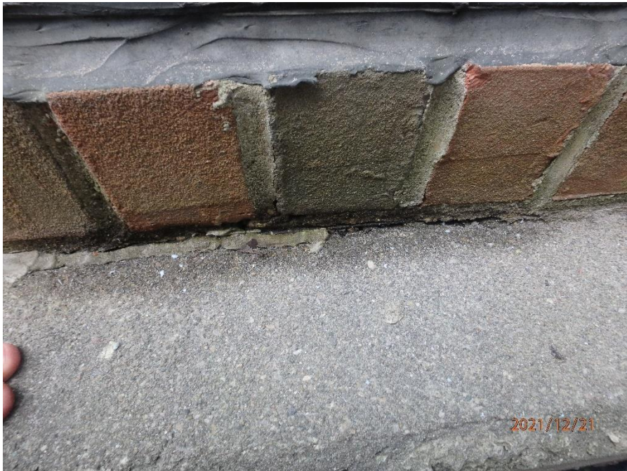
Figure 21. Damp appearance at mortar and concrete. Concrete is not pitched to drain. Sealant is applied at mortar bond failure to concrete.
