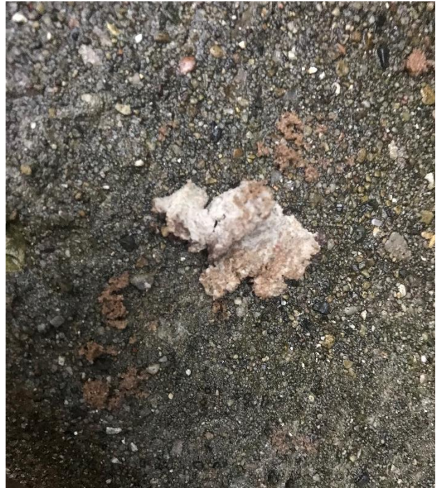
Figure 15. Light gray waterproofing is not a sheet product.
