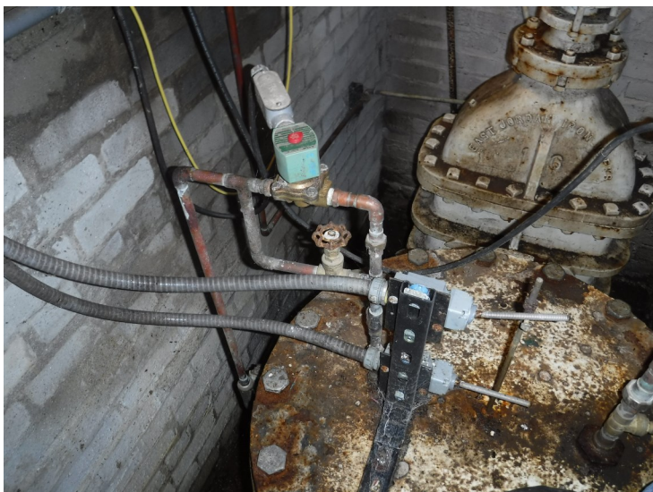
60) There are a few different connection points that could serve as a chemical feed line.
