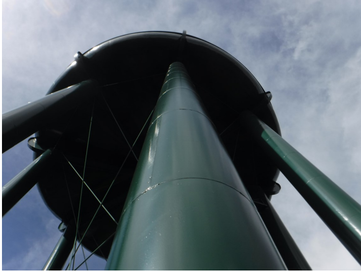
16) The leg coating is in good condition overall.
