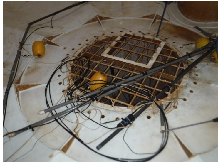
53) The cathodic protection system appears to have broken supporting ropes.
