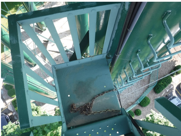
15) The step-off platform at the top of the leg ladder is in good condition.
