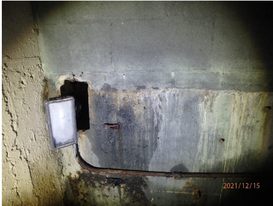
Figure 3. Water entry observed on the south wall at the horizontal joint between the concrete foundation wall below and CMU shaft wall above. The south wall is an interior wall separating the elevator shaft from Stair B.
