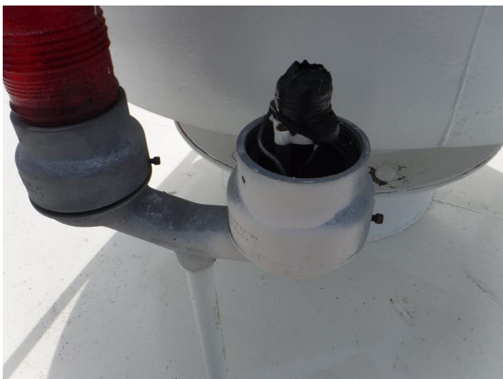
27) One globe is missing and the socket is taped over.
