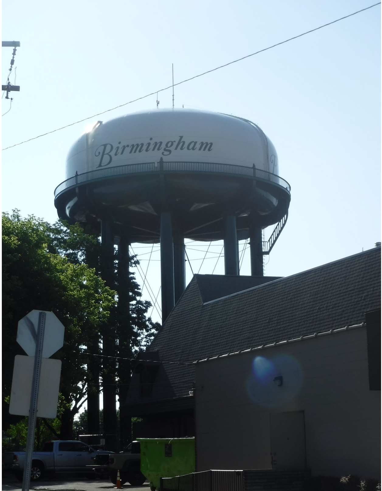
500,000 gallon radial arm (Hunter) elevated water storage tank located in Birmingham, Michigan.
