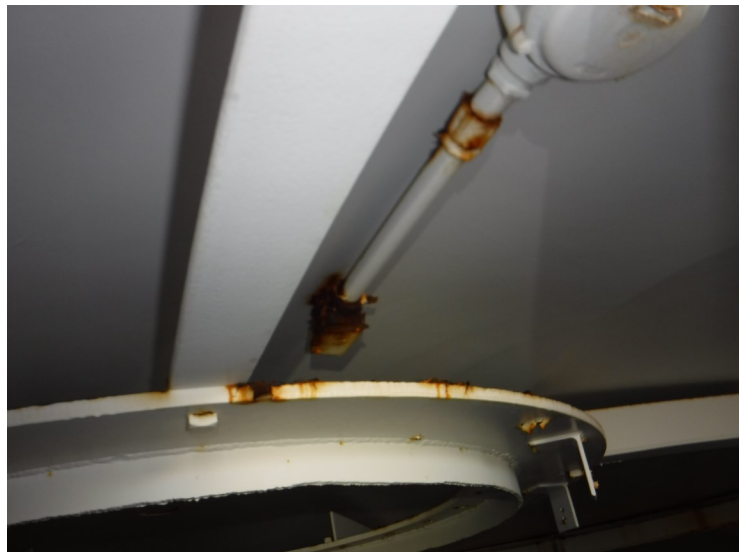
44) Spot coating failures on a conduit section.
