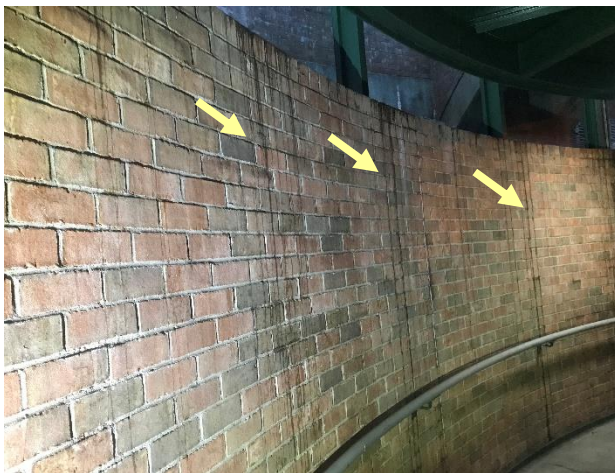
Figure 9. Water tracking down inboard surface of brick.
