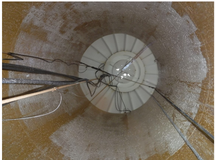
53) The riser coating is in good condition overall.
