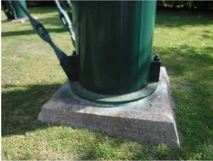
7) The leg foundations are in good condition. There is some exposed aggregate on the foundations.
