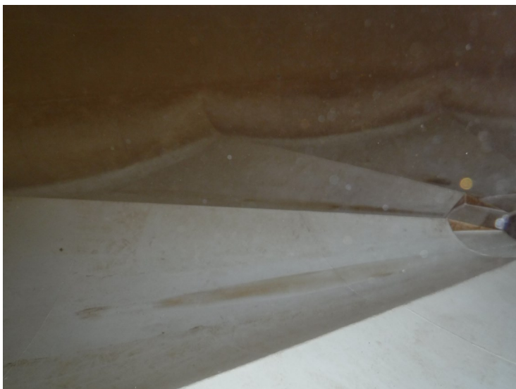
48) Minor pinhole coating failures in the bowl.
