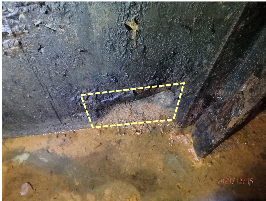
Figure 5. Void observed near the middle of the base of the south wall.
