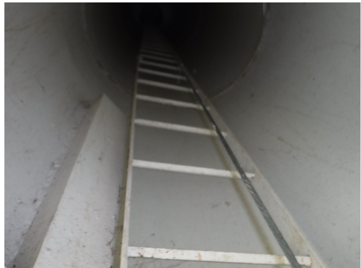
32) The leg ladder is in good condition. The ladder is equipped with a fall prevention device.
