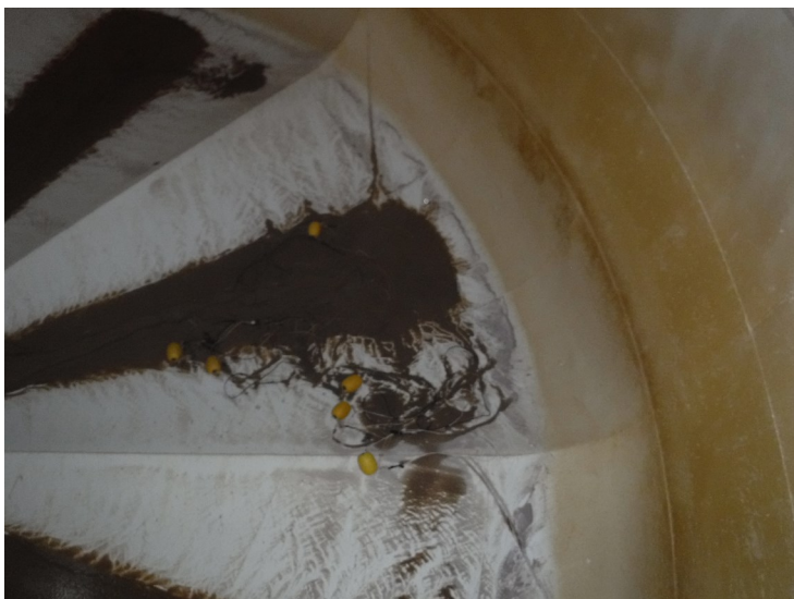
45) Broken ropes supporting the cathodic protection system.
