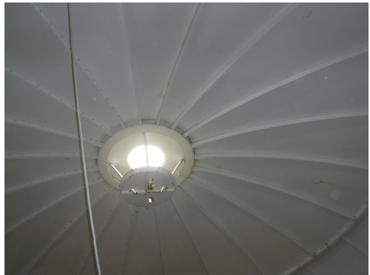
41) The wet interior roof coating is in good condition overall.
