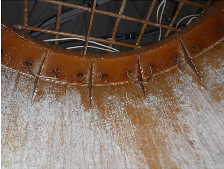
55) The riser coating is in good condition overall.
