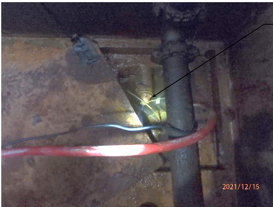
Figure 2. Elevator sump pit during water removal using a portable pump and red hose.
