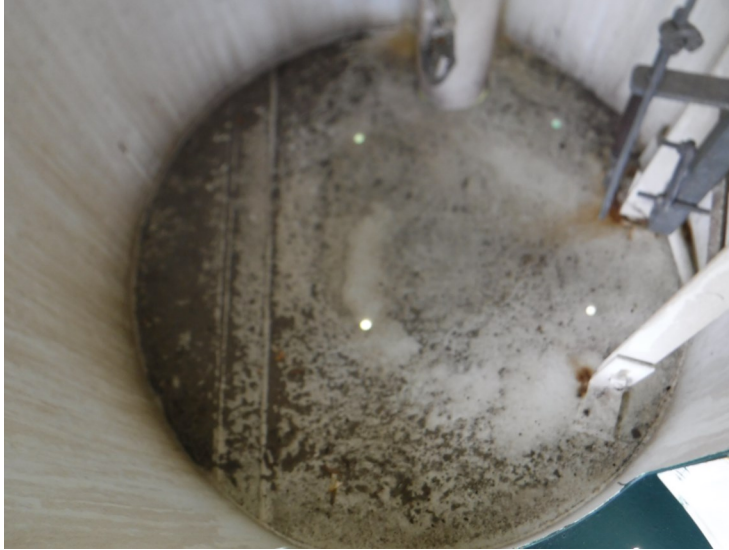
37) The access tube floor coating is in good condition.
