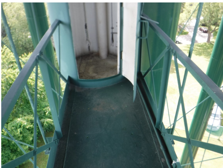
18) The catwalk between the access leg and access tube is in good condition.
