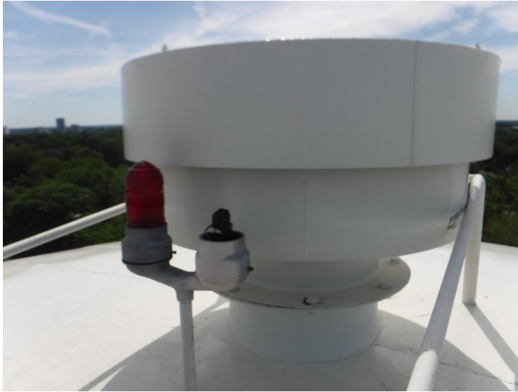
22) The pressure vacuum vent is in good condition.
