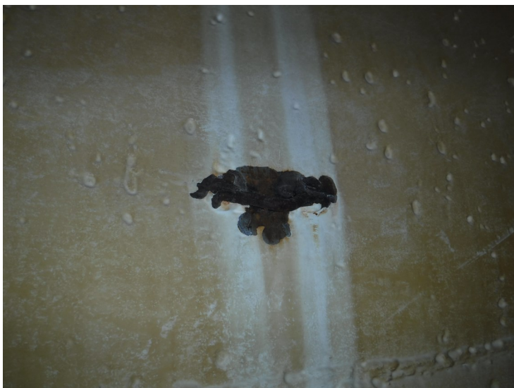
51) A spot coating failure in the wet riser.
