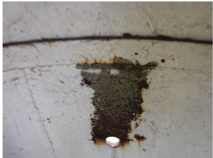
35) Spot coating failures in the dry interior leg.
