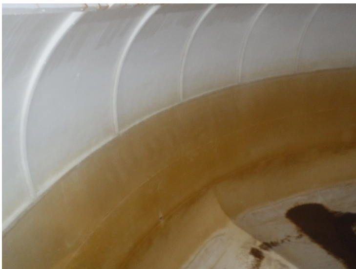
42) There is no significant coating deterioration on the wet interior sidewall.
