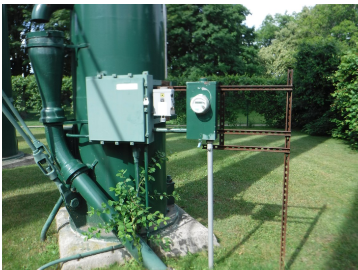
12) The overflow pipe routes underground.
