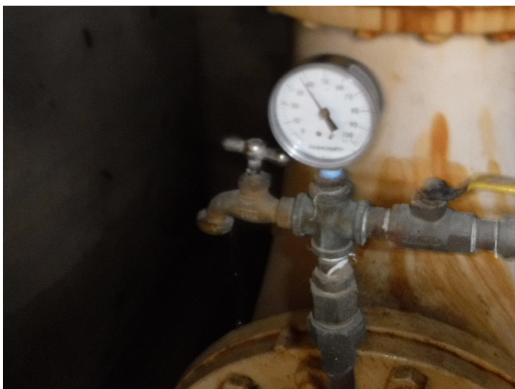
63) The sample tap is in good condition but is threaded.
