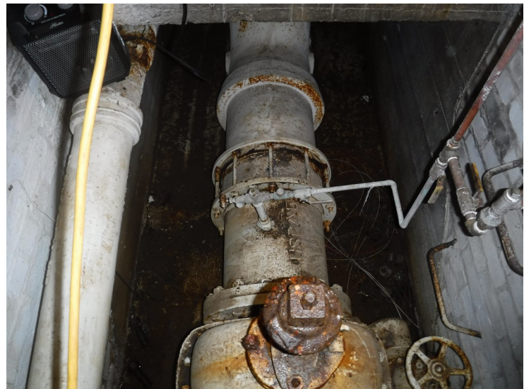
59) Coating failures on the pit piping. There is a threaded sample tap on the piping.
