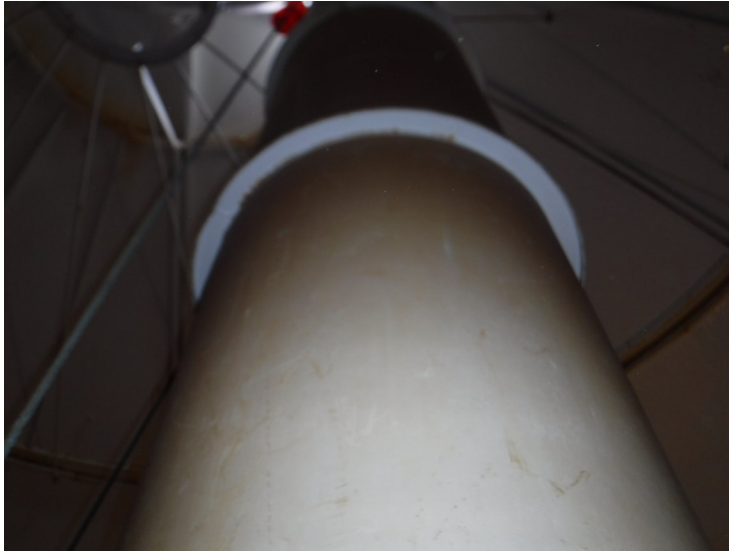
49) The access tube coating is in good condition overall.
