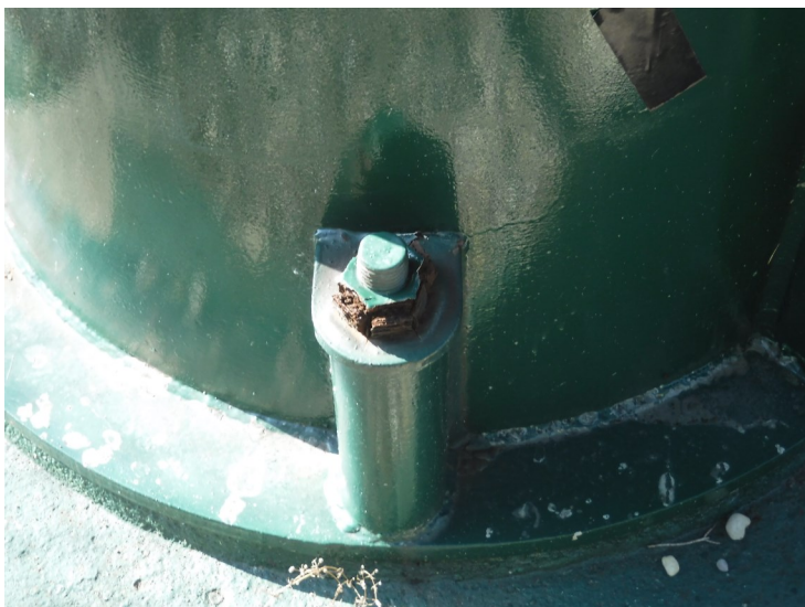
6) There is heavy corrosion on several of the anchor bolt nuts on the legs.
