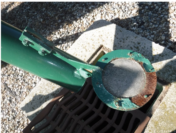
12) The screened flap gate on the overflow pipe is in good condition.
