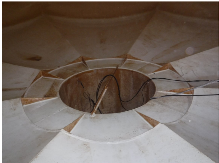
50) There is no safety grate over the riser in the wet interior.
