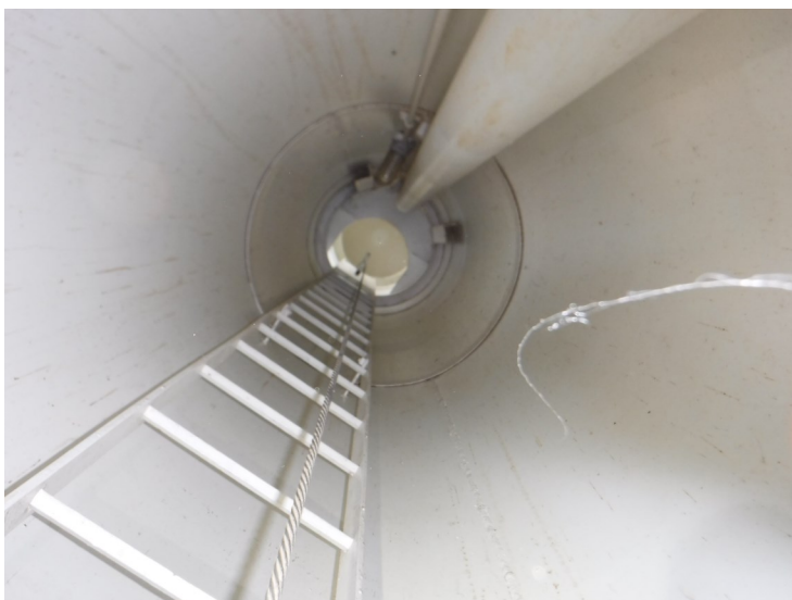
33) The dry interior leg coating is in good condition with no significant deterioration.
