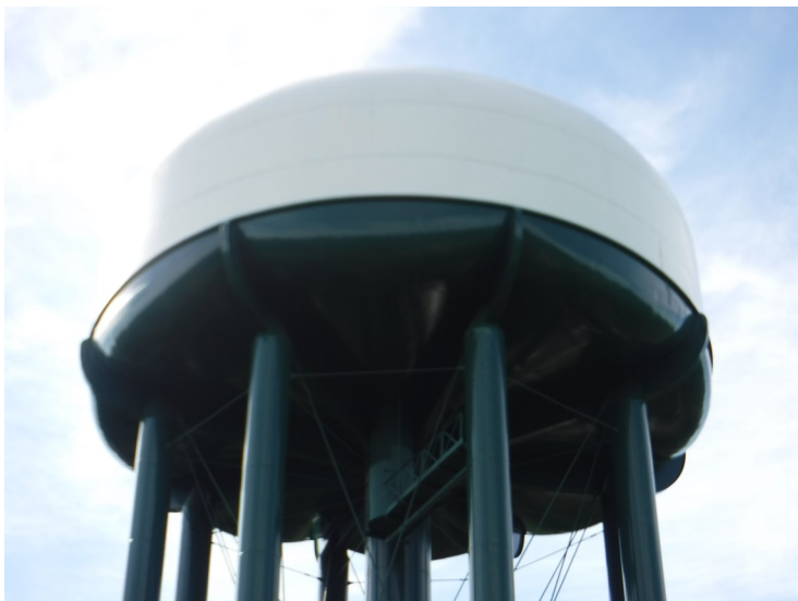
21) The sidewall coating is in good condition overall.
