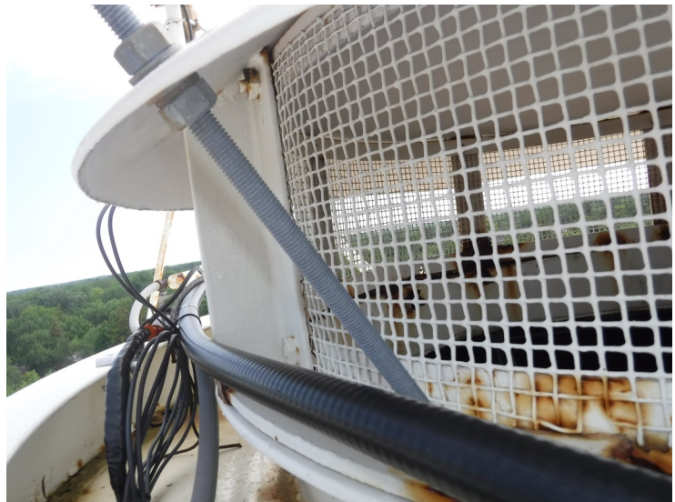
35) The roof vent screen is in good condition, but is oversized.
