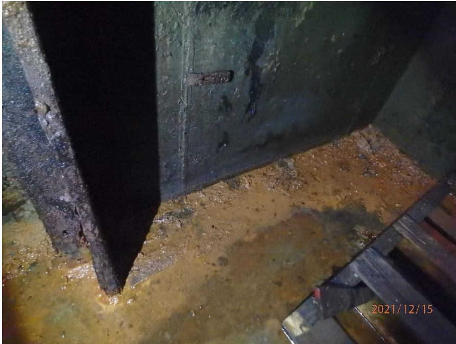
Figure 1. Water on floor of elevator pit. Note the walls are painted green and are not exposed concrete.
