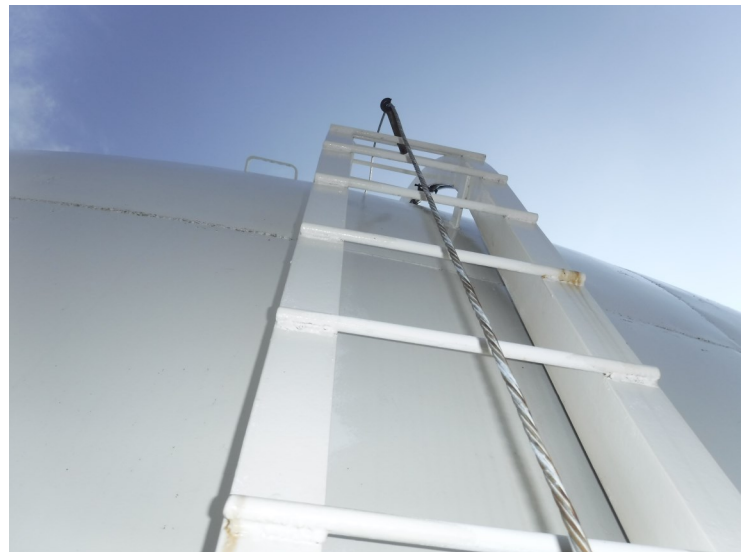
26) The sidewall/roof ladder is in good condition. The ladder is equipped with a fall prevention device.
