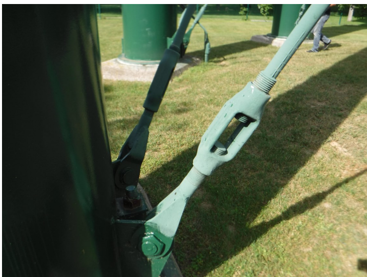
9) Typical tie rod connection that is in good condition. There are clear coat failures on the tie rods.
