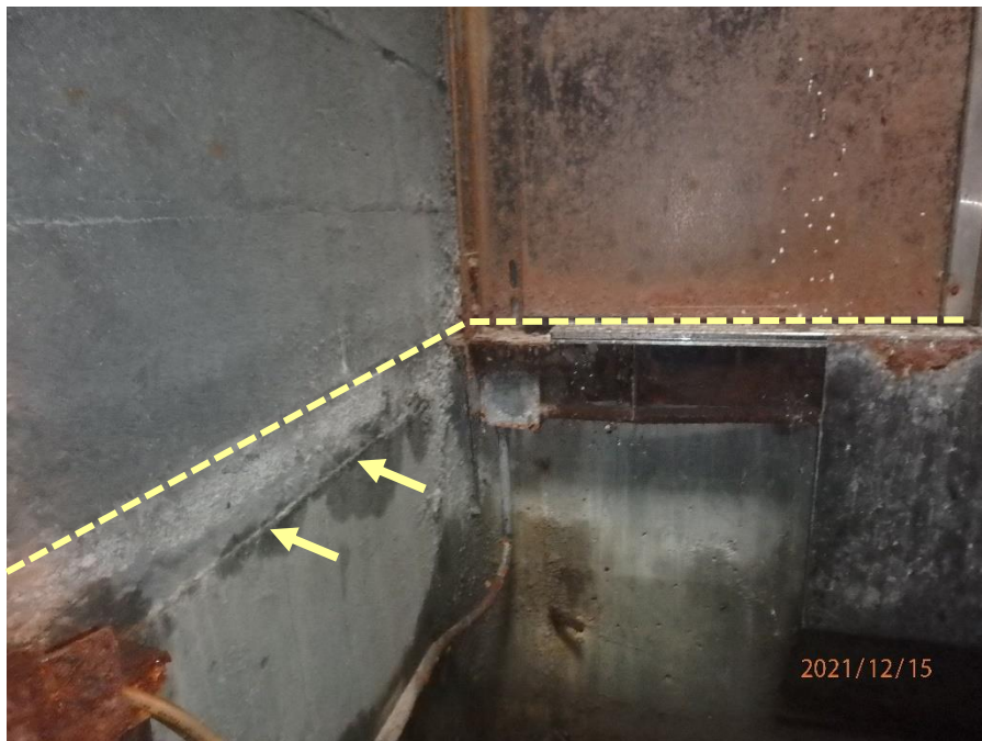
Figure 4. The horizontal joint is intermittently damp along the south wall of the elevator shaft. There is one course of brick-sized concrete masonry present below the floor level, resulting in the water infiltration occurring approximately 3-1/2" below the floor elevation of the stairs, depicted by the yellow dashed line.
