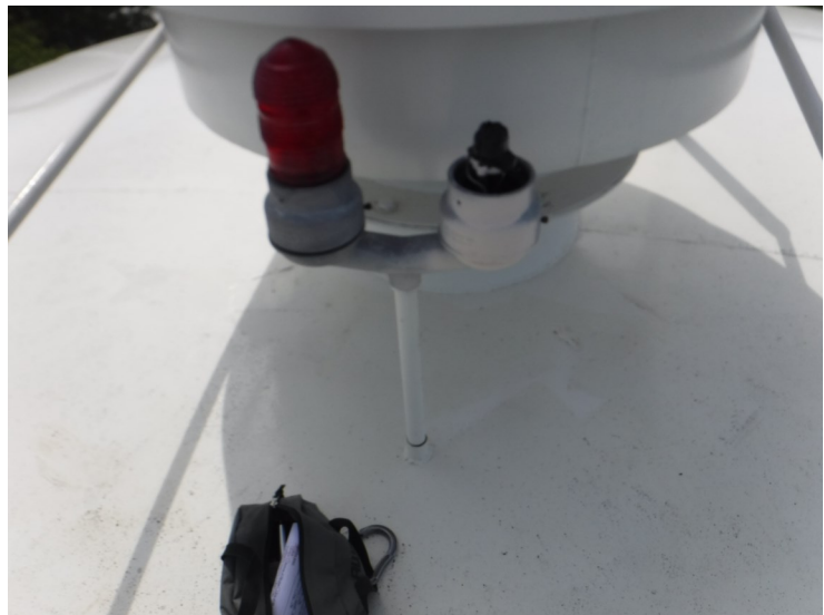
26) The double red aviation light is in poor condition.
