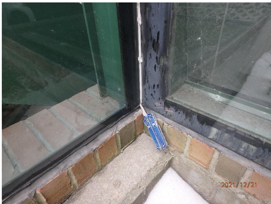
Figure 19. Sealant defects with white remedial sealant present. The probe is inserted in a void in the sealant. Above the probe the untooled white sealant is assumed to cover a defect along the joint.
