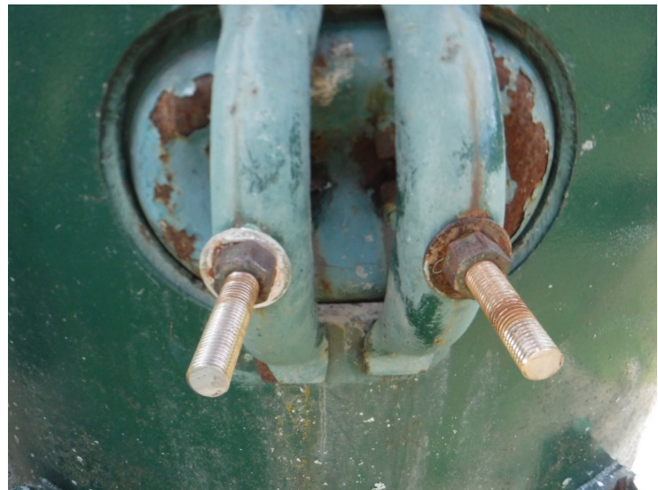
5) The riser manway is in good condition. Spot coating failures on the cover and bolts.
