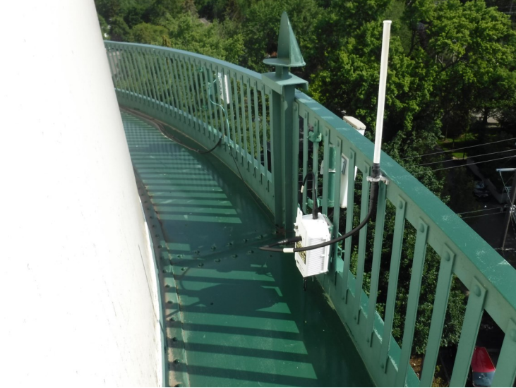
22) There are loose antenna cables on the balcony.
