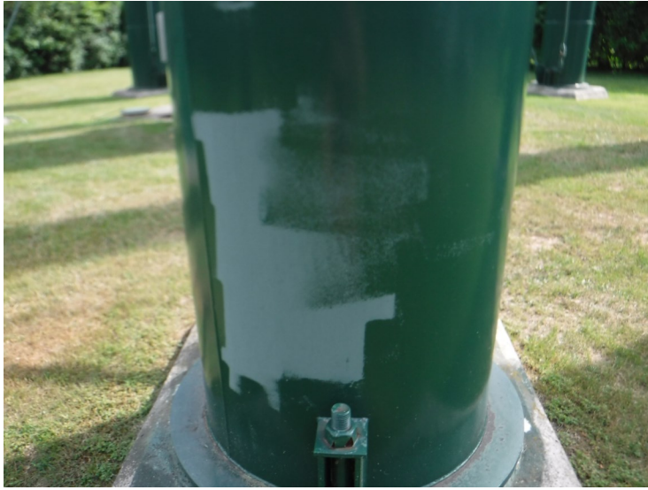
13) Clear coat failures at a leg section.
