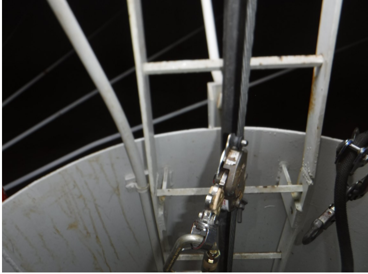
40) The top of the access tube is open to the wet interior.
