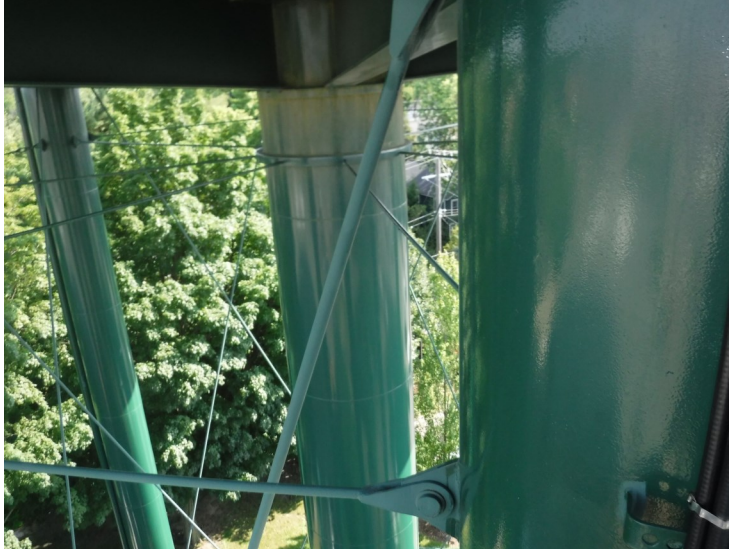
4) The riser tie rods are in good condition.
