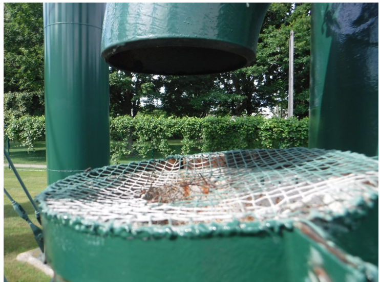
11) The overflow discharge is not screened.
