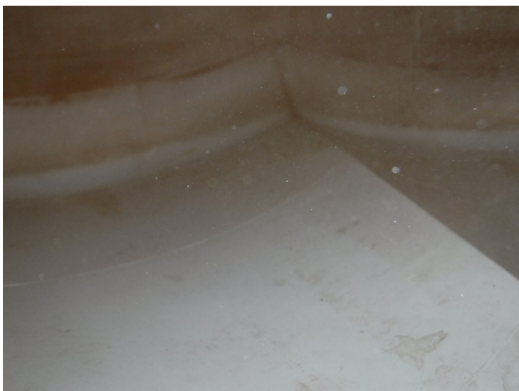
51) Typical bowl section with no significant coating failures.
