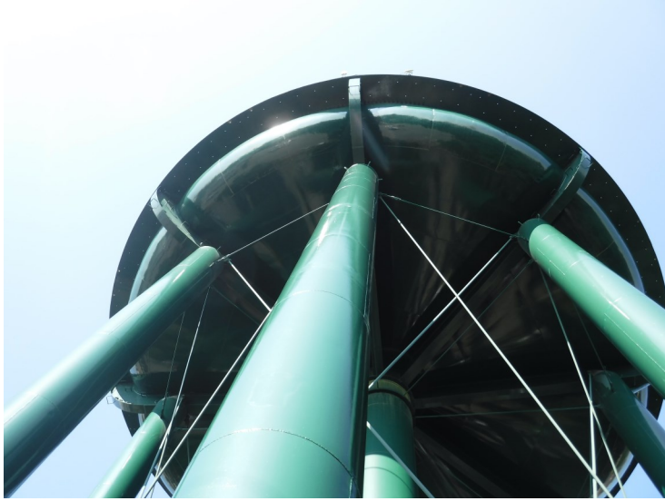
10) The sway rods are in good condition.
