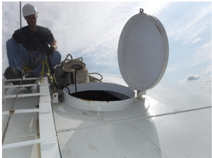
29) The wet interior roof hatch is in good condition.
