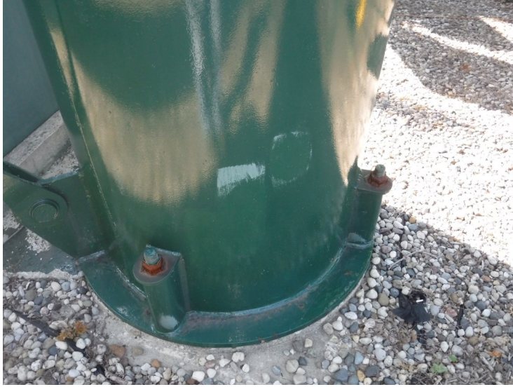
7) Coating failures on a leg.
