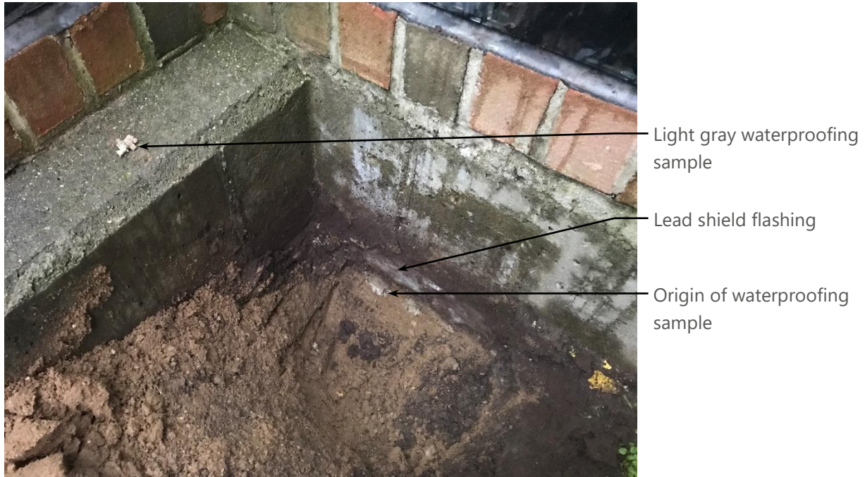
Figure 13. Shallow excavation to observe foundation waterproofing.
