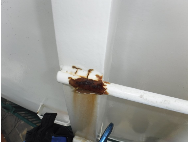
28) Coating failure on the sidewall/roof ladder.
