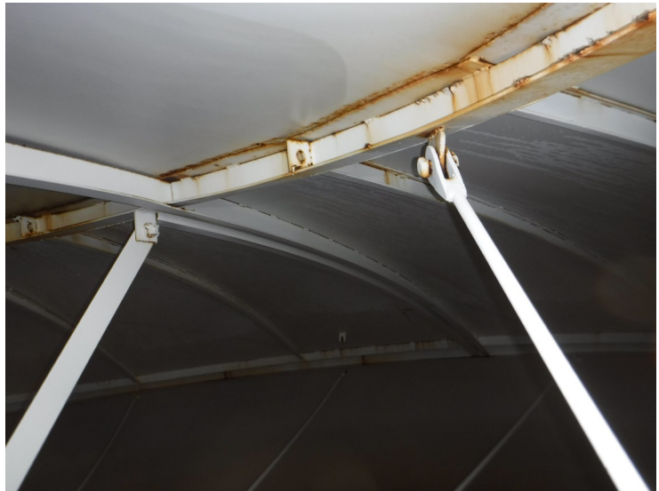
41) The wet interior roof coating is in good condition. There is rust bleedthrough at the lap seams and gap above the roof beams.
