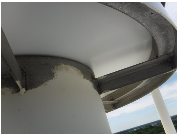
24) The pressure plate is in good condition. The plate was found to be properly aligned during the inspection.
