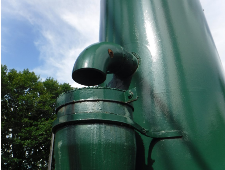
10) The overflow pipe and funnel are in good condition.
