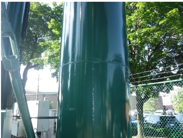
9) The coating on the legs is in good condition overall.
