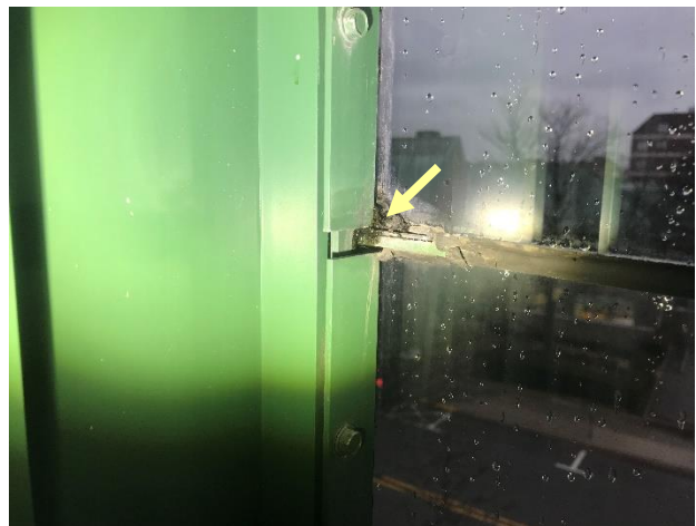
Figure 12. Water entry at glazing column.
