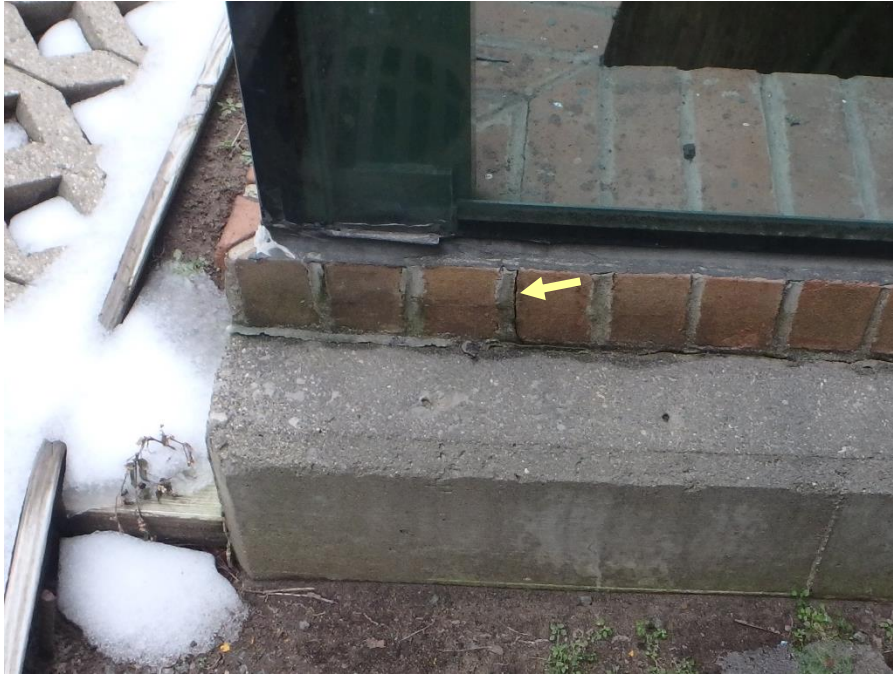
Figure 20. Mortar bond failure at brick sill.
