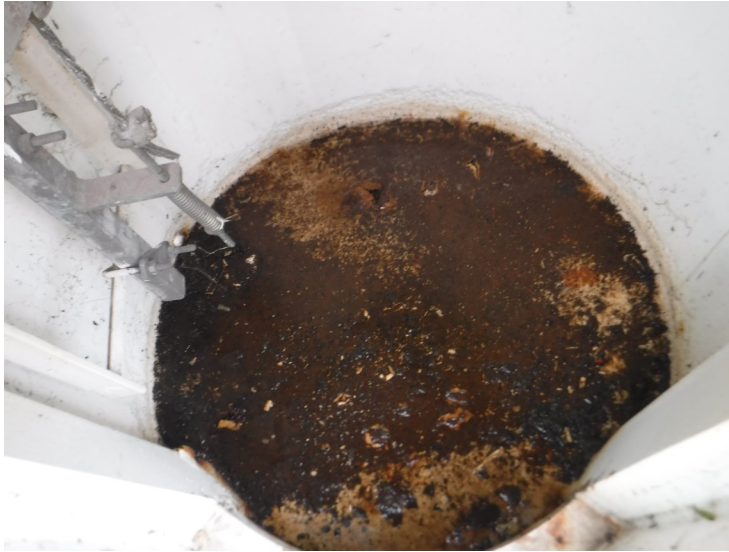
31) Spot coting failures at the bottom of the access leg.
