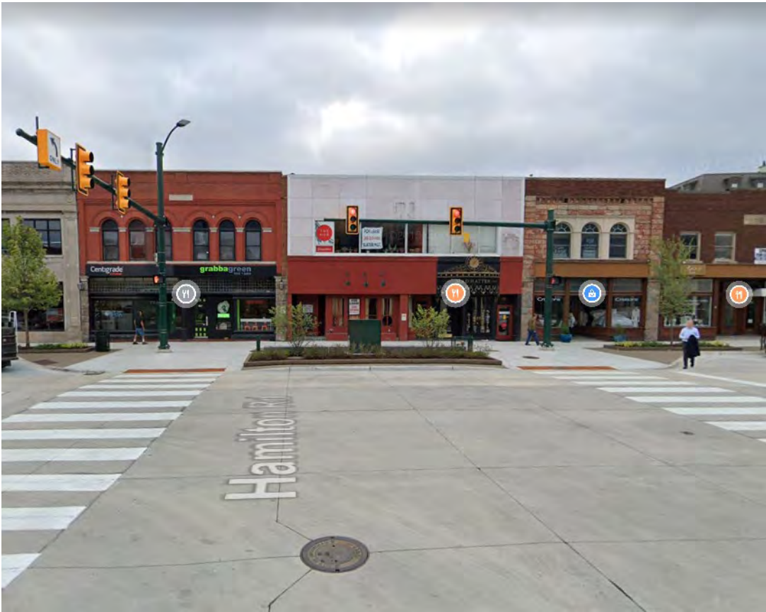
3 - Electric box design at N. Old Woodward and Hamilton Row
