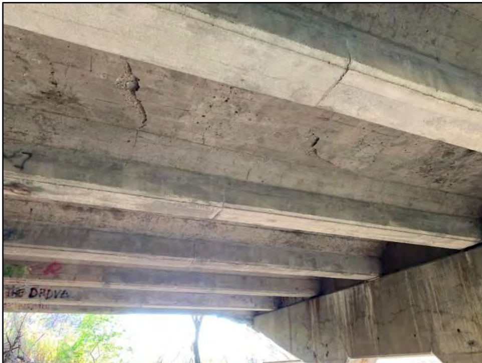
Deck delamination in east span
