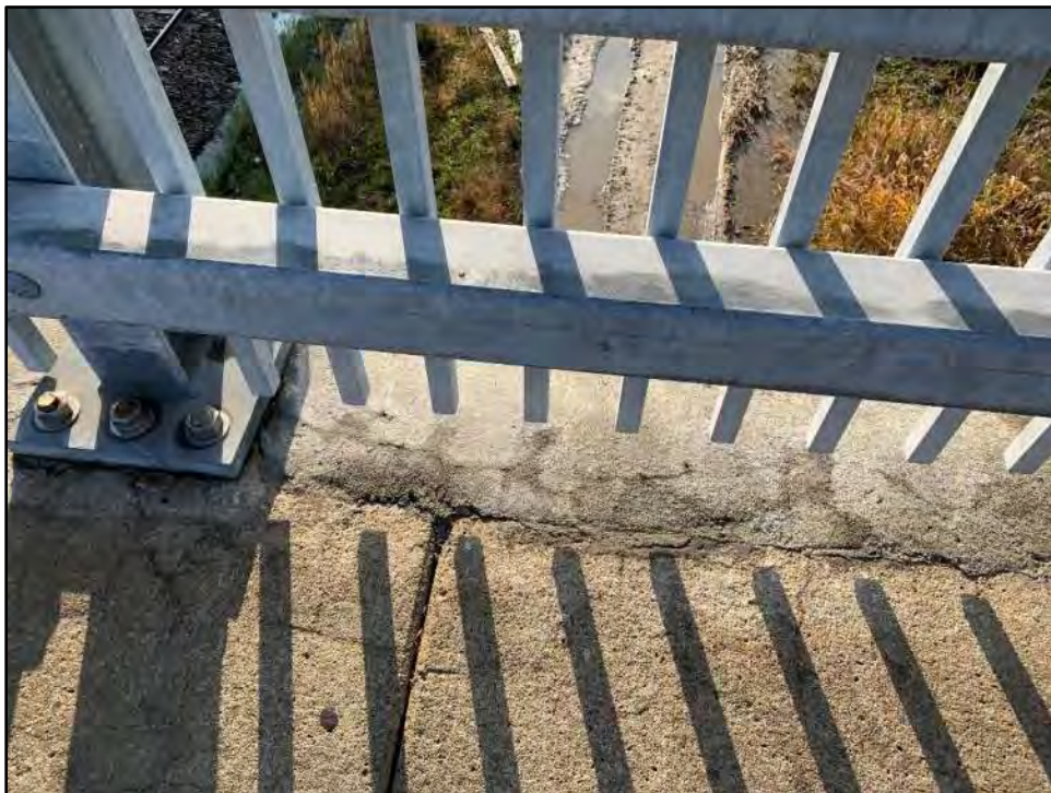
Hairline cracking in top surface repair of sidewalk under railing in southwest quadrant
