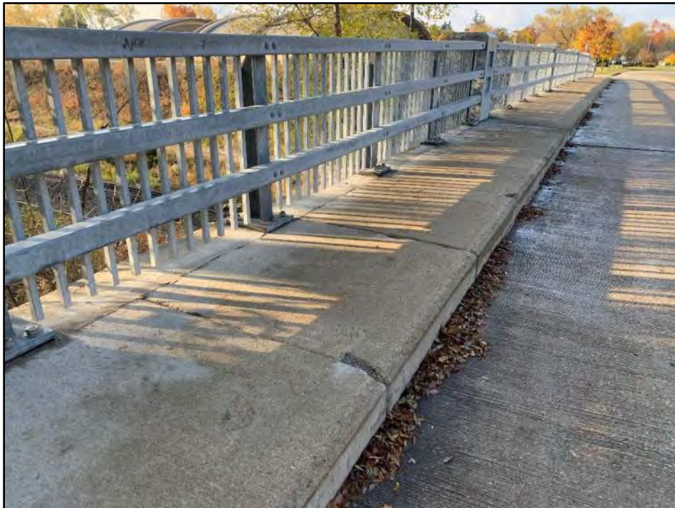
Spalling of south sidewalk
