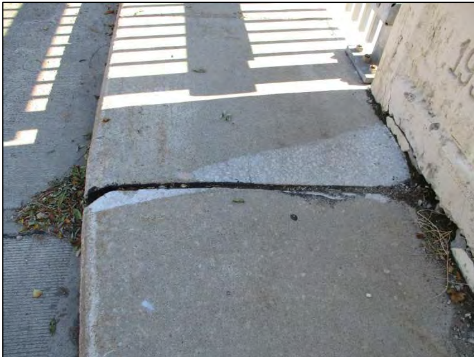
Sidewalk deterioration at abutment
