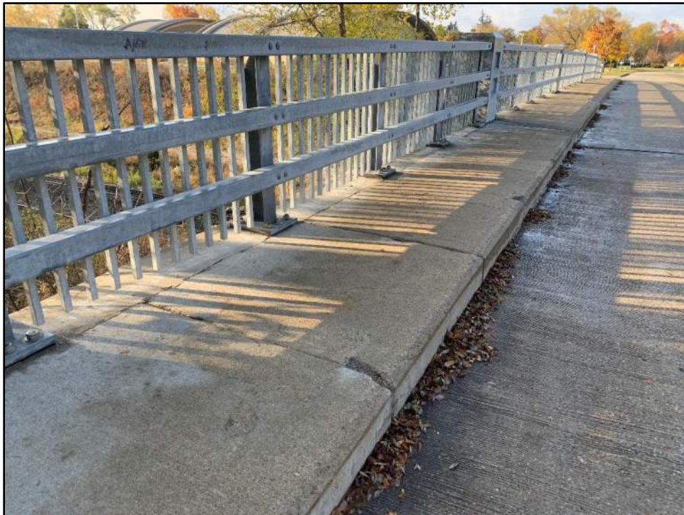
Spalling of south sidewalk
