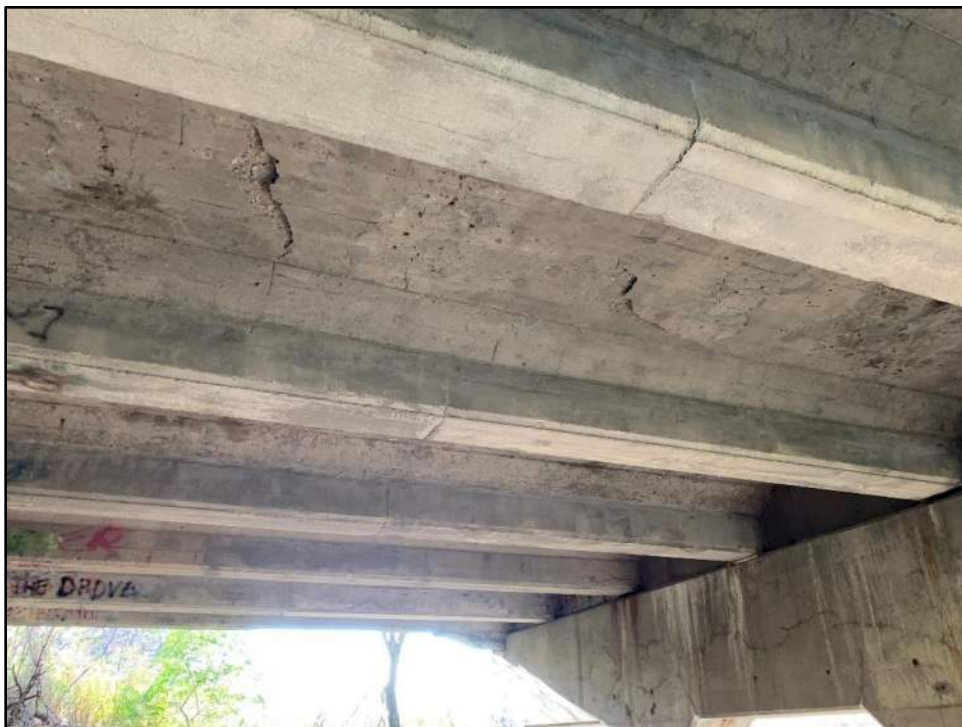
Deck delamination in east span
