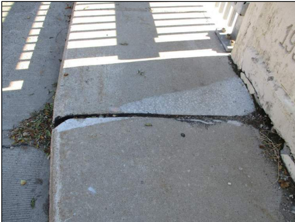
Sidewalk deterioration at abutment
