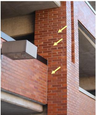
Figure 7. Distress at Column 19A prior to brick removal.
