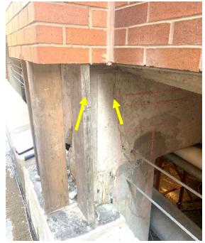
Figure 14. Cracks in west and south faces of Column 11A extend toward a converging point.
