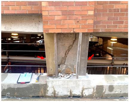
Figure 8. Brick veneer removed at Column 11A (west face) and supported by wood framing indicated with red arrows.
