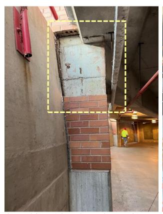
Figure 1. Column 10J inspection opening at Level 1 PT beam end (brick veneer removed).
