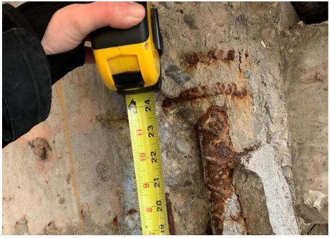
Figure 6. 24 inches from curb to first exposed stirrup at Column 10A.
