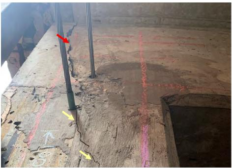
Figure 11. Cracks throughout concrete at Column 11A. Crack propagates through original concrete above as indicated with red arrow. Note the displacement across the crack in the original concrete where the concrete material has spalled.
