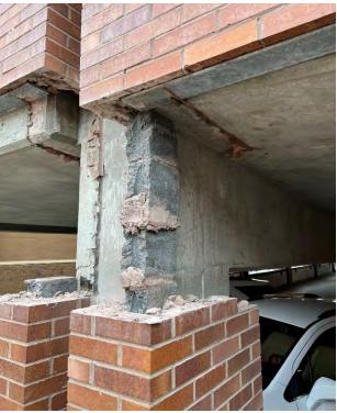
Figure 4. Column 19A inspection opening at Level 2 PT beam end (brick veneer at concrete block infill removed).
