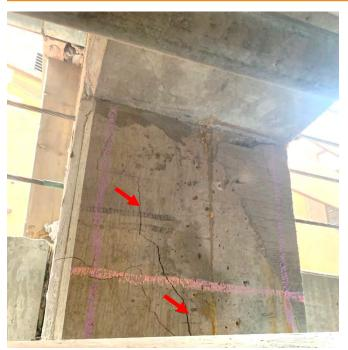
Figure 13. Cracks throughout original concrete at Column 11A.
