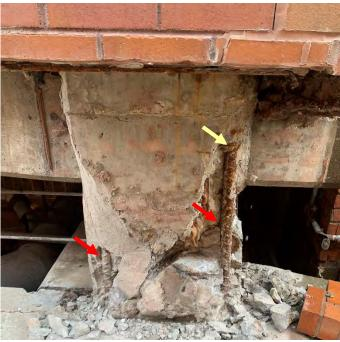
Figure 5. #11 longitudinal bars at corner of Column 10A are indicated with red arrows. Stirrup indicated with yellow arrow.
