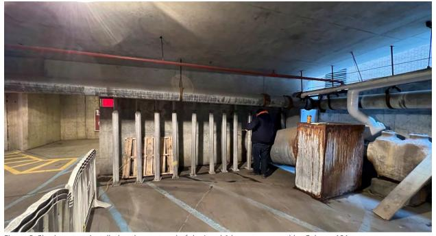
Figure 2. Shoring posts installed at the west end of the Level 1 beam supported by Column 10A.
