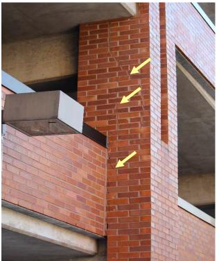
Figure 7. Distress at Column 19A prior to brick removal.
