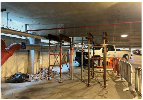
Figure 1. Shoring installed at the west end of the Level 1 beam supported by Column 11A.
