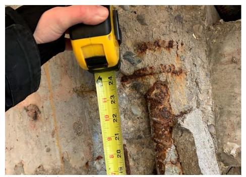
Figure 6. 24 inches from curb to first exposed stirrup at Column 10A.
