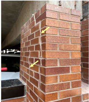
Figure 6. Brick distress below the existing inspection opening at Column 19A.
