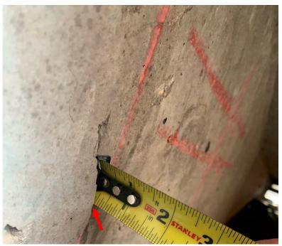
Figure 12. Approximately 1/4" displacement across crack in original concrete at Column 11A.
