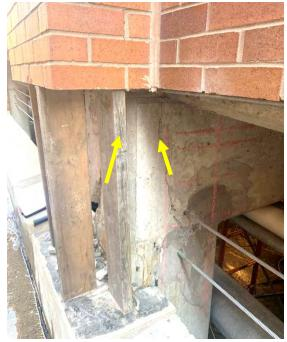
Figure 14. Cracks in west and south faces of Column 11A extend toward a converging point.
