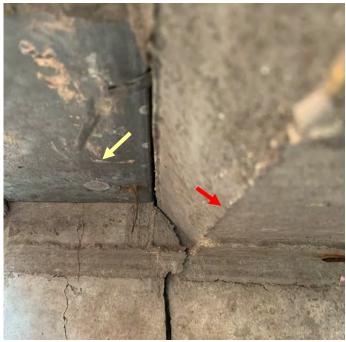
Figure 15. Crack in original concrete at south face of Column 11A extends along slab edge bearing at column. Slab indicated with red arrow and shelf angle indicated with yellow arrow.
