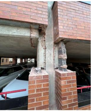
Figure 3. Column 19A inspection opening at Level 2 PT beam end (brick veneer at concrete block infill removed).
