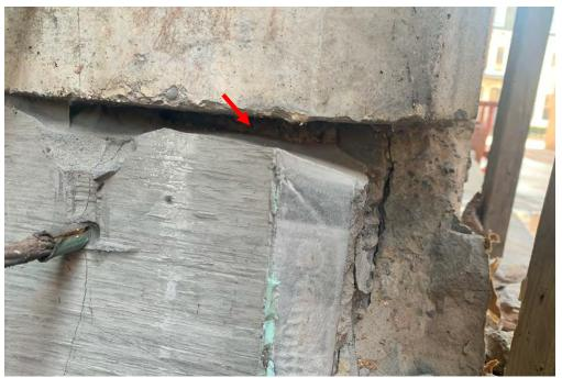
Figure 16. Wide cold joint at north face of Column 11A between original concrete and concrete repair. Joint is approximately four inches deep.
