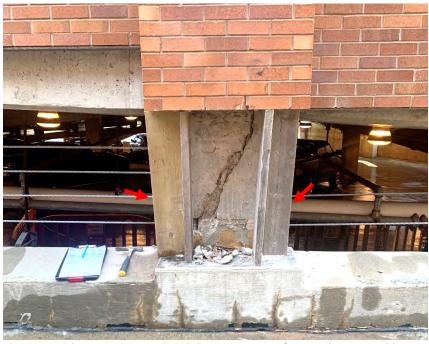
Figure 8. Brick veneer removed at Column 11A (west face) and supported by wood framing indicated with red arrows.
