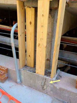
Figure 2. Column 12A inspection opening at Level 1 PT beam end (brick veneer removed, wood 2x installed as temporary support for brick). Note the concrete distress at the retaining wall.
