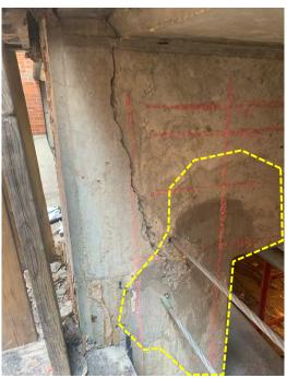
Figure 9. Previous concrete repair at beam to column interface at south face of column.
