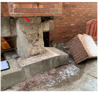
Figure 3. Brick veneer removed from the base of Column 10A. A steel shelf angle supporting the brick veneer indicated with red arrow.
