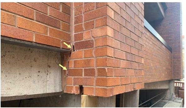
Figure 17. Cracks propagating through previous sealant repairs in the brick veneer at Column 11A.
