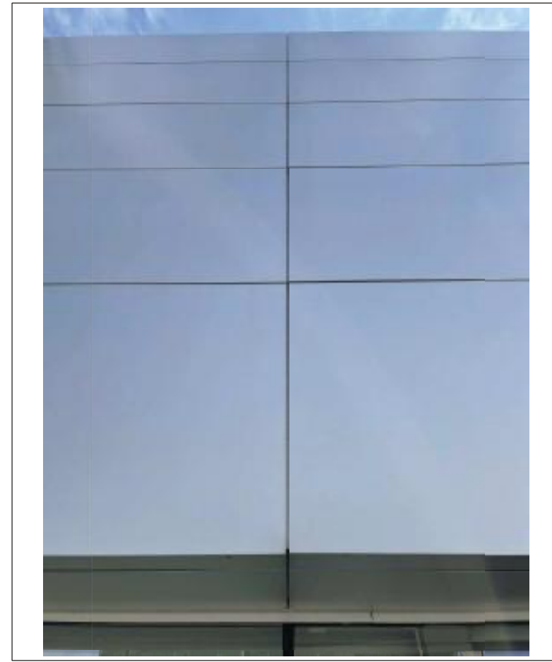
4 TYPICAL METAL COMPOSITE WALL PANELING (CP-1)
