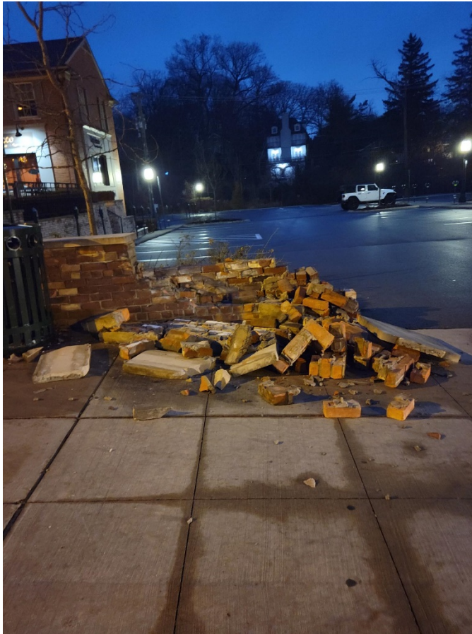
View East at Parking Lot No. 6
