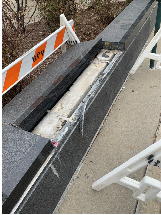
View North at Shain Park Parking Lot
