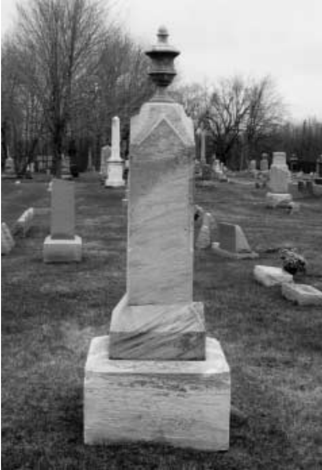
Obelisks (photo C) as well as larger, thicker tablets can be set onto a base (photo D).
