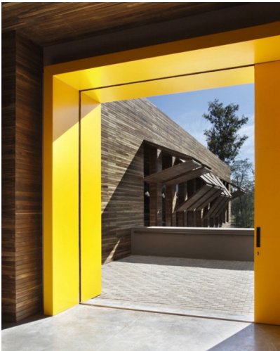
PROTRUDING PORTAL FRAME BUILT INTO EXISTING OPENING
