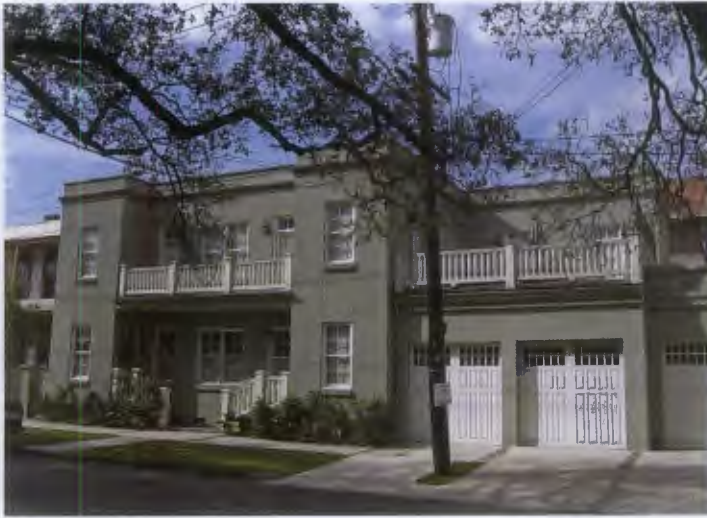
Figure 6. A new addition (left) is connected to the garage which separates it from the main block of the c. 1910 former florist shop (right). The addition is traditional in style, yet sufficiently restrained in design to distinguish it from the historic building.
