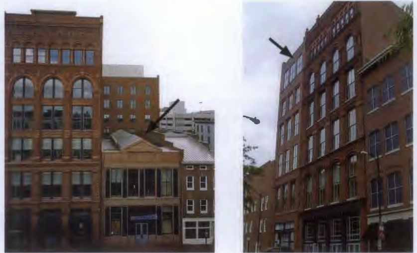
Figure 21. Both wings of this historic L-shaped building (top), which fronts on two city streets, adjoined vacant lots. A two-story addition was constructed on one lot (above, left) and a six-story addition was built on the other (above, right). Like the historic building, which has two different facades, the compatible new additions are also different and appear to be separate structures rather than part of the historic building.
