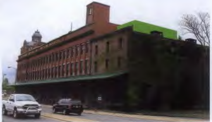
Figure 24. How to Evaluate a Proposed Rooftop Addition. A sight-line study (above) only factors in views from directly across the street, which can be very restrictive and does not illustrate the full effect of an addition from other public rights of way. A mock up (above, right) or a mock up enhanced by a computer-generated rendering (below, right) is essential to evaluate the impact of a proposed rooftop addition on the historic building.
