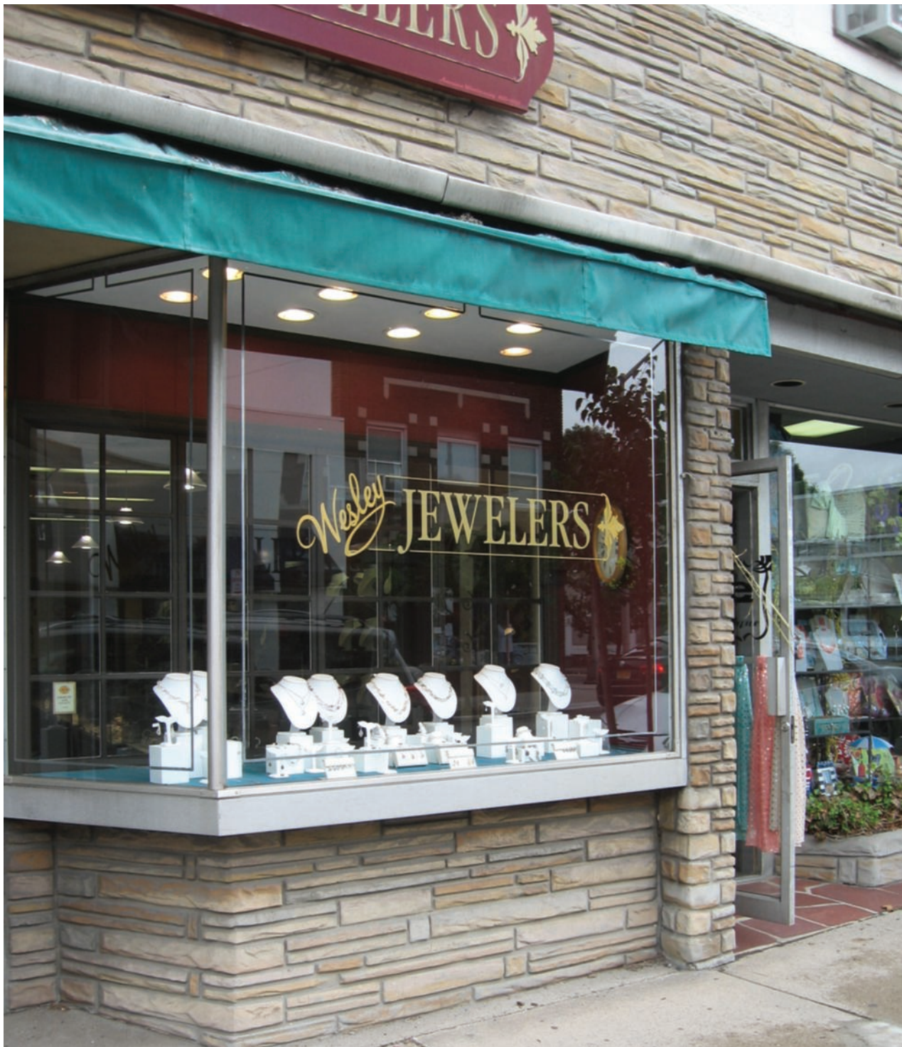
Figure 2: Thin slabs of stone veneer were widely used on remodeled storefronts in the 1950s and 1960s such as this example in Montclair, New Jersey.
