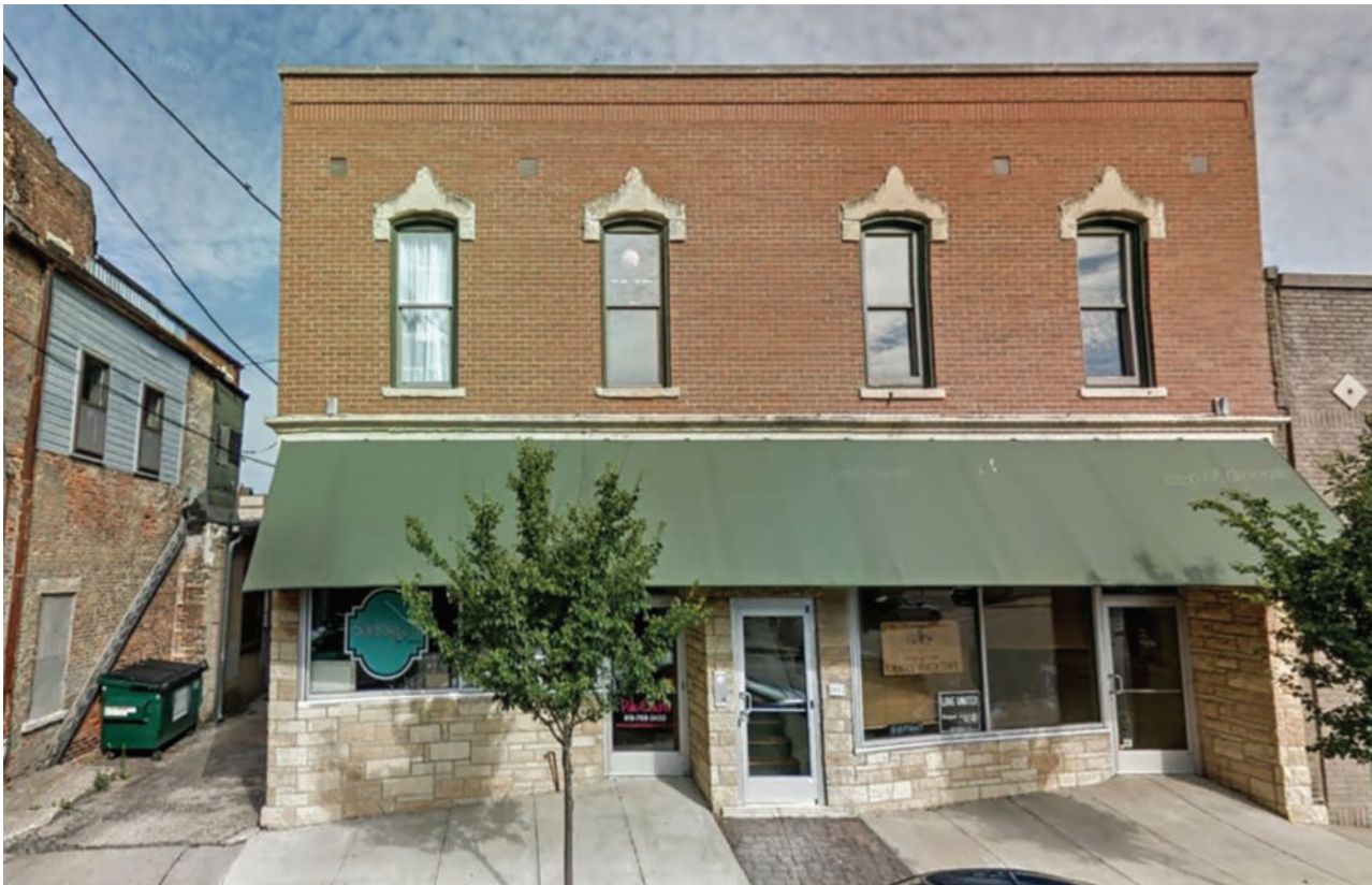
Figure 8: For purposes of the federal historic tax credit project the SHPO and NPS said that the midcentury storefront was historic, and required its retention. The owner kept the midcentury storefront and installed a compatible clear-view door and canvas awning.
