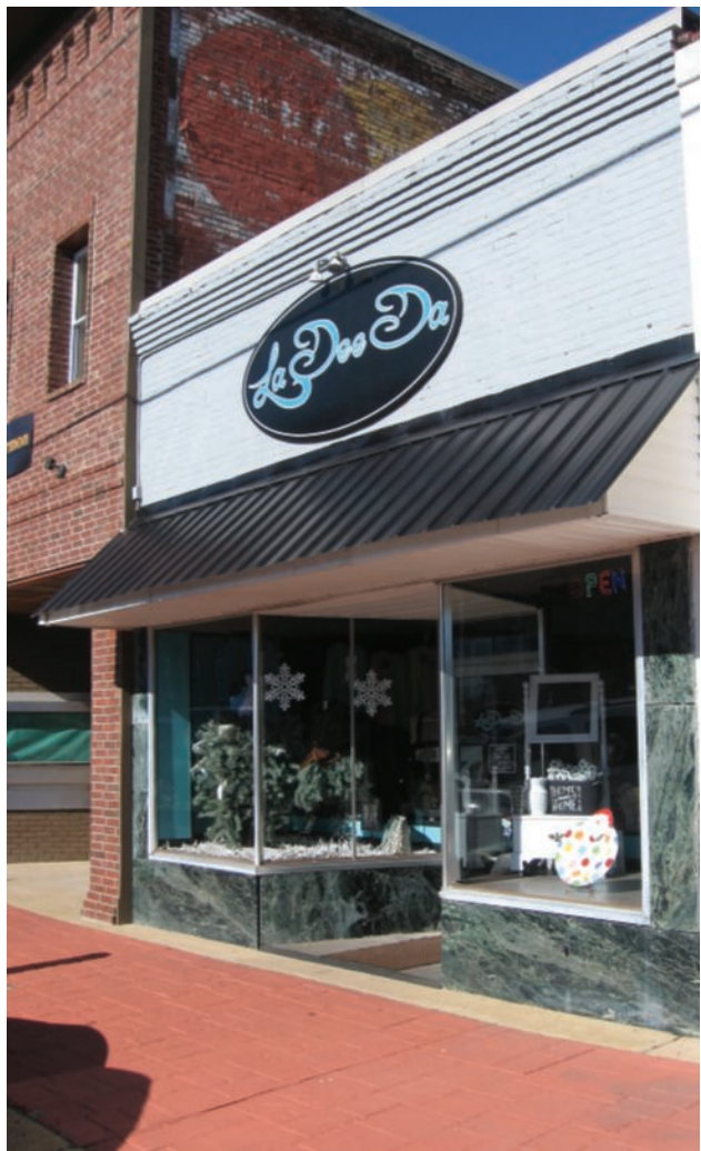
Figure 9: This midcentury storefront of marble panels is significant to the design of this ca. 1900 building in Savannah, Tennessee. The metal awning is a recent addition.
