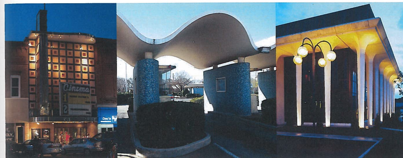
Figure 7: Left, a Taylorville, Illinois cinema was refaced in the mid-century with polychromed porcelain enamel panels and a swooping stainless steel and aluminum canopy, roof and dramatic pylon, photo: IHPA archives. Middle, the elegant Oklahoma City, Oklahoma, Central Motor Bank drive-up, built in 1959, combines a thin-shell concrete roof with bright blue mosaic tile encased piers, photo: Ann V. Swallow. Right, precast concrete columns surround a dark curtain wall on this Moline, Illinois, bank, designed by John Van Schellema of the Illinois Bank Building Corporation in the 1970s, photo: John Van Schellema.
